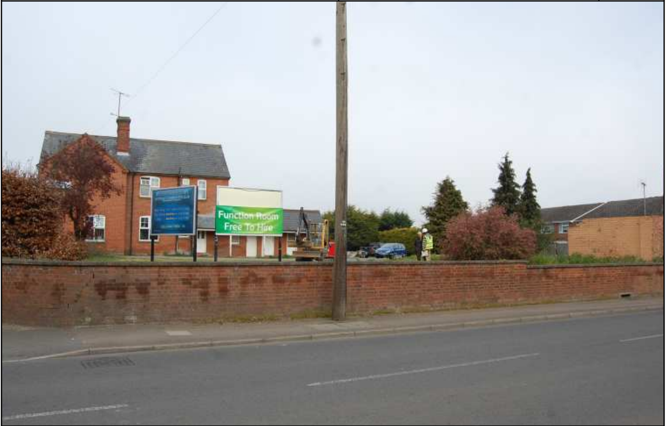
Plate 1: Site, looking north from Regent Street, showing raised ground surface
