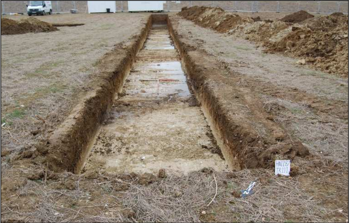
Plate 17: Trench 111, looking south east
