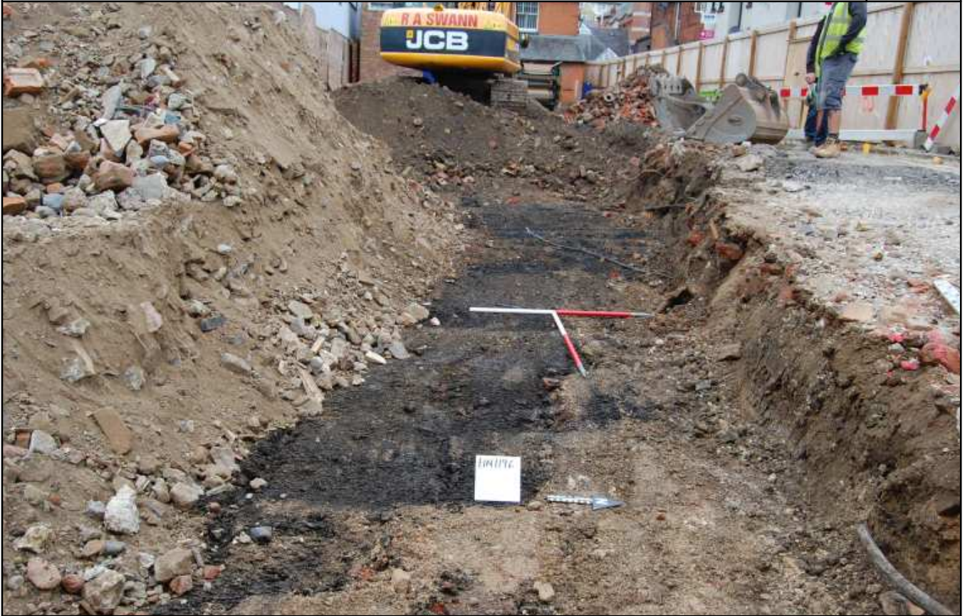
Plate 3: Ground reduction, showing alluvium in base of trench, looking west
