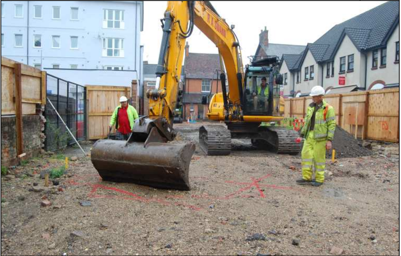
Plate 1: View of site prior to ground reduction, looking west
