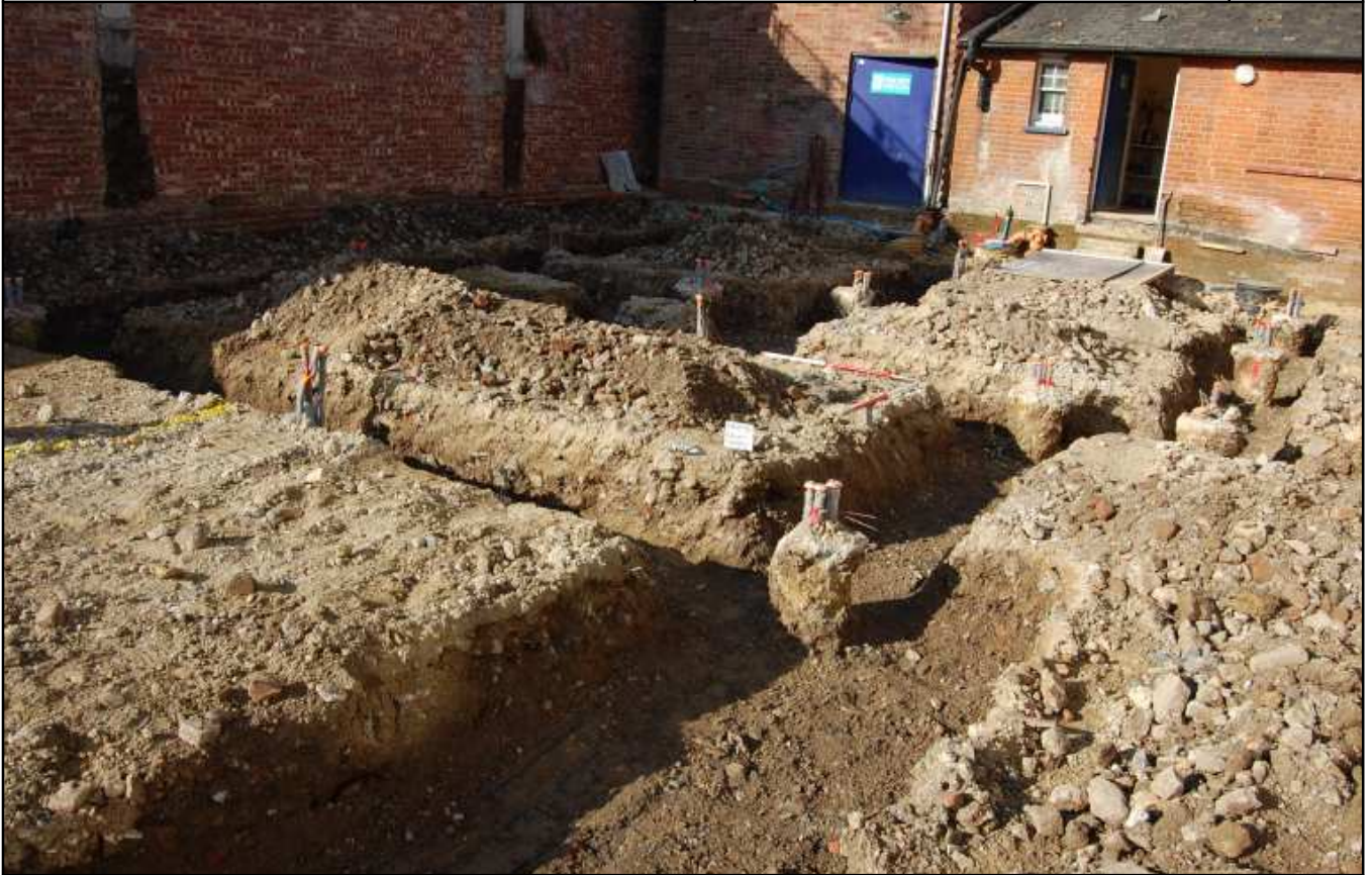
Plate 9: Ground beam trenches, west end of site, looking west
