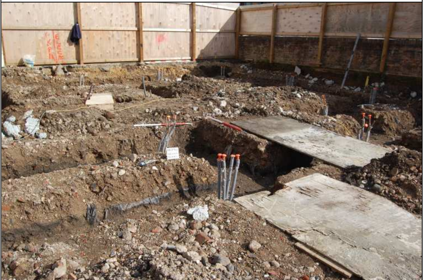
Plate 10: Ground beam trenches, east end of site, looking south-east
