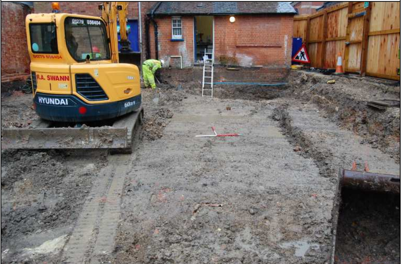
Plate 4: Reduced ground, showing depth of excavation and alluvium spread, looking west
