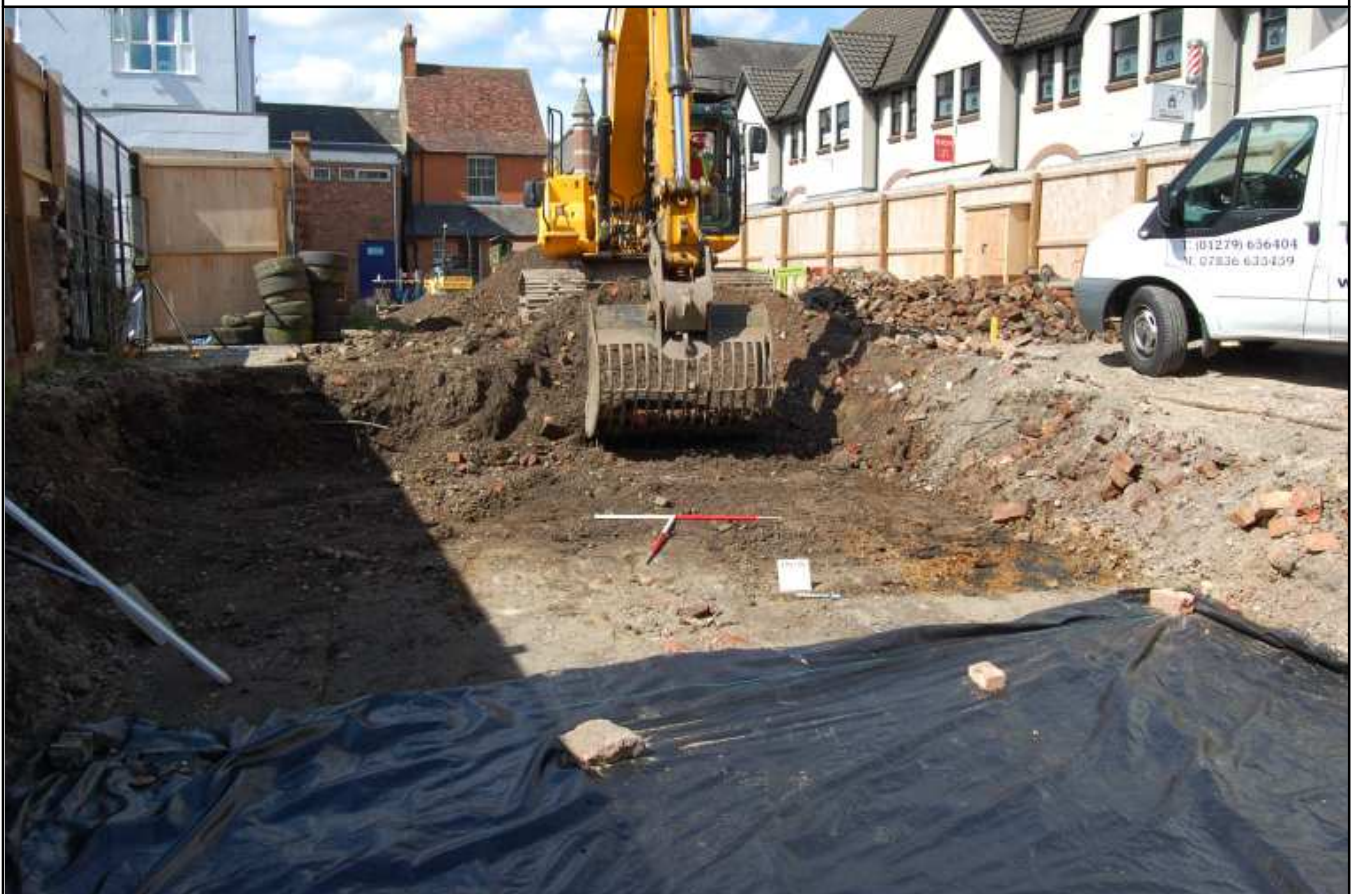
Plate 2: View of ground reduction, looking west
