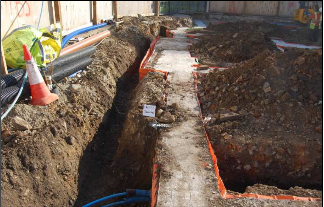
Plate 11: Drainage run, looking east
