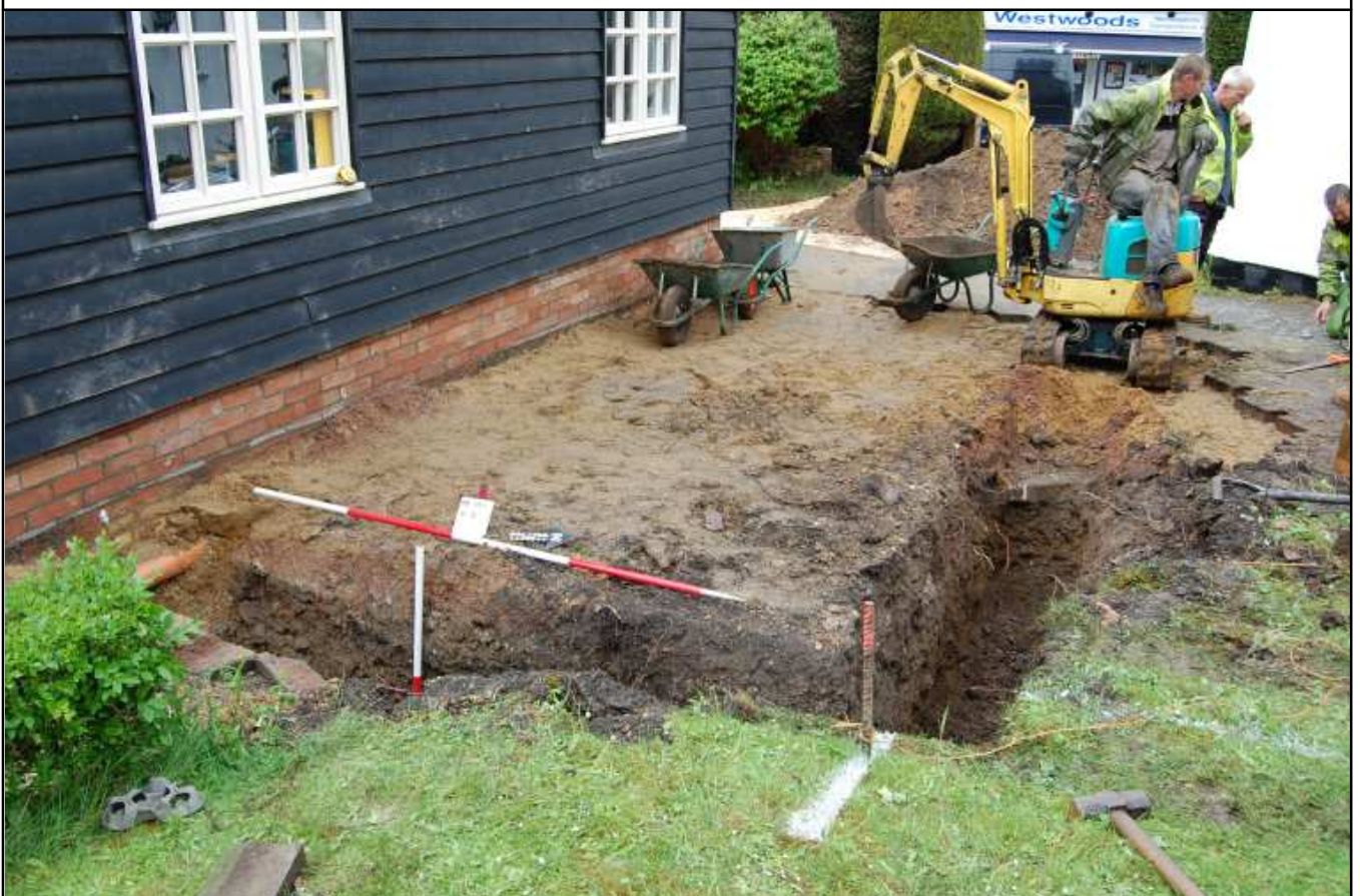
Plate 2: View of trench, looking north west
