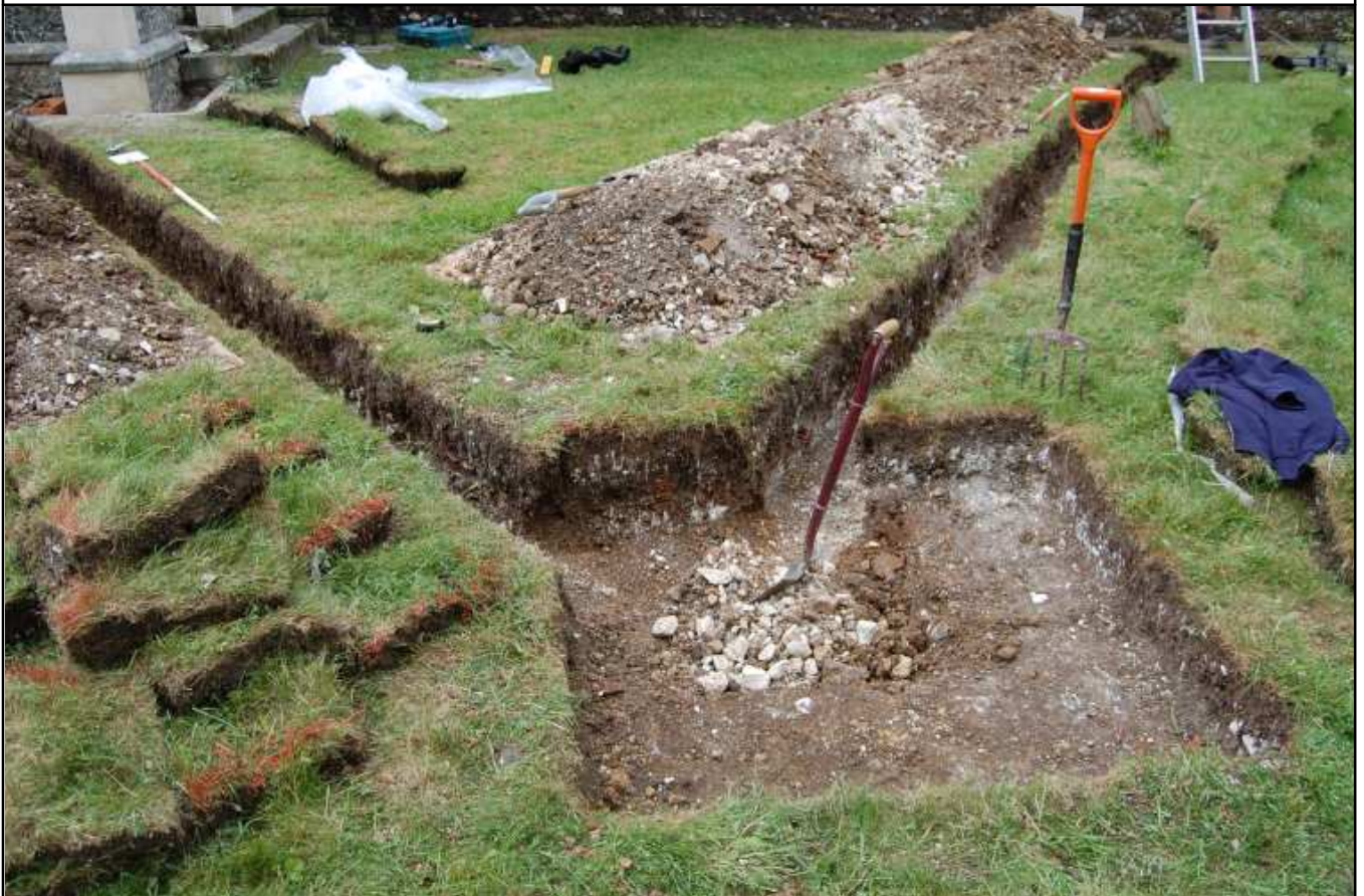
Plate 2 Drain run trenches to soakaway looking S
