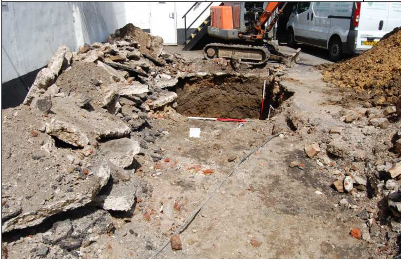
Plate 1: Evaluation trench, looking north-west
