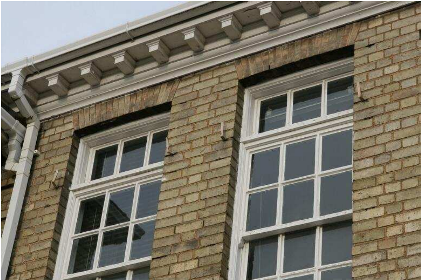
Plate 06 - S elevation, detail of metal brackets flanking the windows
