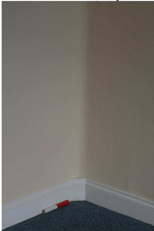
Plate 16 - Room F2, original skirting in NE corner
