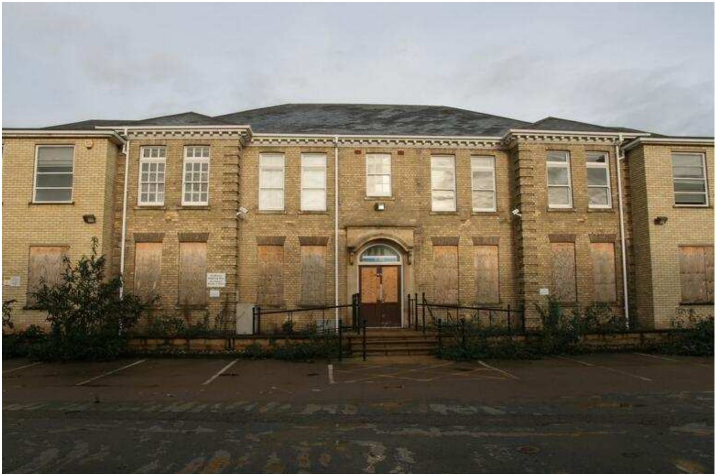
Plate 04 - S elevation, Central bays
