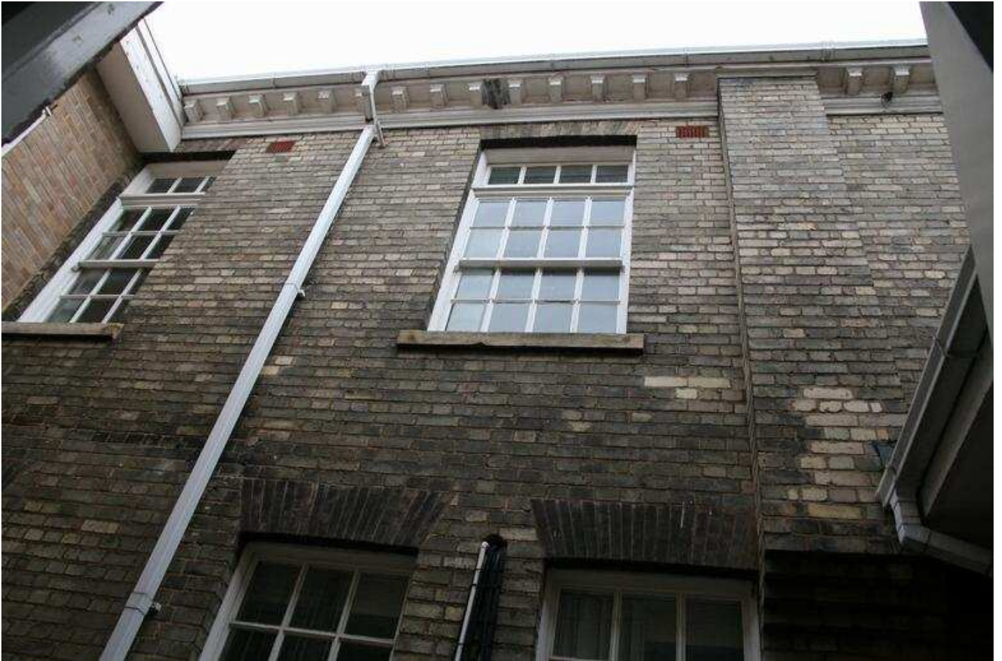
Plate 11 - Surviving part of original north elevation
