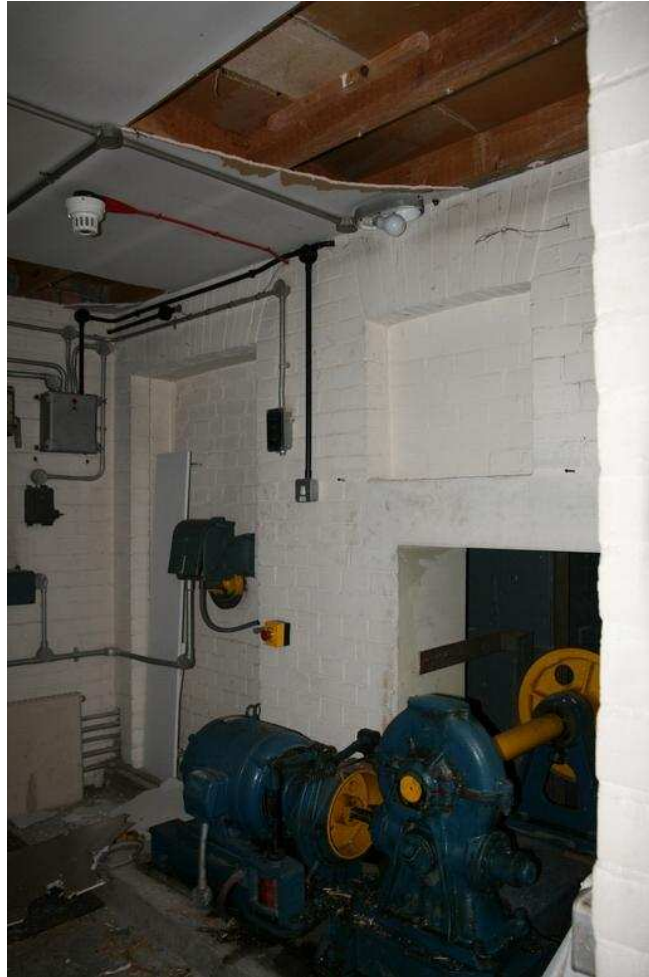
Plate 13 - Original doorways in east elevation of Plant Room
