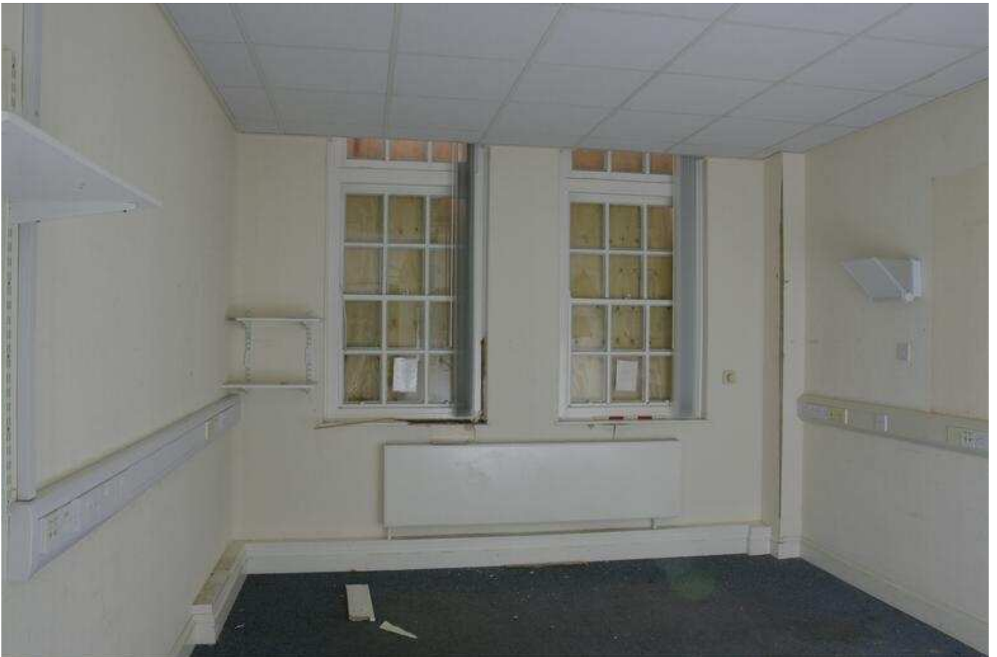
Plate 12 - Room G2, looking S
