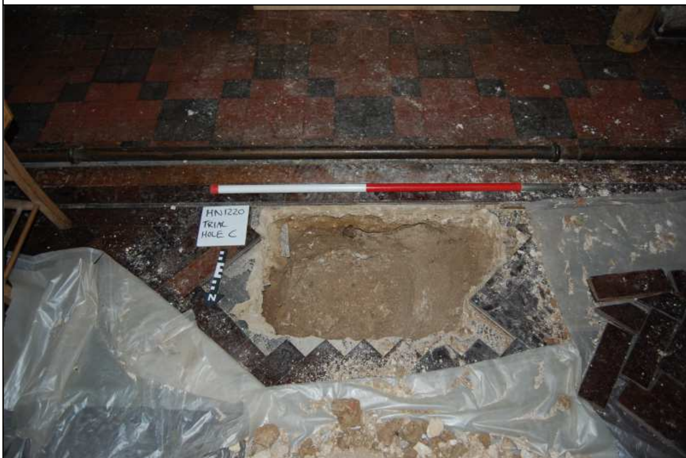
Plate 4 Trial Hole C Looking South
