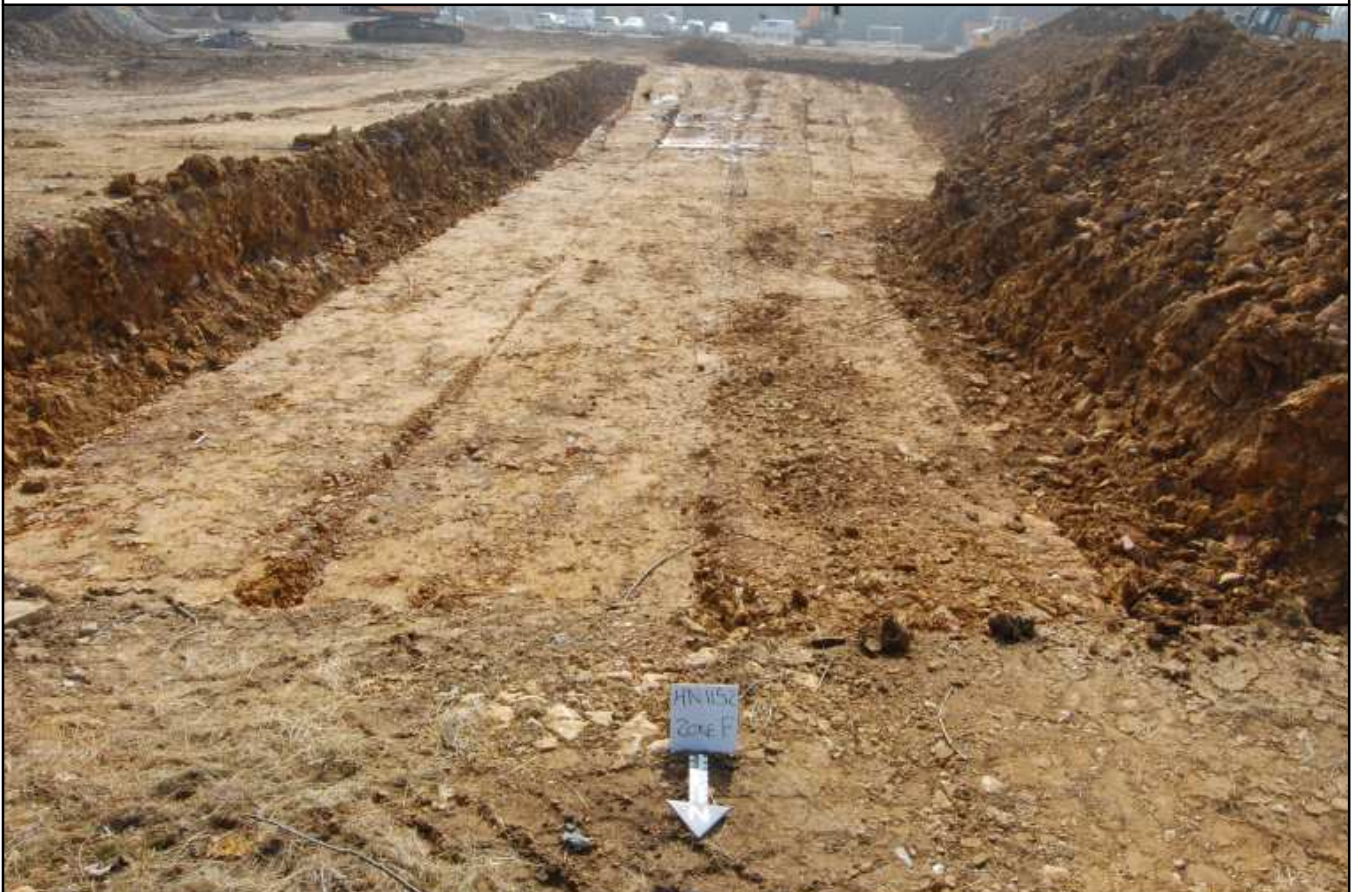
Plate F8: Zone F, remediation works, looking south
