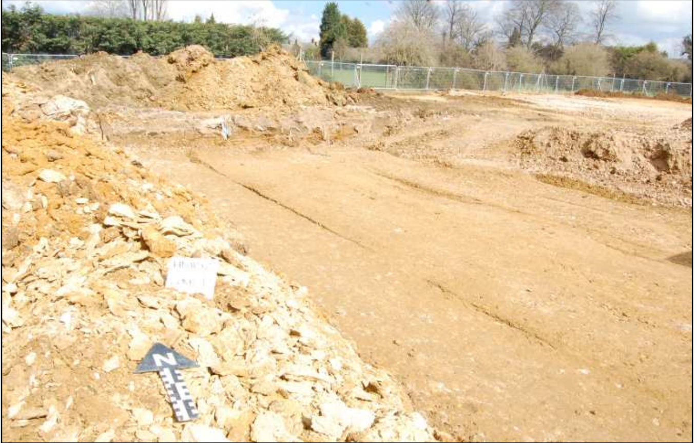
Plate F9: Zone F, remediation works, looking north
