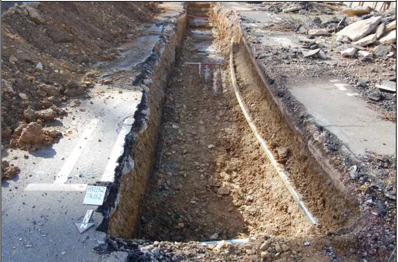
Plate B2: Trench B2, looking south
