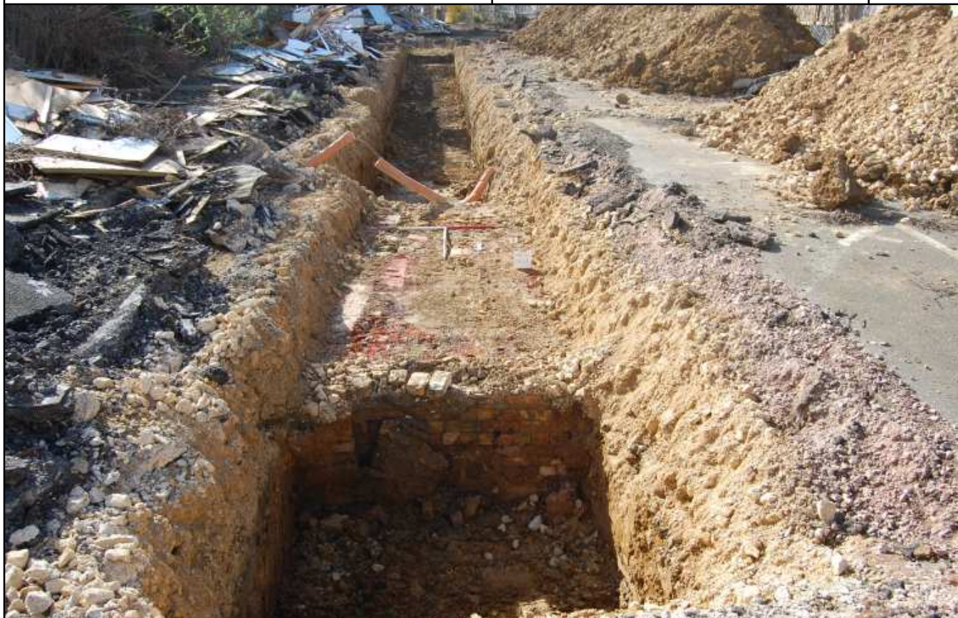
Plate B3: Trench B3, showing wall foundations, looking south
