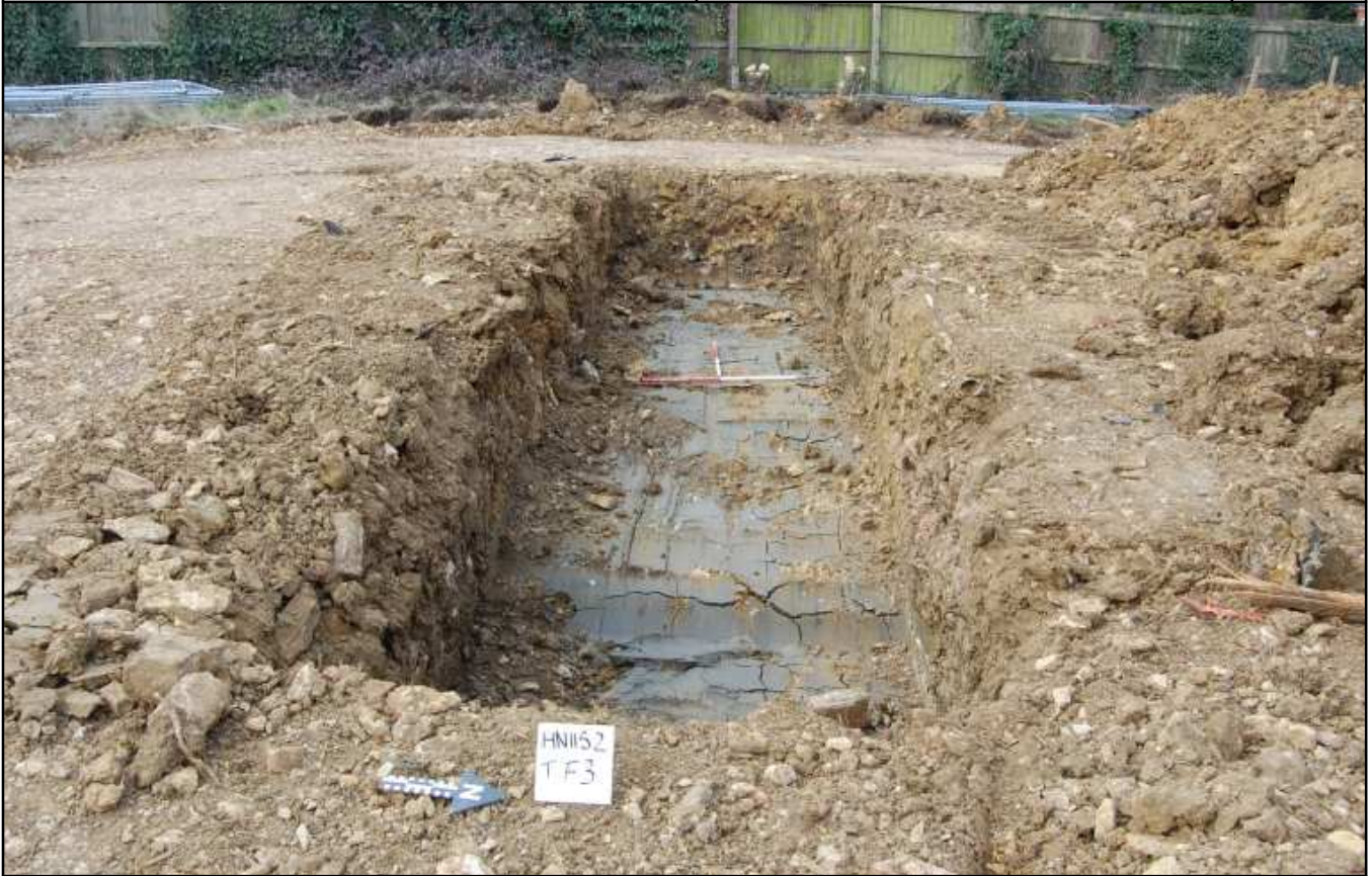
Plate F3: Trench F3, looking west
