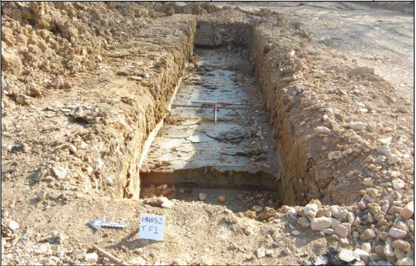
Plate F1: Trench F1, looking east
