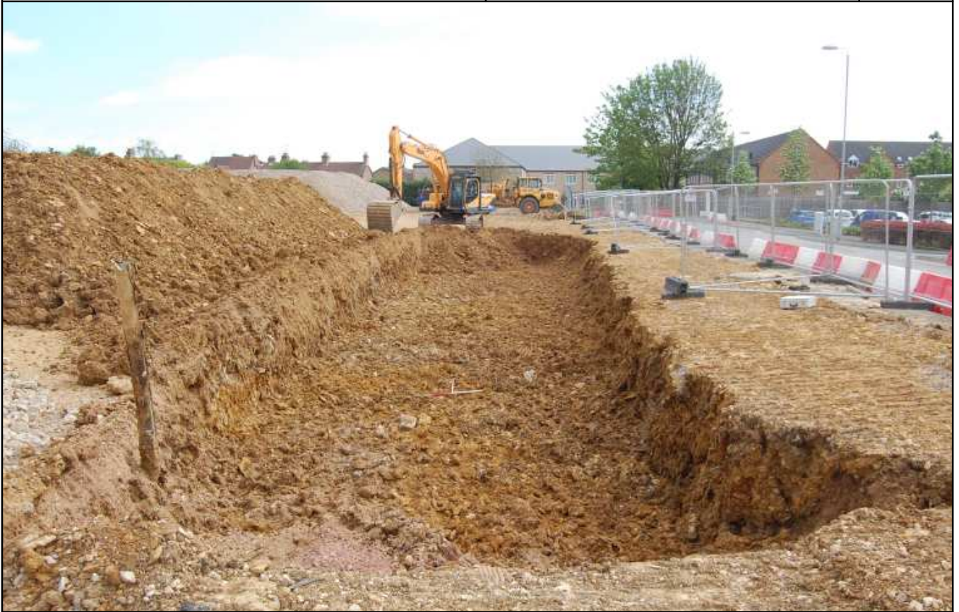
Plate E23: Zone E, remediation works, looking east
