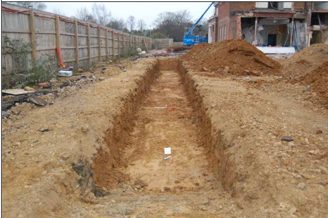
Plate B10: Trench B5, looking south east
