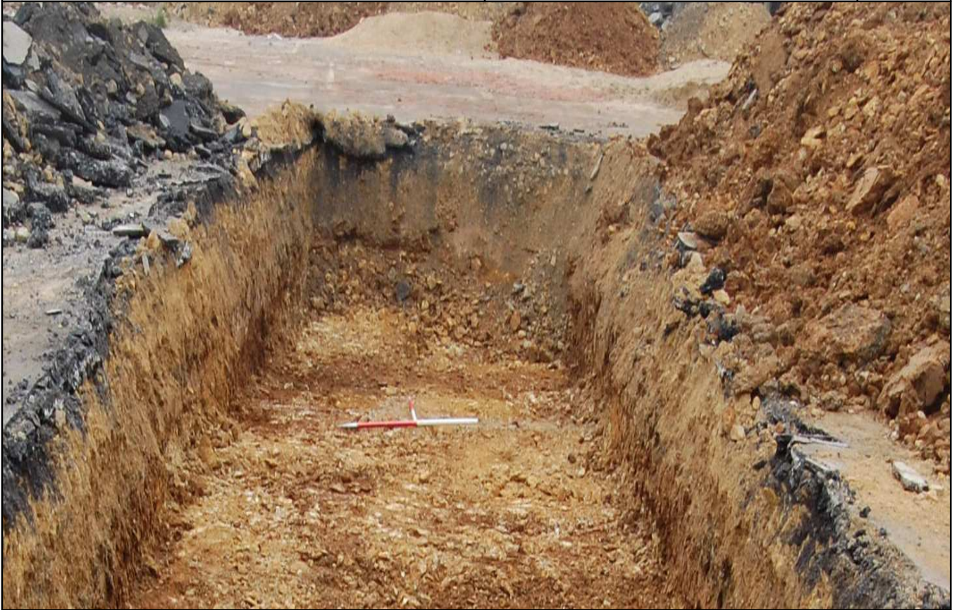
Plate E7: Linear ditch [201], looking west. (Pre-excitation)
