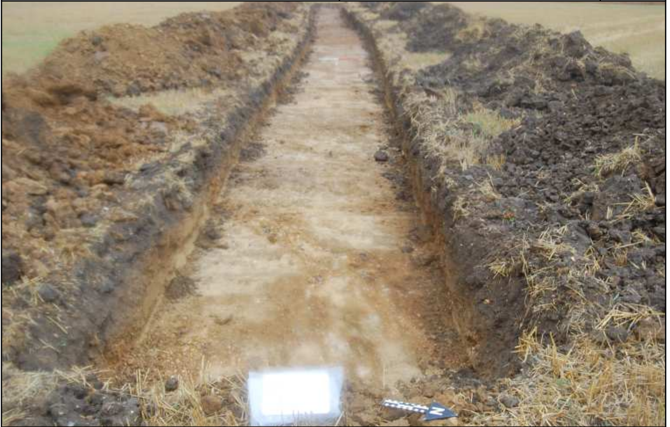
Plate 5: Trench 4, looking south-west
