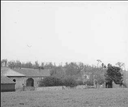
Frame 7: General view looking SE
