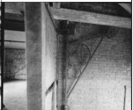
Frame 12: Western hoist
