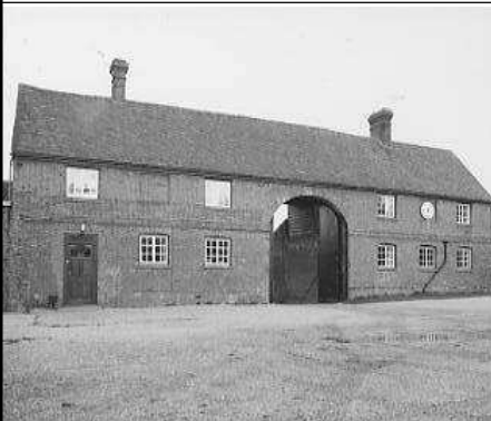
Frame 10: Former stable block, western elevation
