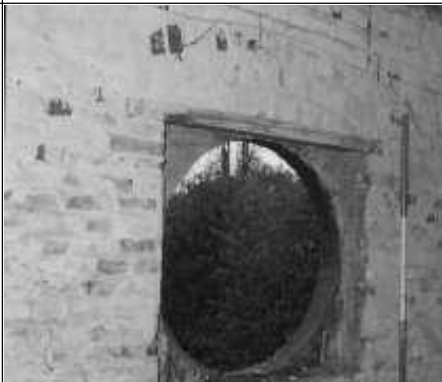
Frame 5: First floor, W half, S elevation circular window opening
