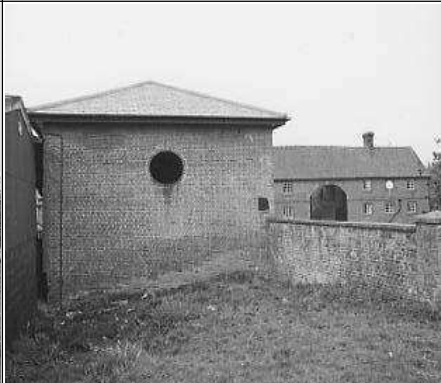
Frame 5: Western exterior elevation and former stable block
