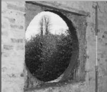
Frame 4: First floor, W half, S elevation circular window opening
