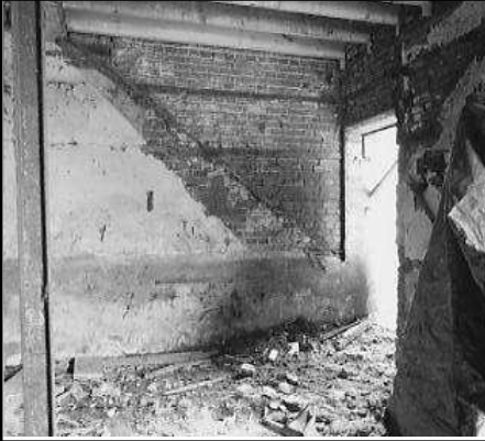
Frame 1: Ground floor, eastern half Doorway & outline of staircase
