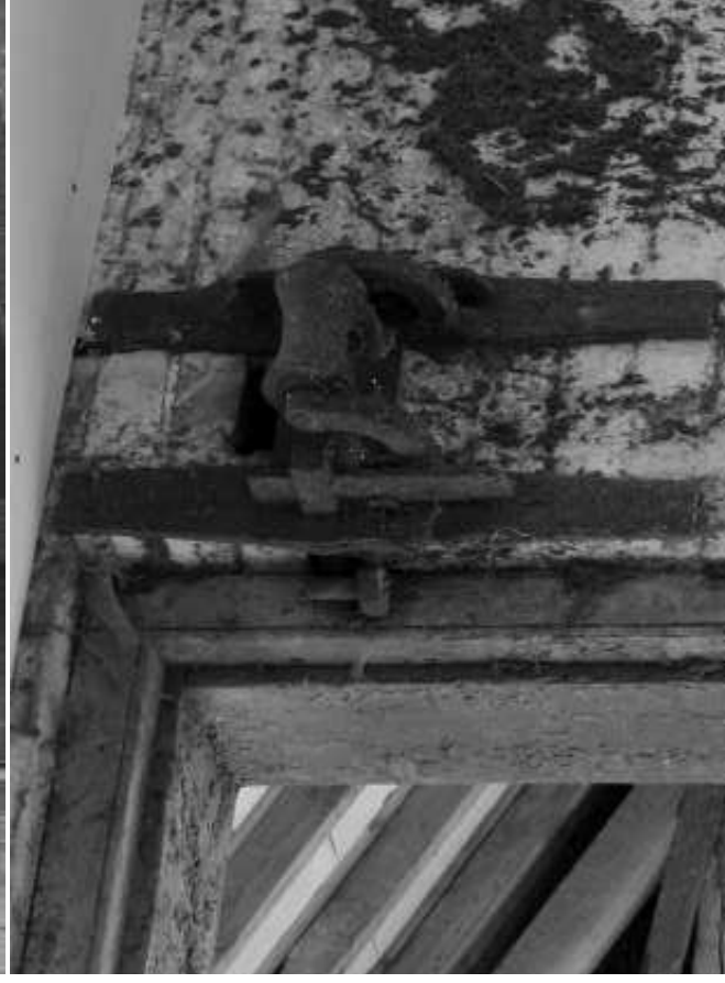
Plate 10: Hoist pulley details (exterior west/interior east)
