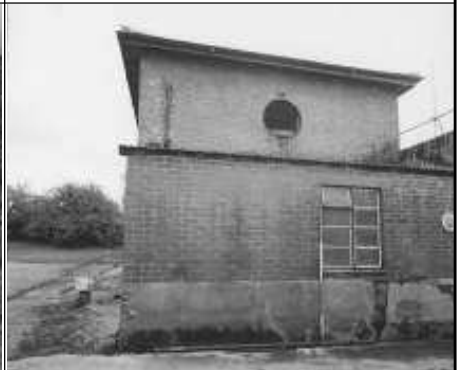
Frame 9: Eastern exterior elevation
