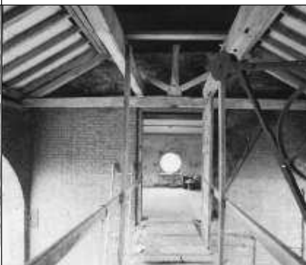
Frame 11: Rooftruss over bridge
