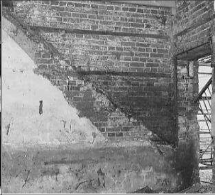
Frame 2: Ground floor, eastern half Doorway & outline of staircase
