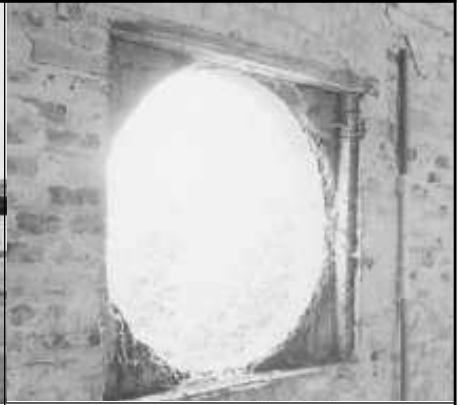
Frame 3: First floor, W half, S elevation circular window opening
