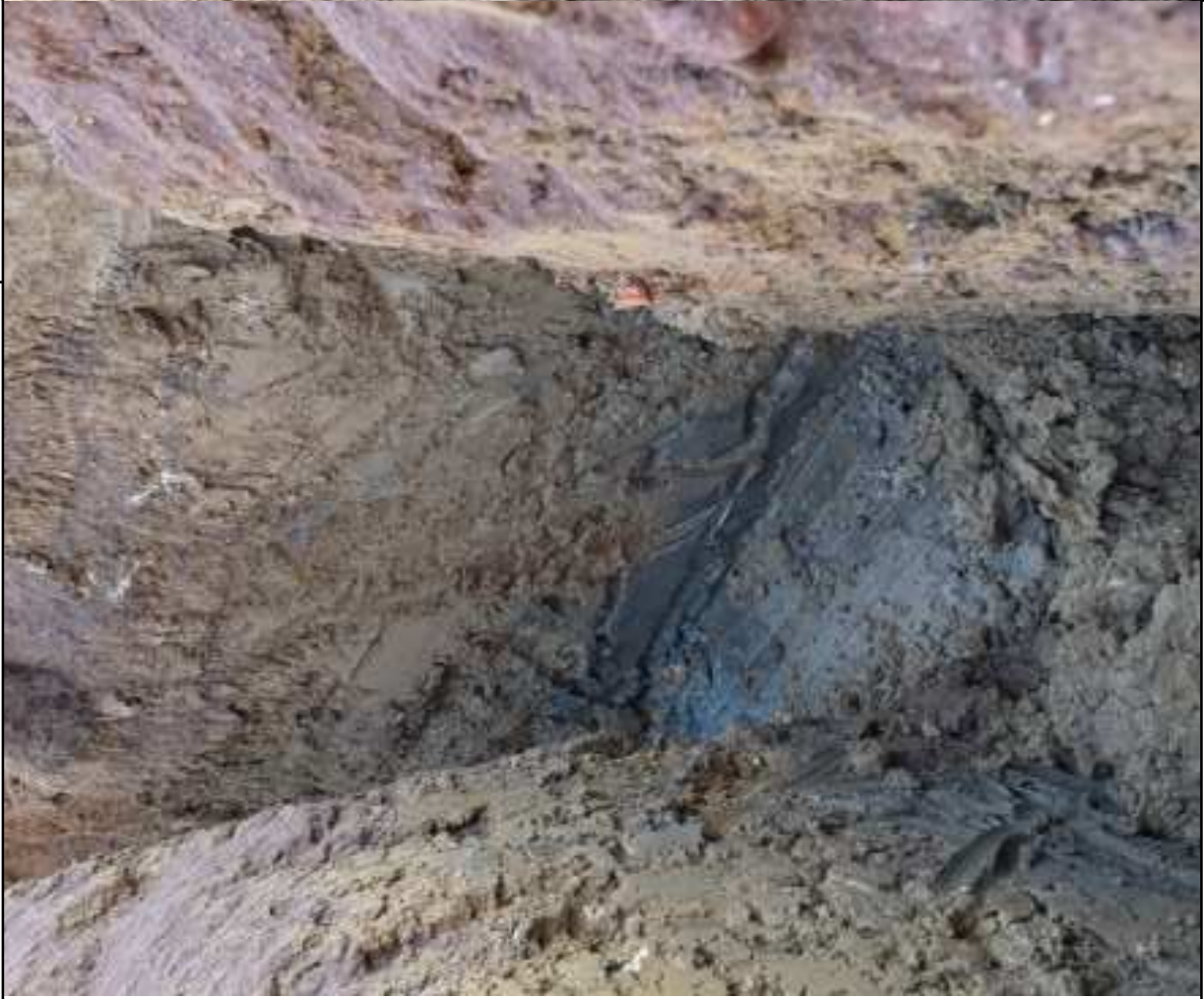
Plate 5: Foundation trench sections looking N
