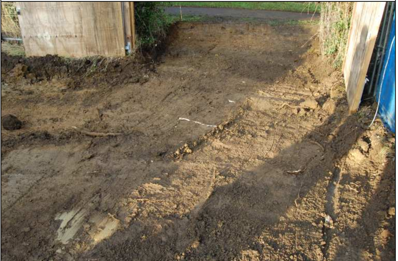
Plate 4: Reduced access road looking north
