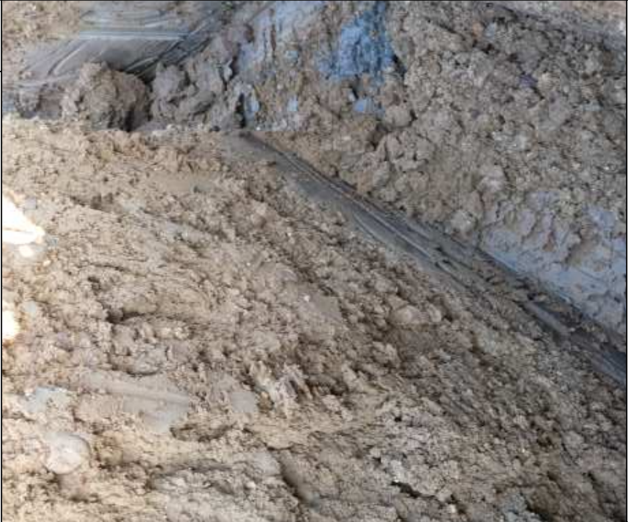
Plate 6: Foundation Trench sections looking south
