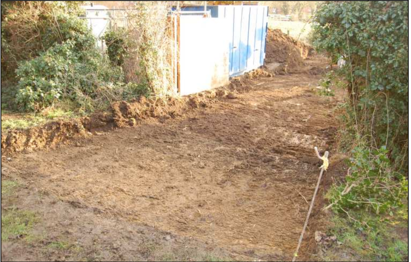
Plate 3: Reduced area of access road looking south
