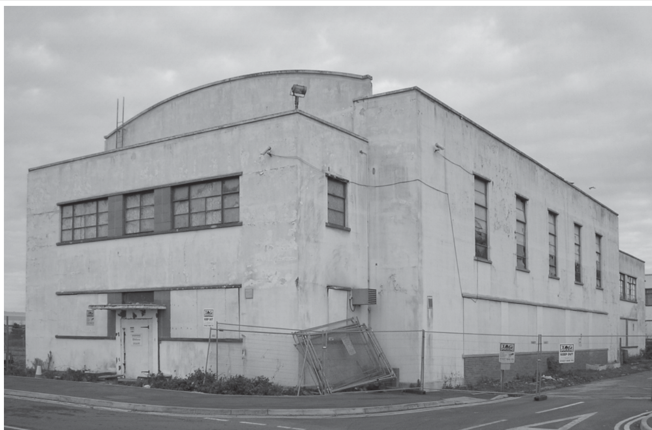
Plate 2: Canteen block, southern and eastern elevations
