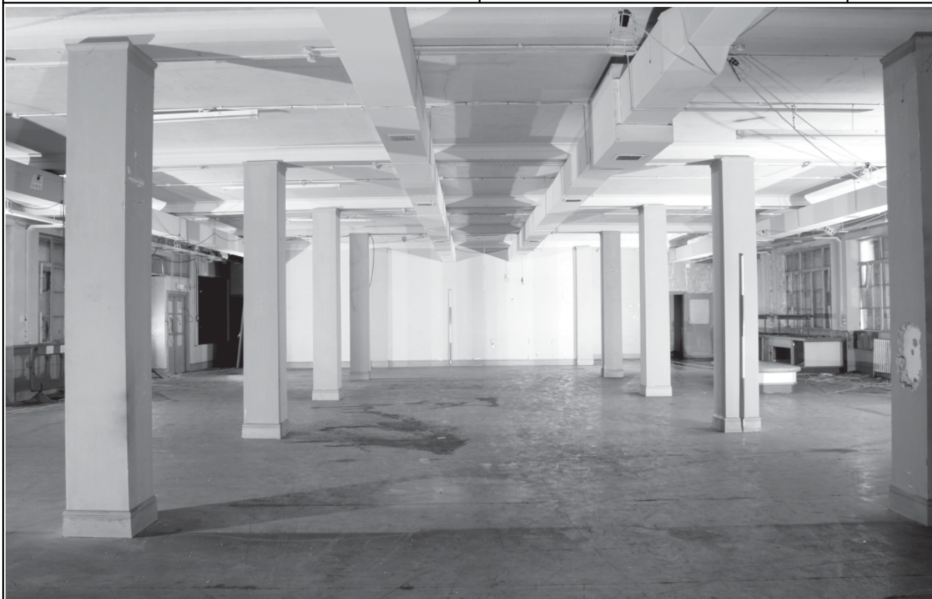
Plate 5: Canteen block, ground floor canteen, looking N
