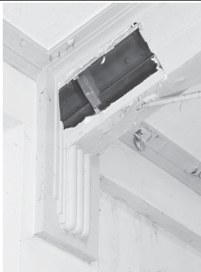
Plate 10: Canteen block, first floor hall, decorative corbel and boxed joist
