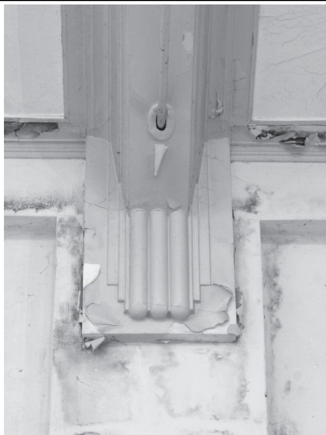
Plate 10: Canteen block, first floor hall, decorative corbel and boxed joist
