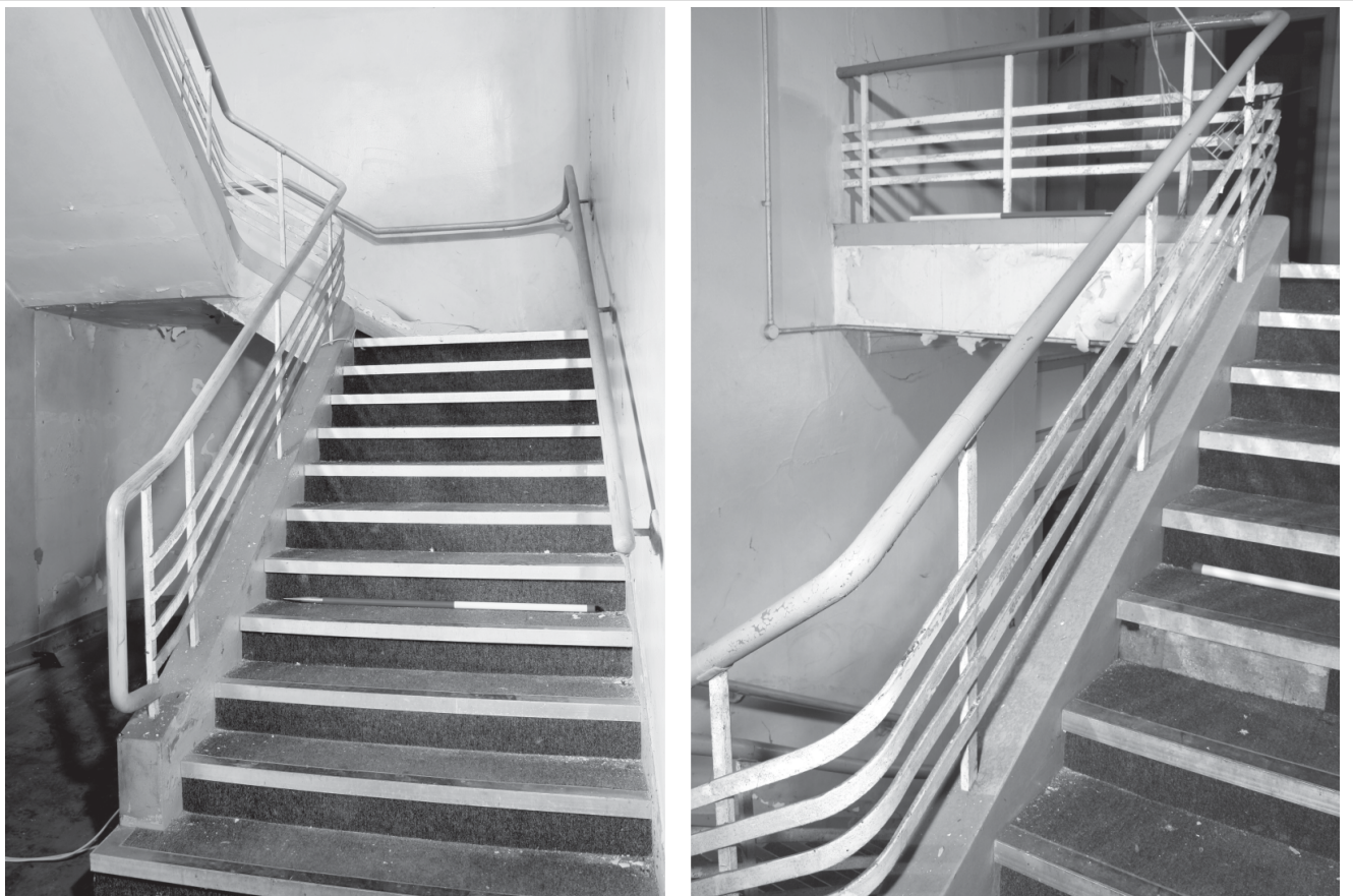
Plate 4: Canteen block, southern staircase
