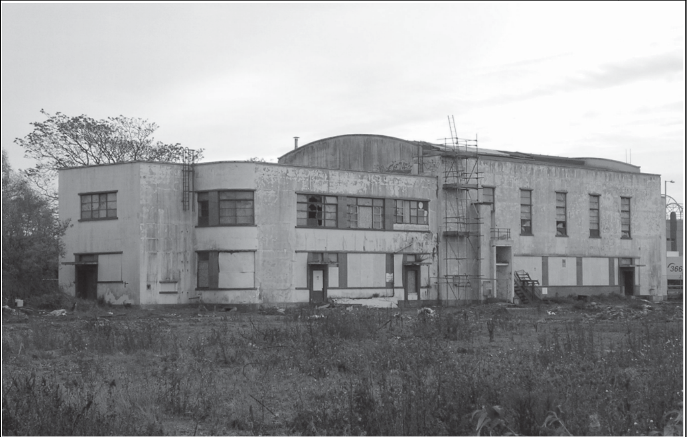
Plate 3: Canteen Block, northern and western elevations
