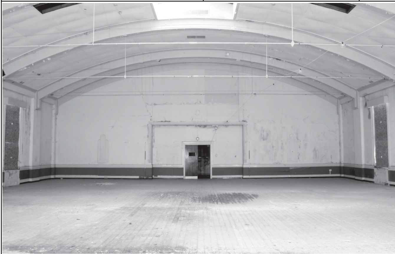
Plate 9: Canteen Block, first floor hall, looking S
