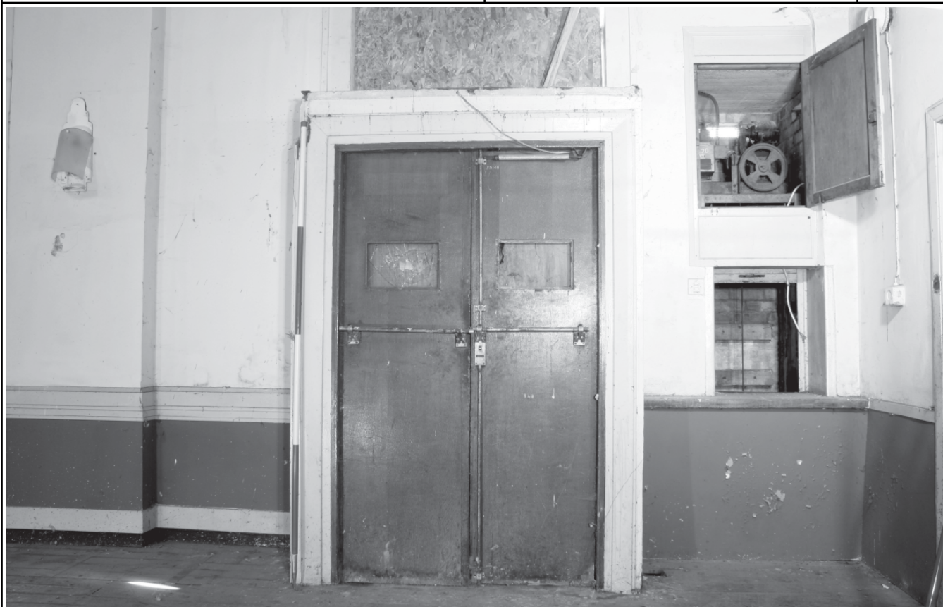
Plate 11: Canteen block, first floor hall, emergency exit and dumb waiter
