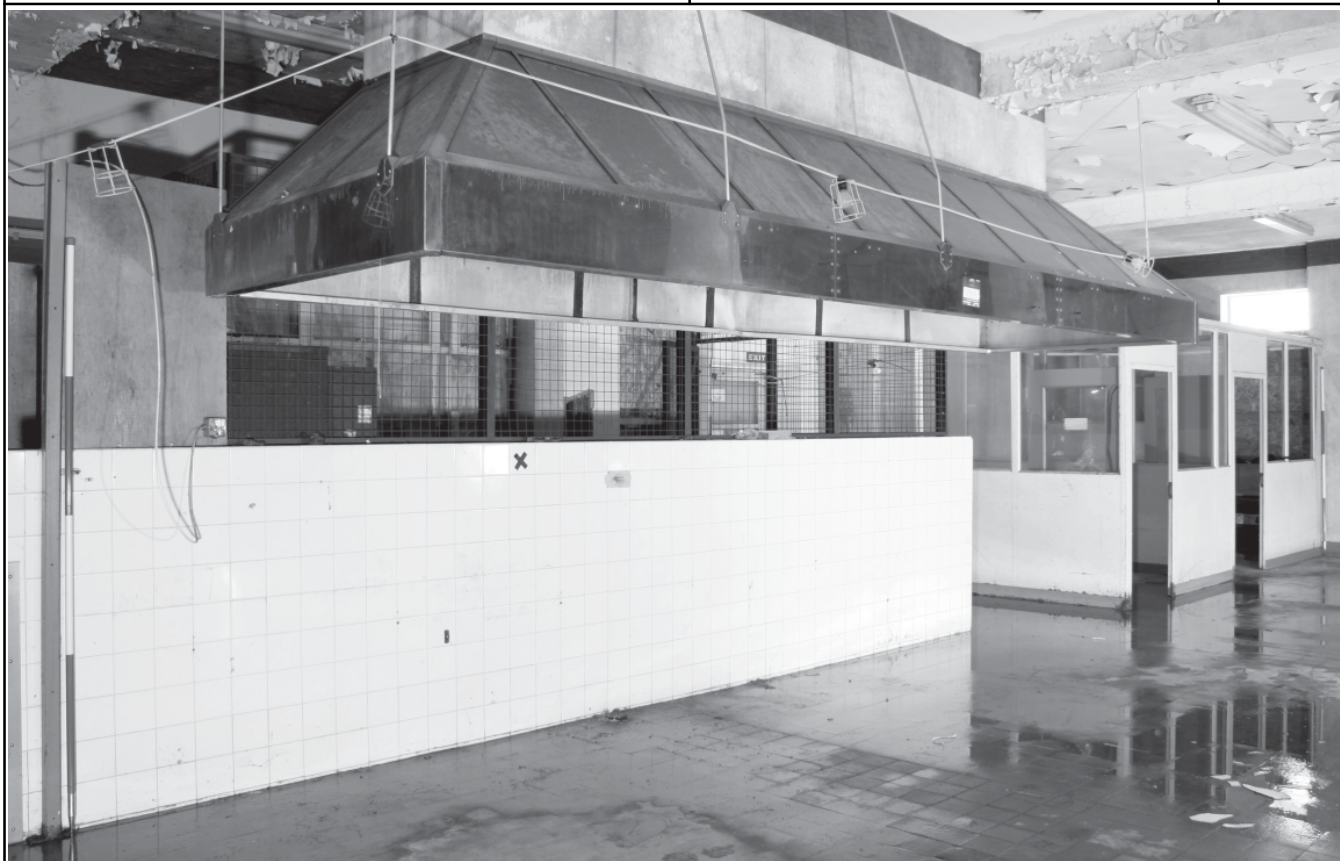
Plate 7: Canteen block, kitchen, looking NW
