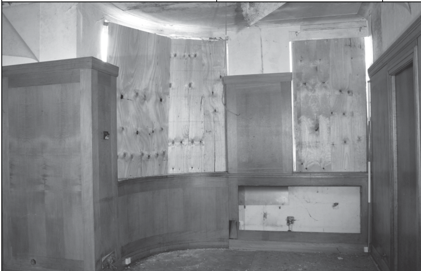
Plate 27: Administration block, Room 49, E elevation
