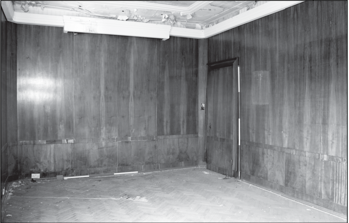
Plate 25: Administration block, boardroom, looking S
