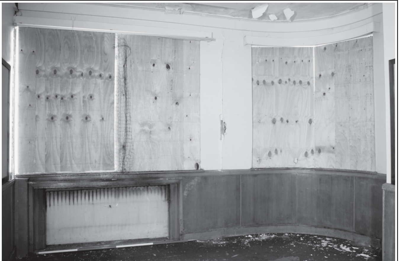
Plate 32: Administration block, Room 51, E elevation
