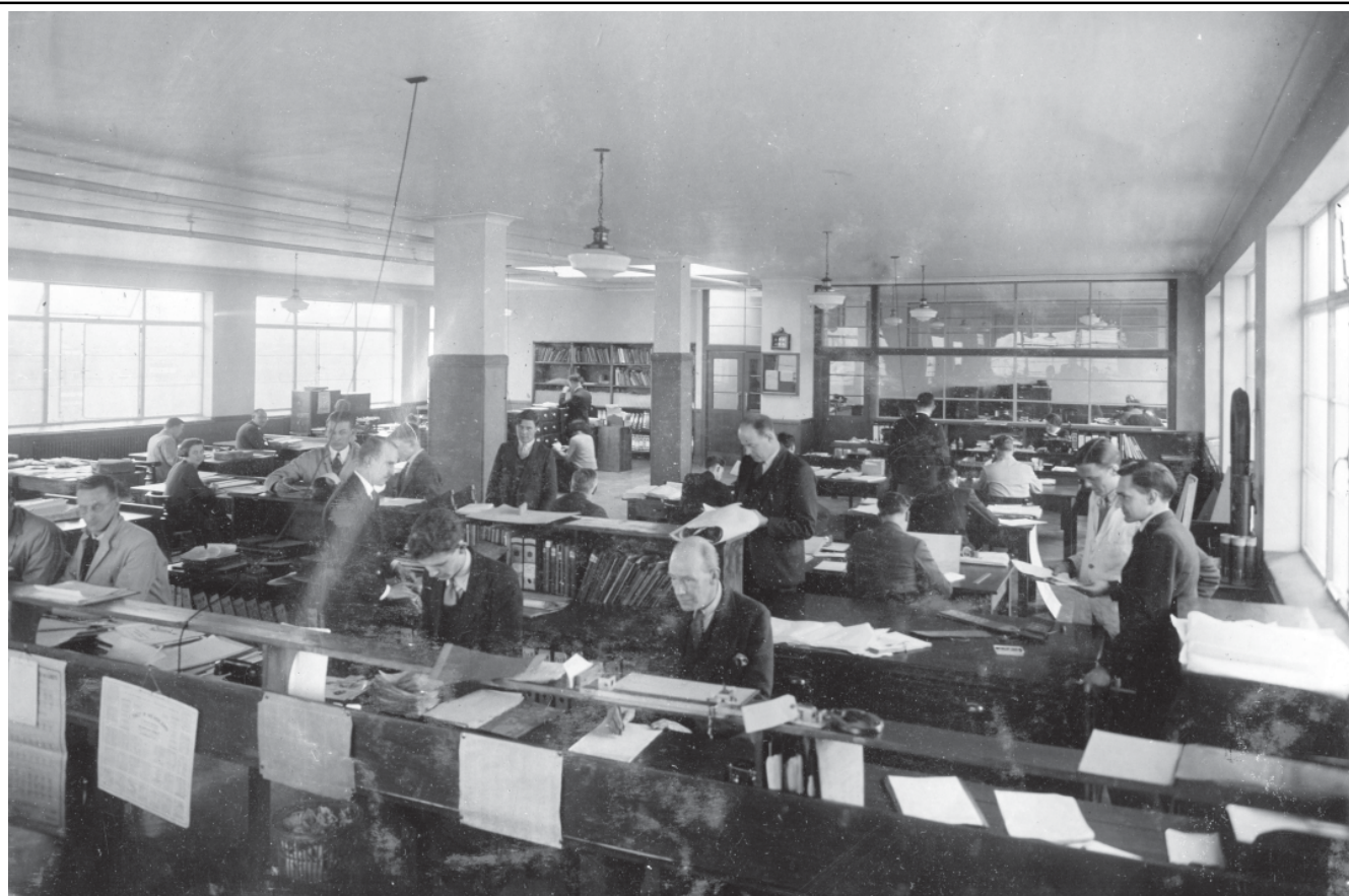
Plate 36: Administration block, engineering office, 1930s (London & Provincial 7 from BAE SYSTEMS archive)
