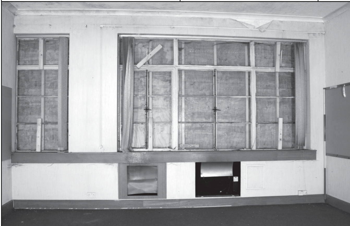
Plate 17: Administration block, typical office arrangement, southern corridor, western side
