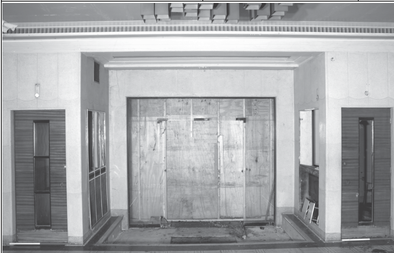
Plate 15: Administration block, lobby and lodges, looking E
