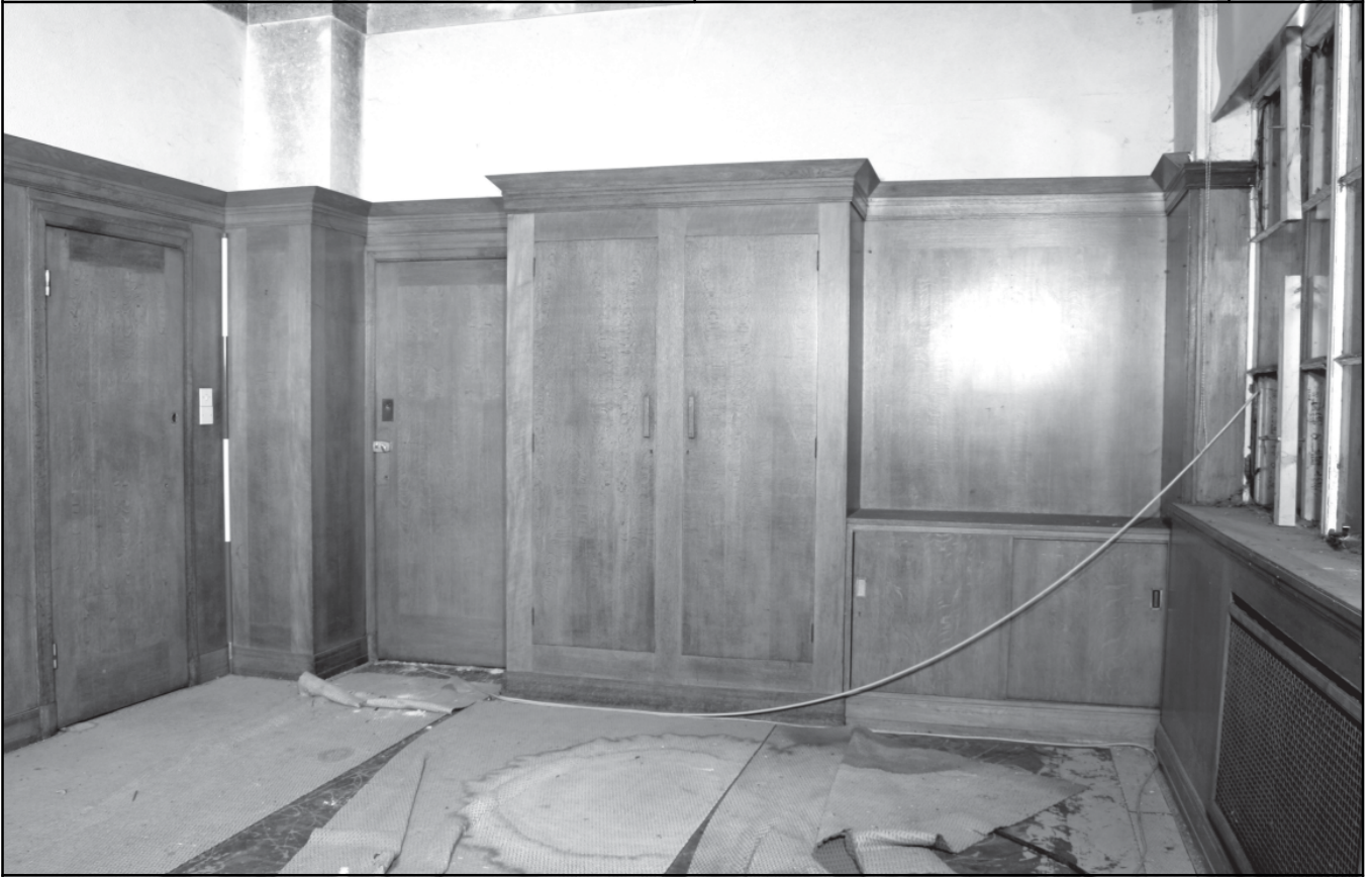
Plate 19: Administration block, Room 38, E elevation
