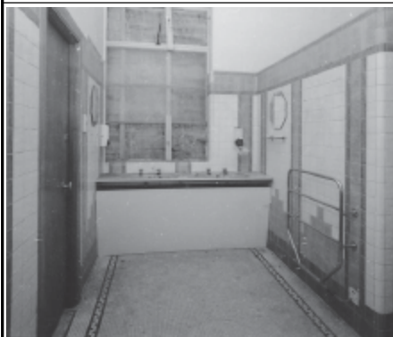
Frame 4: Admin Block, G floor WC adj. Room 32, facing W
