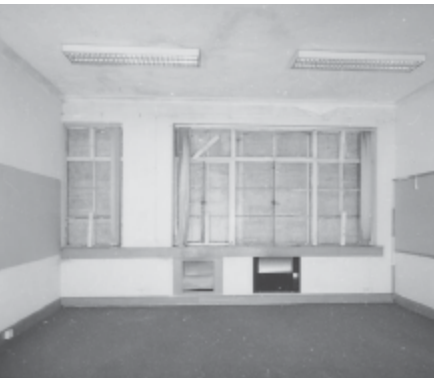
Frame 4: Admin Block, G floor Room 35, facing W
