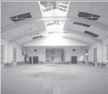
Frame 4: Canteen, 1st floor Ballroom, facing N
