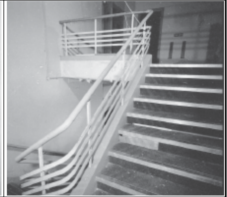
Frame 3: Canteen S staircase, upper level, facing E
