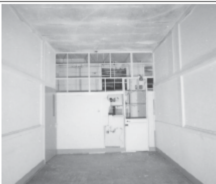
Frame 8: Admin Block, 1st floor Room 47, facing W
