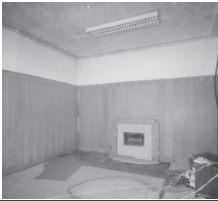
Frame 1: Admin Block, G floor Room 1, facing NE
