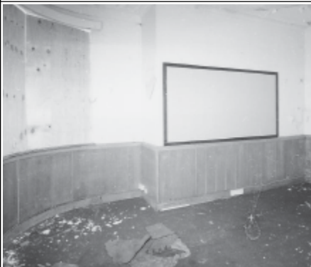
Frame 10: Admin Block, 1st floor Room 51, facing SW
