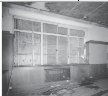
Frame 3: Admin Block, G floor Room 38, facing S
