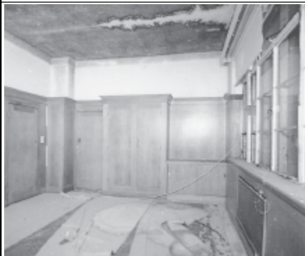
Frame 7: Admin Block, G floor Room 38, facing E
