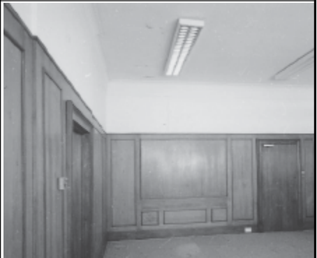
Frame 9: Admin Block, G floor Room 5, facing W
