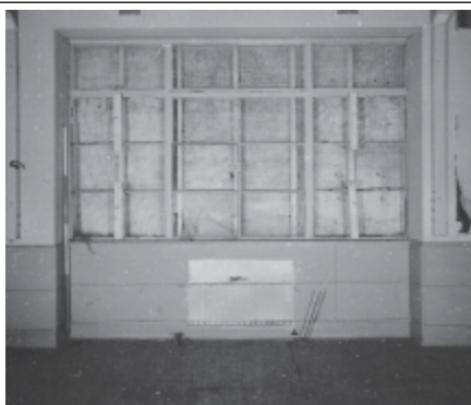
Frame 11: Canteen, G floor Window detail, facing W
