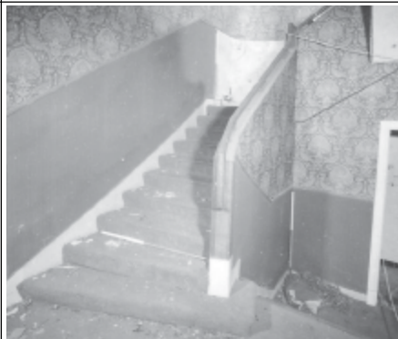
Frame 11: Canteen, G floor N staircase, facing W
