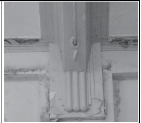
Frame 3: Canteen Ballroom, reeded corbel
