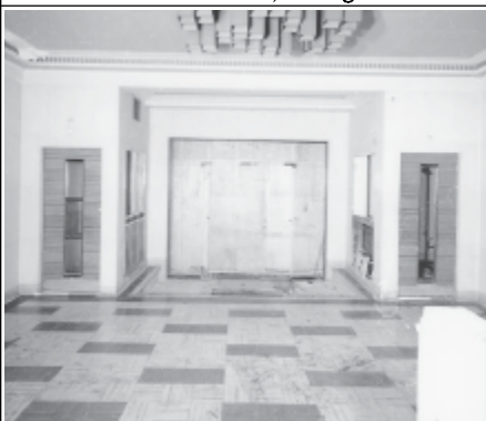
Frame 10: Admin Block, G floor Entrance Hall, facing E
