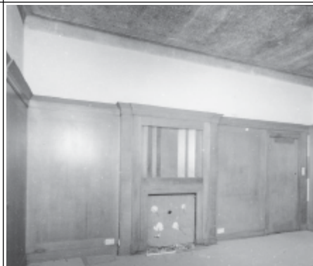
Frame 6: Admin Block, G floor Room 38, facing N
