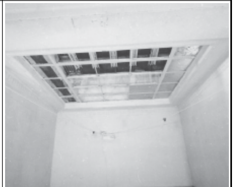
Frame 9: Admin Block, 1st floor Skylight above stairwell, facing W
