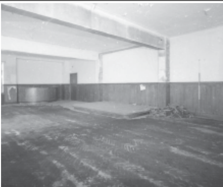
Frame 7: Canteen, 1st floor NW managers' dining room, facing NE
