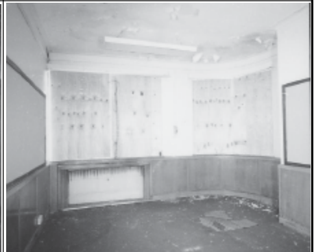
Frame 9: Admin Block, 1st floor Room 51, facing SE
