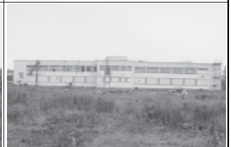
Frame 12: Admin, W exterior elevation
