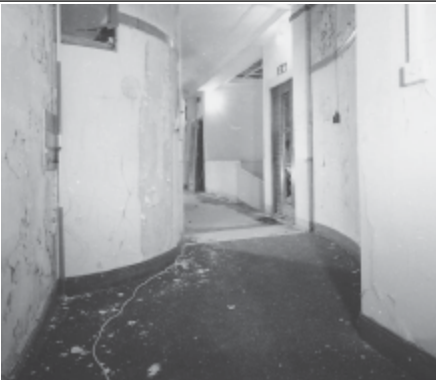
Frame 4: Admin Block, 1st floor Passage and landing, facing S
