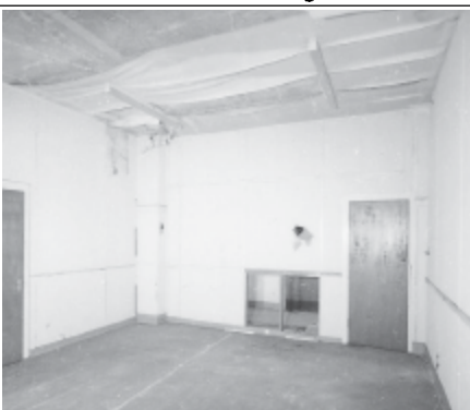
Frame 11: Admin Block, 1st floor Room 75, facing NE
