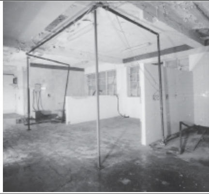
Frame 2: Canteen, G floor Kitchen, E half, facing NE
