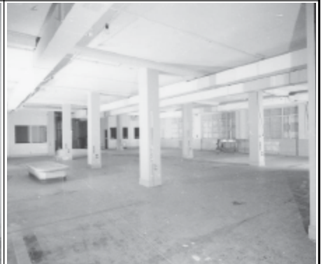
Frame 6: Canteen, G floor Dining room, facing SW
