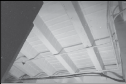
Frame 1: Admin Block, Cellar Coffered ceiling, detail, facing NE
