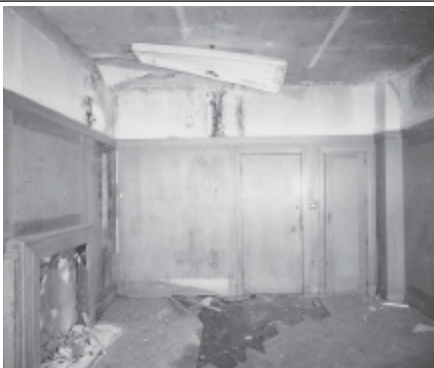
Frame 8: Admin Block, 1st floor Room 49, facing W
