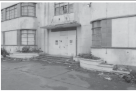
Frame 10: Admin, main entrance
