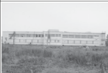
Frame 11: Admin, W exterior elevation
