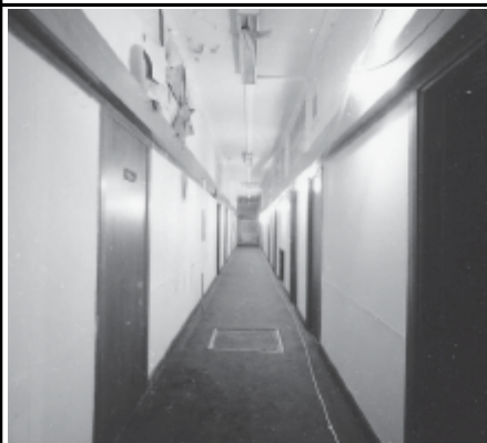
Frame 1: Admin Block, G floor S corridor, facing S
