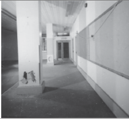
Frame 2: Admin Block, G floor Room 19, facing N
