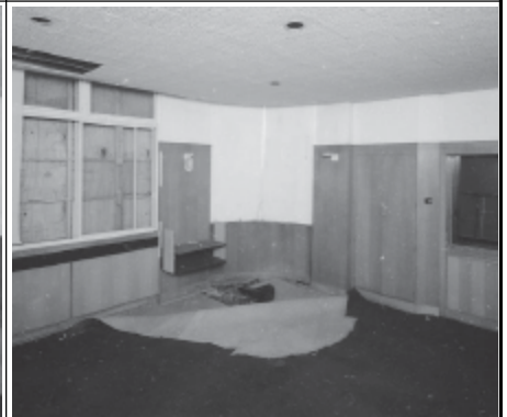
Frame 6: Admin Block, G floor Room 11, facing SE
