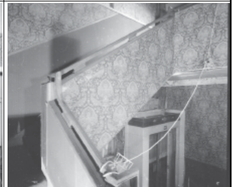
Frame 12: Canteen N staircase, upper level
