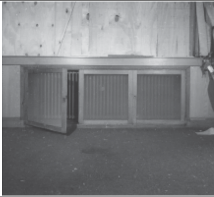
Frame 1: Admin Block, 1st floor Room 52, radiator grill, facing E
