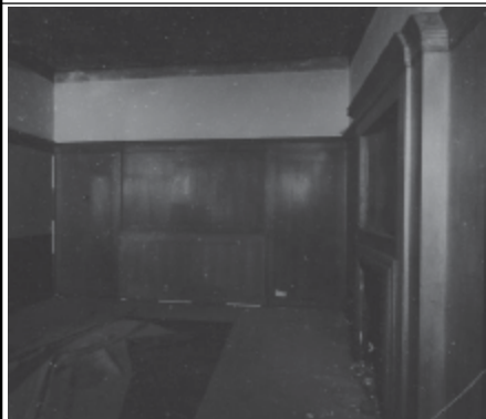
Frame 4: Admin Block, G floor Room 38, facing W
