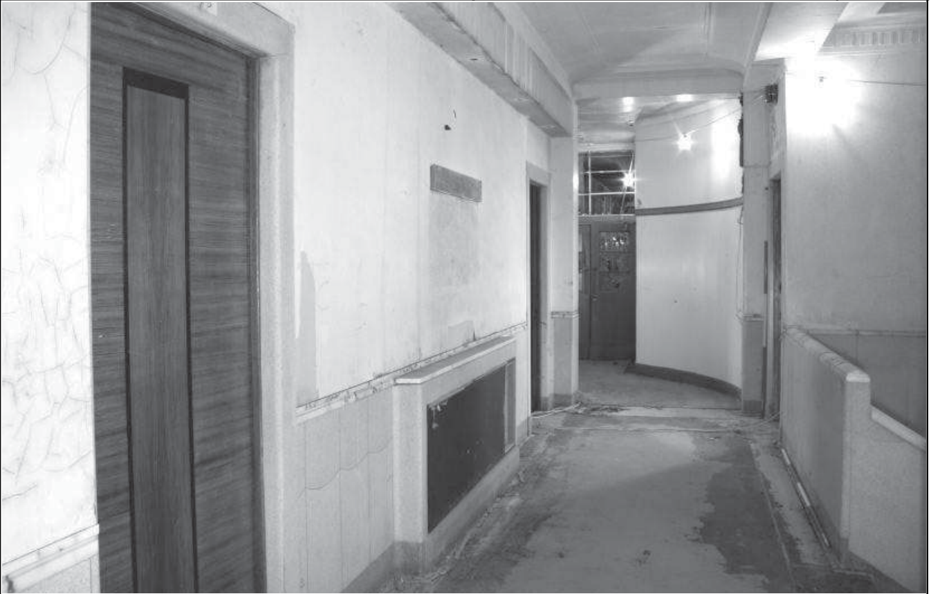
Plate 43: Admin block, first floor landing, looking S (Full report, para.3.16)
