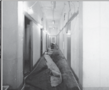
Frame 9: Admin Block, G floor N corridor, facing N
