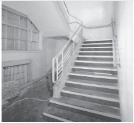
Frame 1: Canteen, G floor S staircase, facing W
