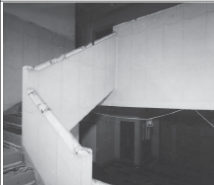
Frame 11: Admin Block Main staircase from 1st half-landing
