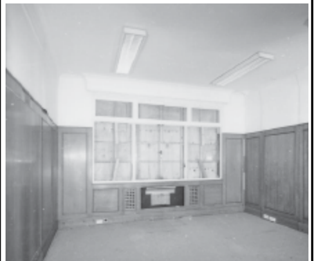
Frame 6: Admin Block, G floor Room 5, facing E
