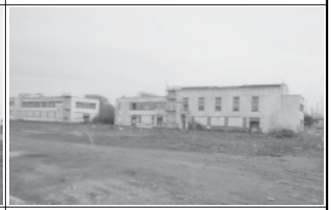
Frame 15: Western elevations, S end
