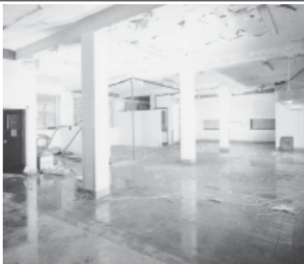
Frame 4: Canteen, G floor Kitchen, S end, facing SE
