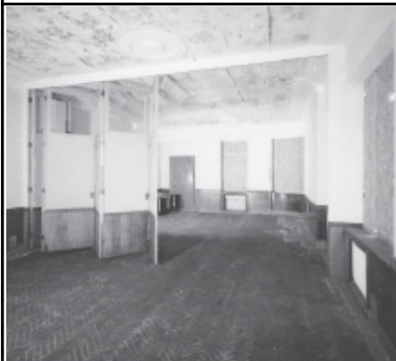
Frame 1: Canteen, 1st floor Managers' Common Room, facing NW
