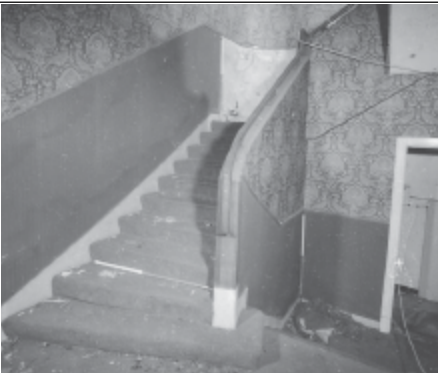
Frame 10: Canteen, G floor N staircase, facing W
