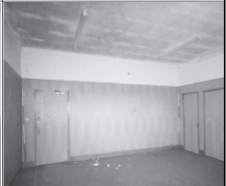
Frame 12: Admin Block, 1st floor Room 52, facing NE
