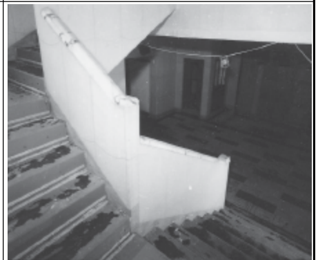
Frame 12: Admin Block Main staircase from 1st half-landing
