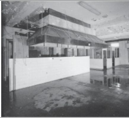
Frame 1: Canteen, G Floor Kitchen, W half, facing NW
