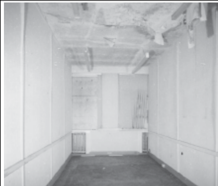
Frame 6: Admin Block, 1st floor Room 46, facing E
