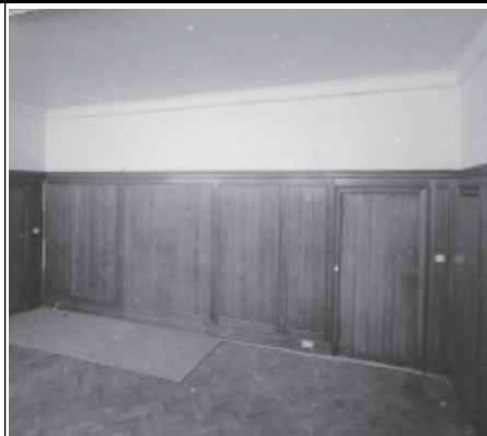
Frame 3: Admin Block, G floor Room 7, facing W
