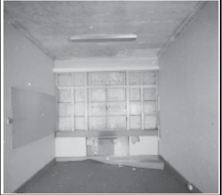
Frame 3: Admin Block, G floor Room 37, facing W
