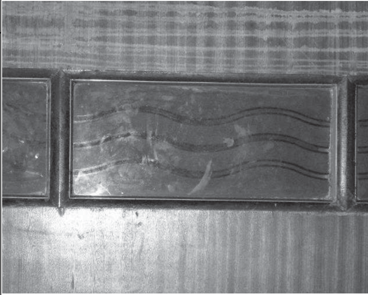
Plate 48: Admin block, entrance hall, decorative glass in doors (Full report, para.3.11)
