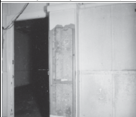
Frame 10: Admin, S upper corridor Concrete stanchion opp. Room 46
