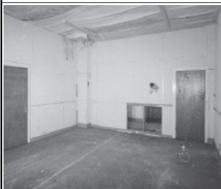
Frame 10: Admin Block, 1st floor Room 75, facing NE
