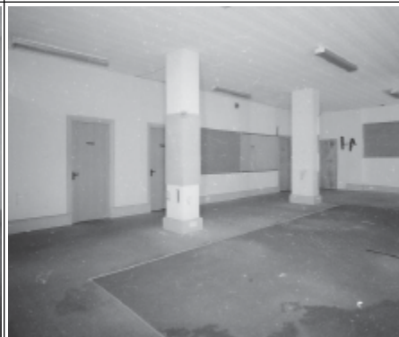
Frame 12: Admin Block, G floor Room 19, facing SE
