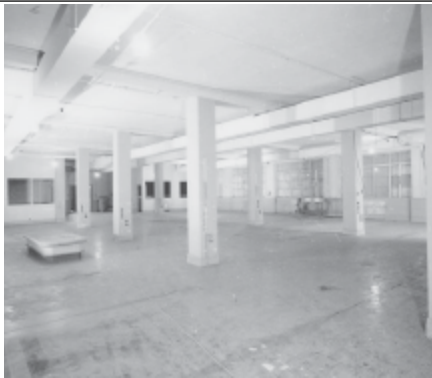
Frame 5: Canteen, G floor Dining room, facing SW
