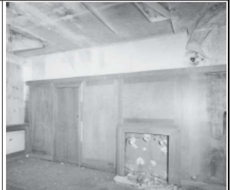
Frame 6: Admin Block, 1st floor Room 49, facing SE
