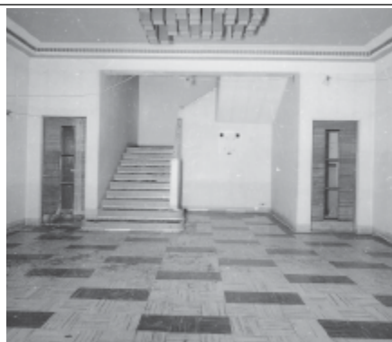
Frame 11: Admin Block, G floor Entrance Hall, facing W
