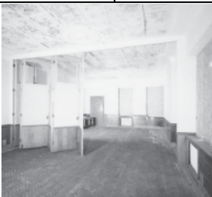
Frame 2: Canteen, 1st floor Managers' Common Room, facing NW
