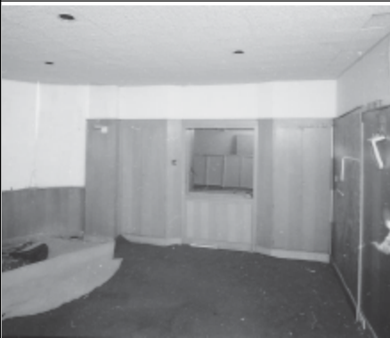
Frame 4: Admin Block, G floor Room 11, facing S
