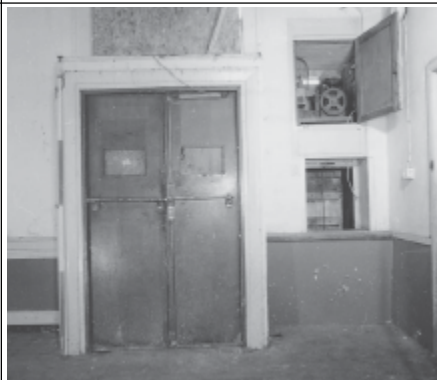
Frame 5: Canteen Ballroom, fire door & dumb waiter
