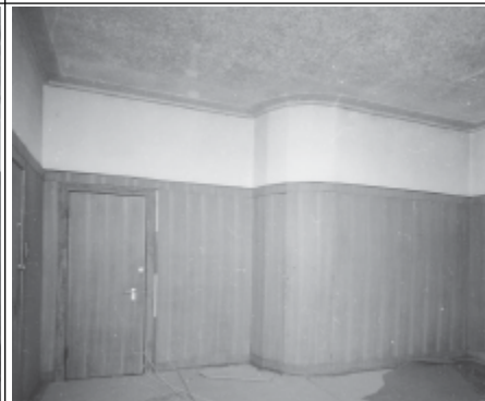
Frame 9: Admin Block, G floor Room 1, facing N
