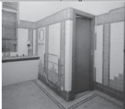
Frame 5: Admin Block, G floor WC adj. Room 32, facing NW
