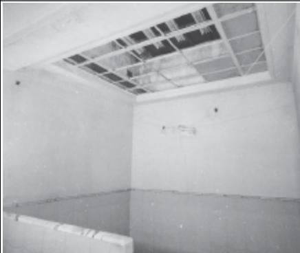
Frame 8: Admin Block, 1st floor Skylight above stairwell, facing SW
