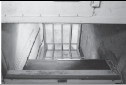
Frame 2: Admin Block, Cellar Interior of vault, facing SE
