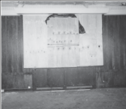
Frame 4: Admin Block, 1st floor Board Room, facing E
