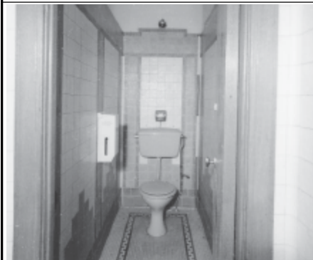
Frame 7: Admin Block, G floor WC adj. Room 32, N cubicle, facing W
