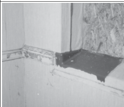
Frame 11: Admin, S upper corridor Moulded ceramic window sill, detail
