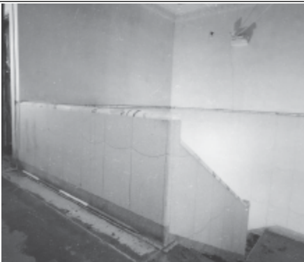
Frame 10: Admin Block, 1st floor Head of main staircase
