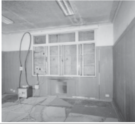
Frame 2: Admin Block, G floor Room 1, facing S
