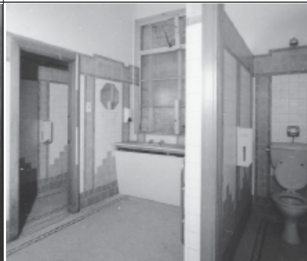
Frame 6: Admin Block, G floor WC adj. Room 32, facing SW
