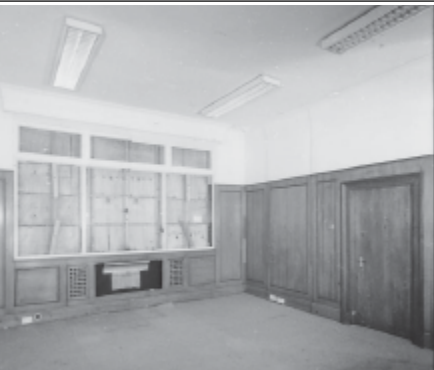
Frame 7: Admin Block, G floor Room 5, facing SE
