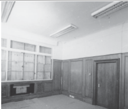
Frame 11: Admin Block, G floor Room 5, facing SE
