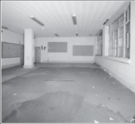
Frame 1: Admin Block, G floor Room 19, facing S
