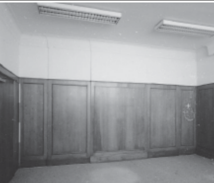
Frame 10: Admin Block, G floor Room 5, facing N
