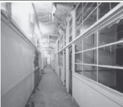
Frame 5: Admin Block, 1st floor S corridor, facing N
