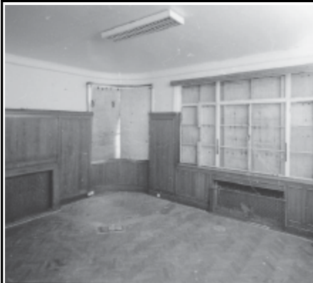
Frame 1: Admin Block, G floor Room 7, facing SE
