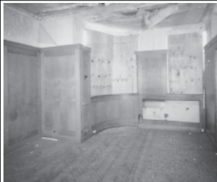
Frame 7: Admin Block, 1st floor Room 49, facing NE
