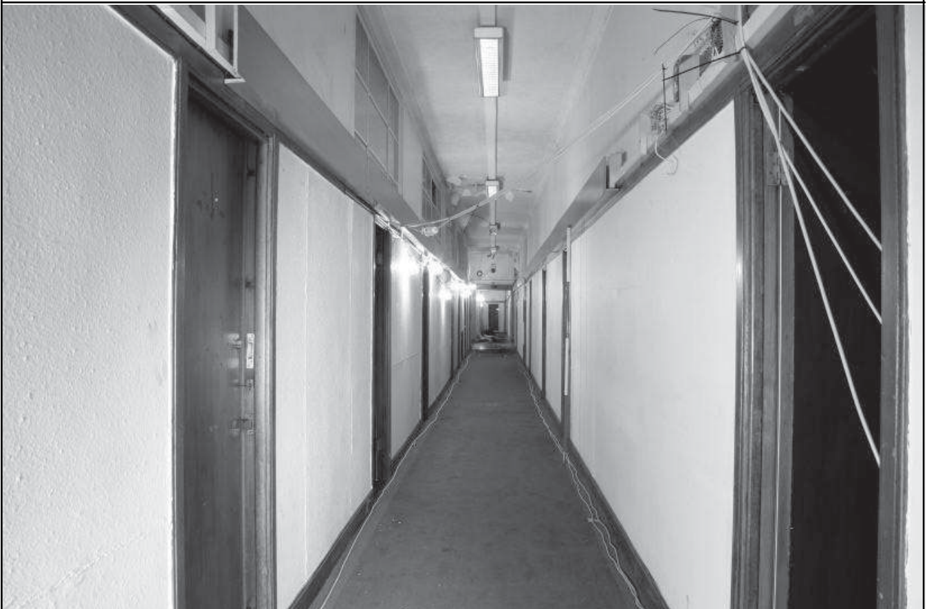
Plate 40: Admin block, ground floor, southern corridor, looking N (Full report, para.3.12)
