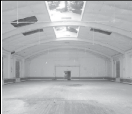
Frame 5: Canteen, 1st floor Ballroom, facing S
