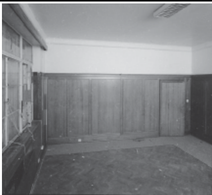
Frame 2: Admin Block, G floor Room 7, facing S
