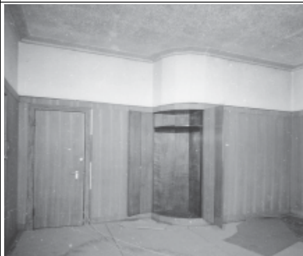
Frame 8: Admin Block, G floor Room 1, facing N
