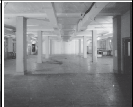
Frame 12: Canteen, G floor Dining room, facing N
