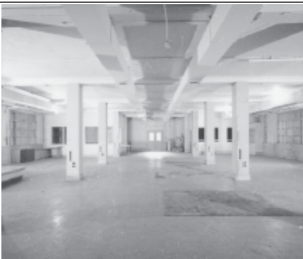
Frame 8: Canteen, G floor Dining room, facing S
