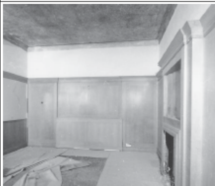
Frame 5: Admin Block, G floor Room 38, facing W
