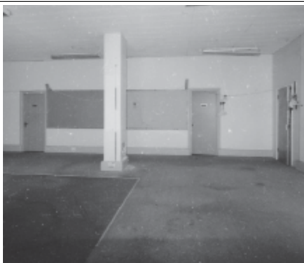
Frame 11: Admin Block, G floor Room 19, facing E
