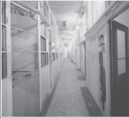
Frame 1: Admin Block, 1st floor S corridor, facing S
