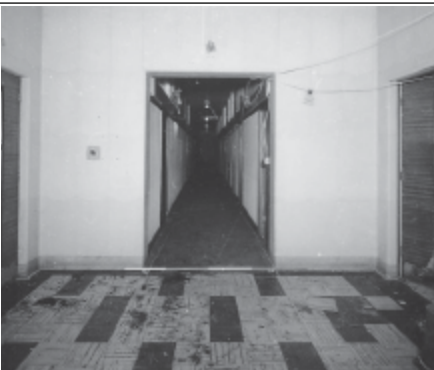
Frame 8: Admin Block, G floor Entrance Hall, facing S
