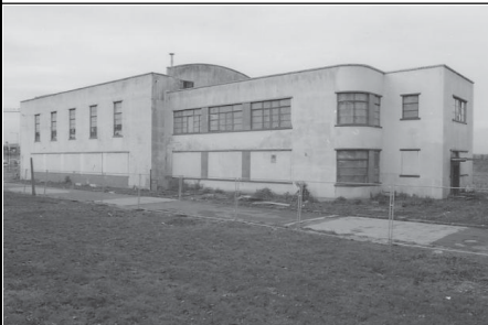
Frame 7: Canteen, N & E ext. elevations
