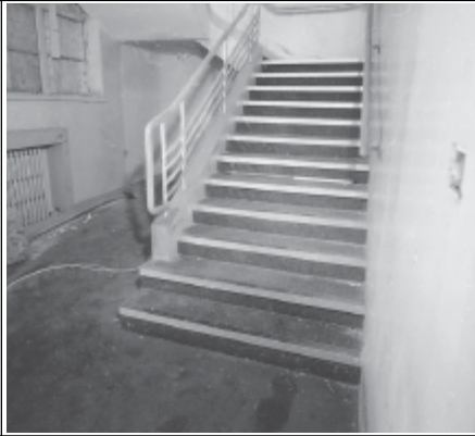
Frame 2: Canteen, G floor S staircase, facing W
