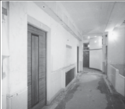
Frame 5: Admin Block, 1st floor Landing, facing S
