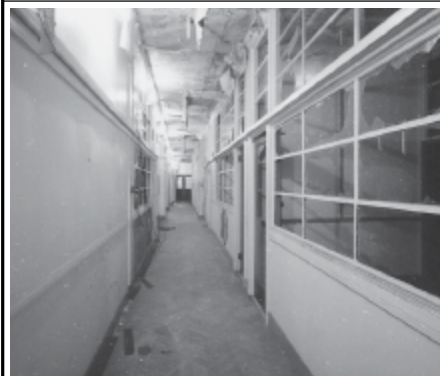
Frame 4: Admin Block, 1st floor S corridor, facing N
