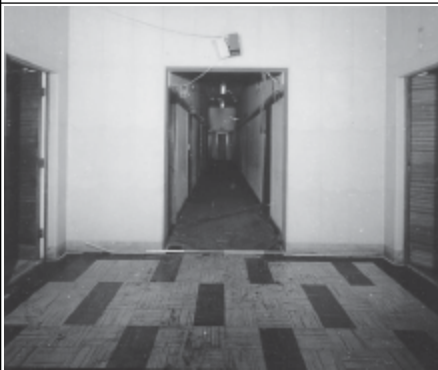
Frame 7: Admin Block, G floor Entrance Hall, facing N
