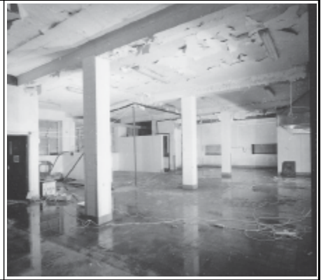
Frame 3: Canteen, G floor Kitchen, S end, facing SE
