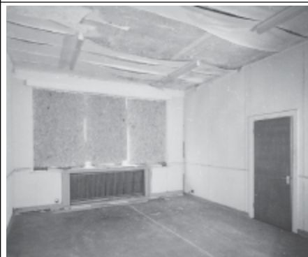
Frame 9: Admin Block, 1st floor Room 75, facing NW
