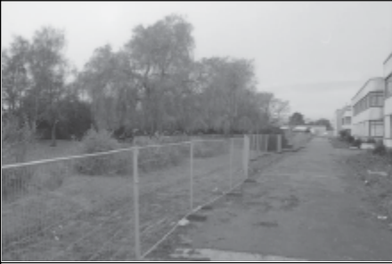
Frame 4: E elevations & apron, looking S
