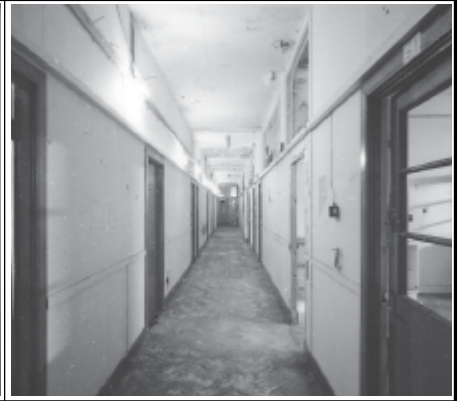
Frame 3: Admin Block, 1st floor N corridor, facing S
