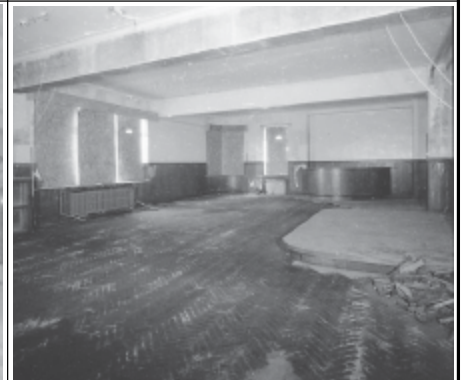
Frame 6: Canteen, 1st floor NW managers' dining room, facing NW
