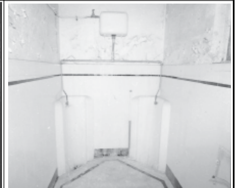
Frame 9: Canteen, G floor Gents' lavatory adj. N entrance, facing N
