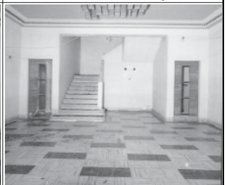
Frame 12: Admin Block, G floor Entrance Hall, facing W
