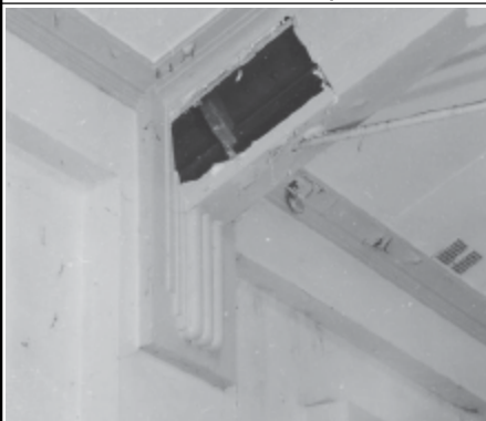
Frame 4: Canteen Ballroom, boxed roof truss
