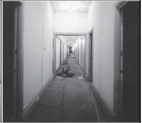
Frame 3: Admin Block, G floor N corridor, facing S
