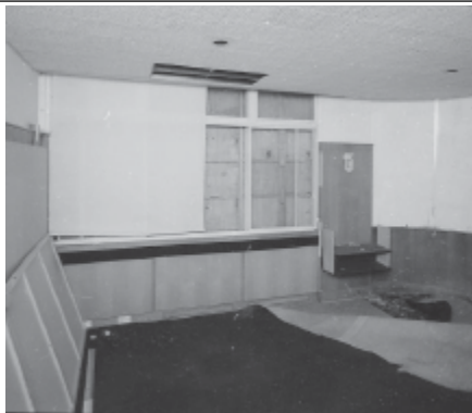
Frame 5: Admin Block, G floor Room 11, facing E
