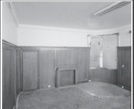
Frame 12: Admin Block, G floor Room 7, facing N
