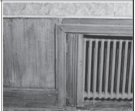
Frame 6: Canteen Reeded radiator enclosure flap
