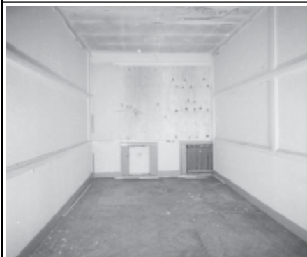
Frame 7: Admin Block, 1st floor Room 47, facing E
