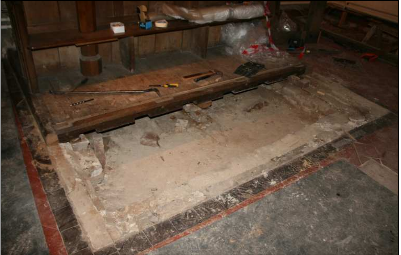
Plate 1: Removal of the pews, looking north-west
