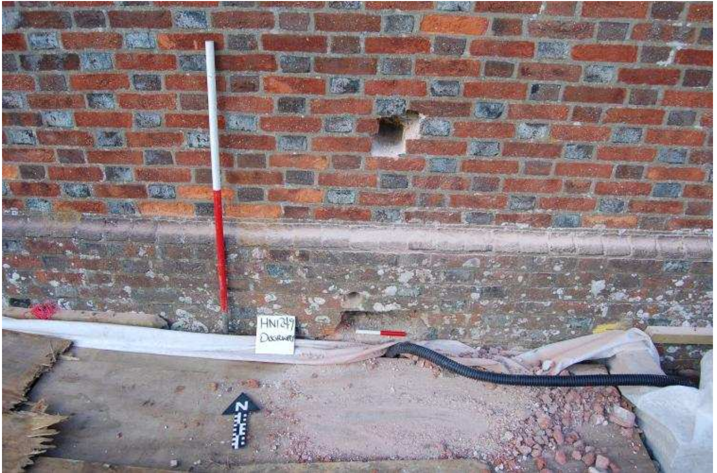
Plate 013 - Test holes for new doorway, looking N
