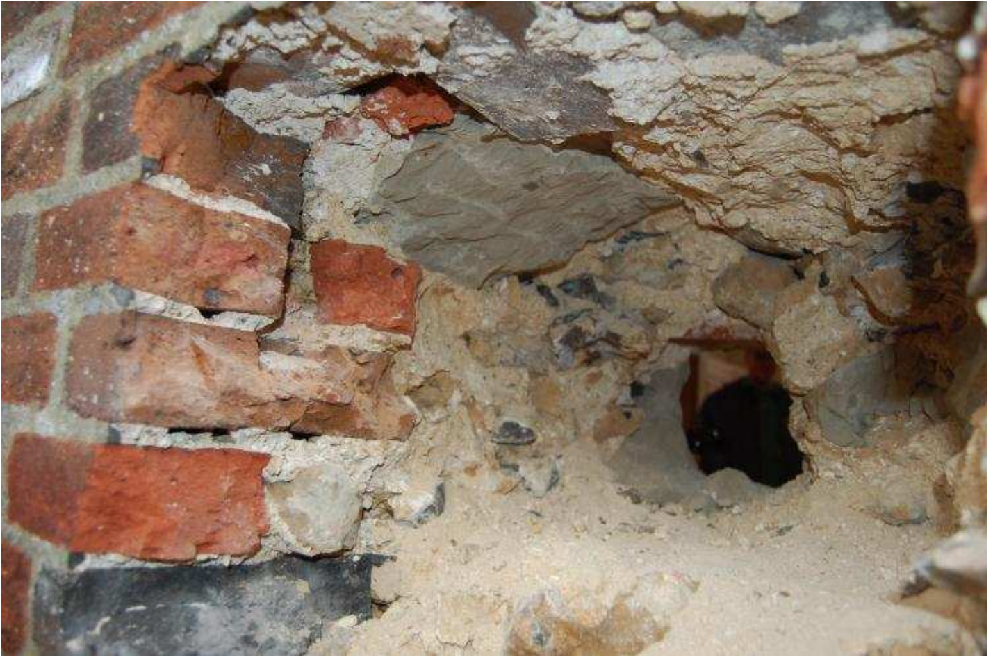
Plate 017 - Section through south wall of nave, looking N
