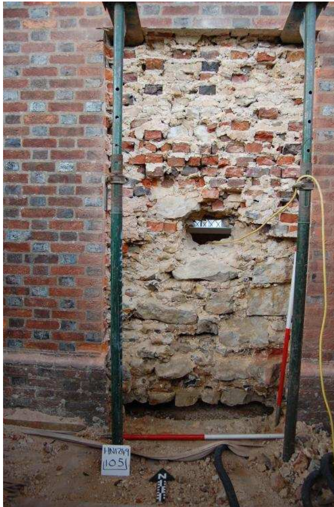
Plate 015 - New doorway after removal of exterior brick facing
