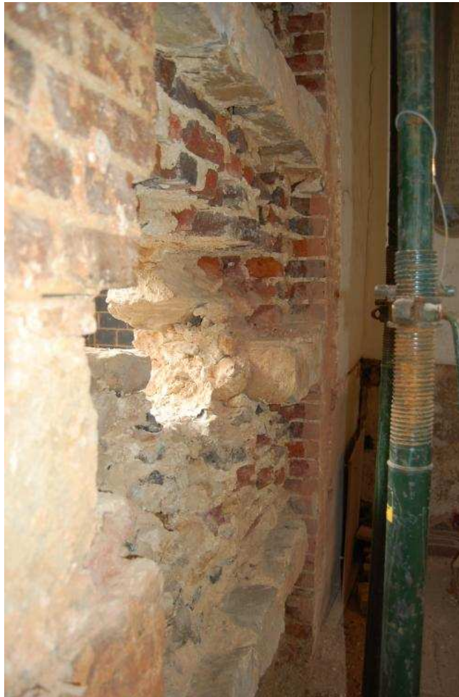
Plate 019 - Detail of stone coursing on internal elevation, looking W
