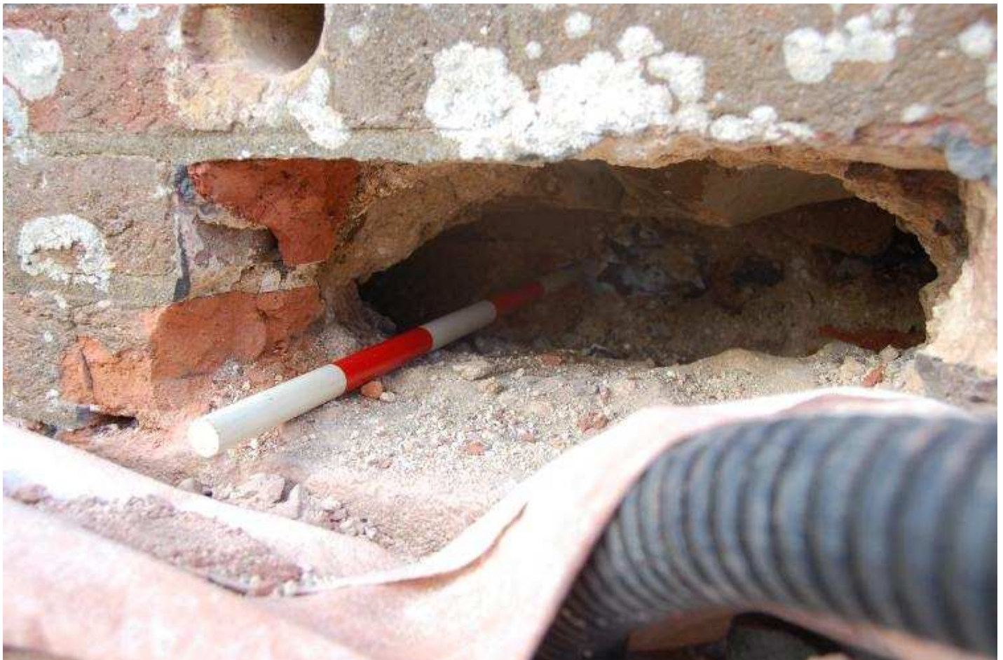
Plate 014 - Test hole, showing earlier wall, looking NW (c) The Heritage Network Ltd.
