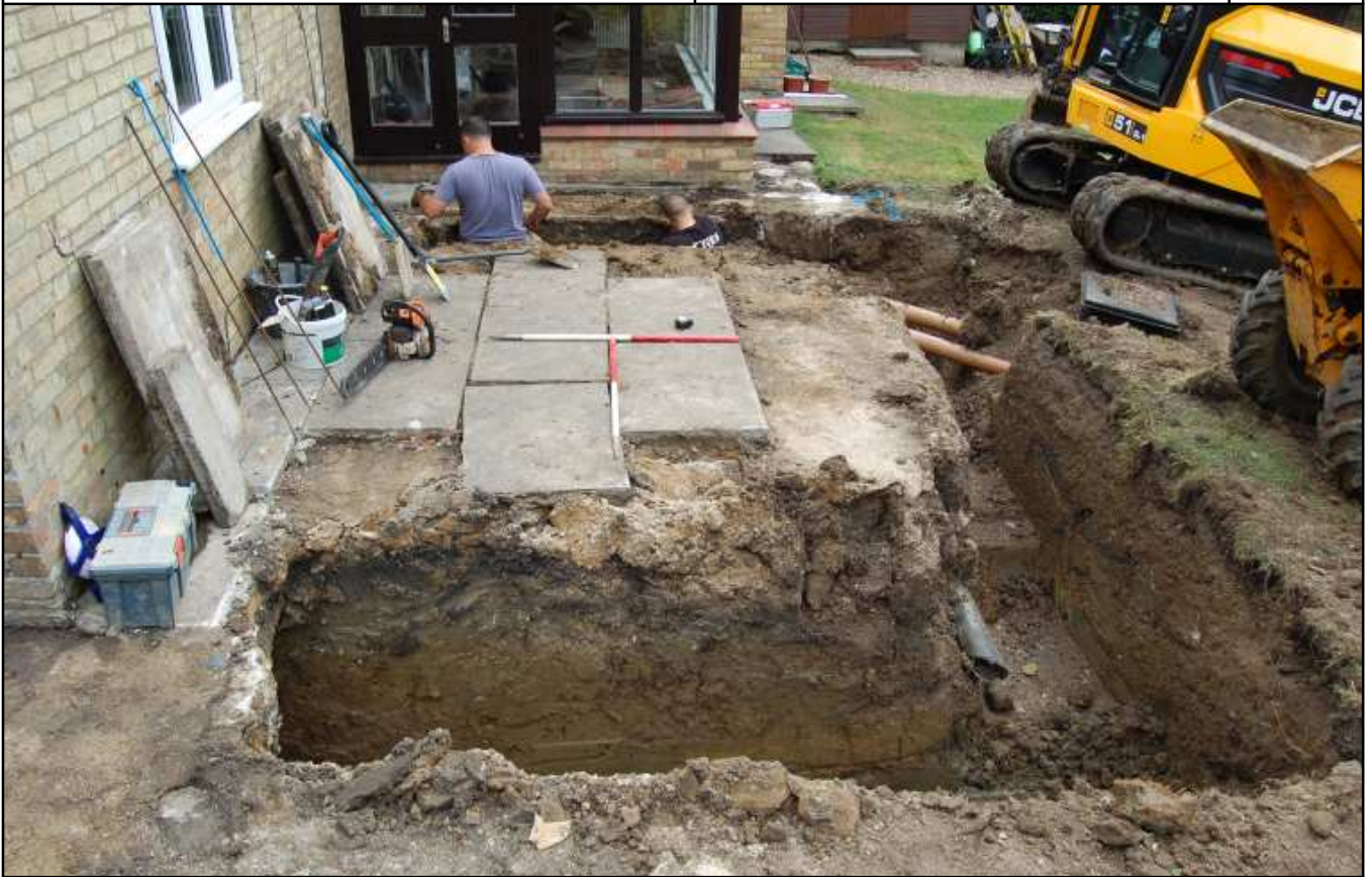
Plate 1: General shot of extension, looking W
