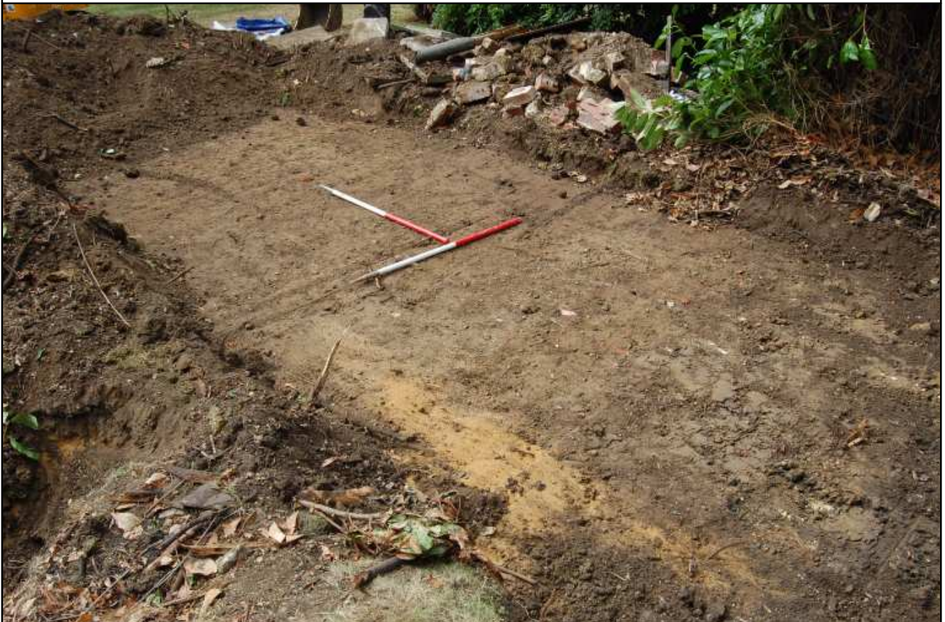
Plate 4: Ground reduction for new driveway, looking SW
