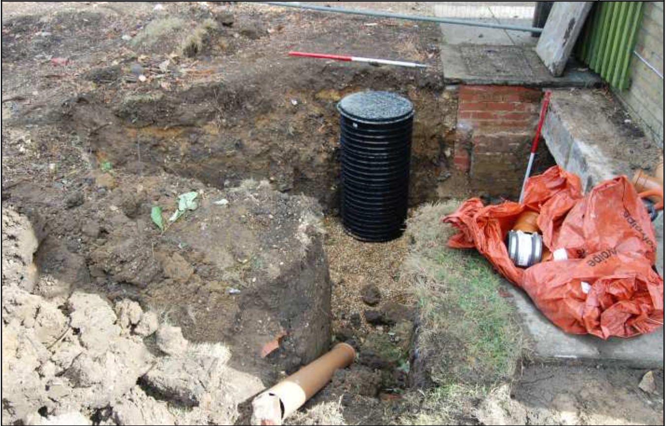
Plate 3: Excavation for new drainage access, looking NE
