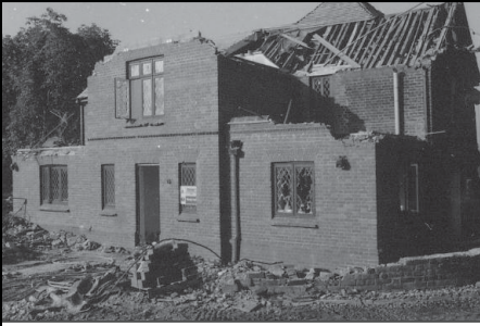
Frame 1: Southern and eastern elevations looking north west
