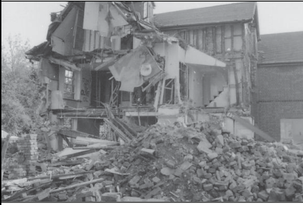
Frame 4: Northern elevation looking south
