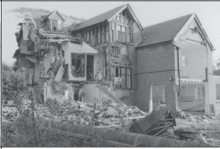
Frame 5: Northern and western elevations looking south east
