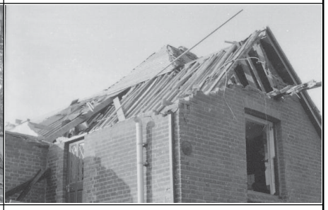
Frame 15: Southern and eastern elevations looking north west
