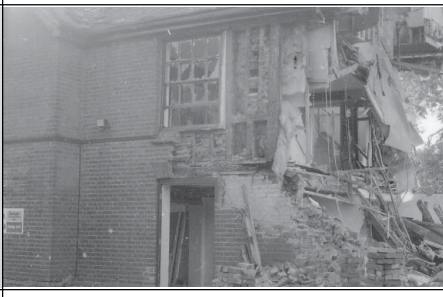
Frame 14: Northern and eastern elevations looking south west
