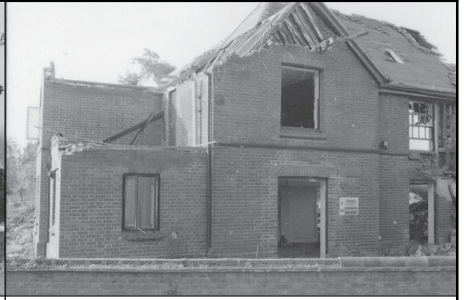
Frame 3: Eastern elevation looking west
