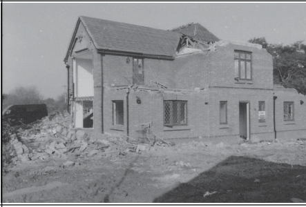
Frame 8: Southern and western elevations looking north east
