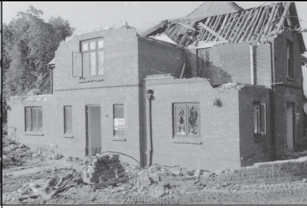
Frame 2: Southern and eastern elevations looking north west
