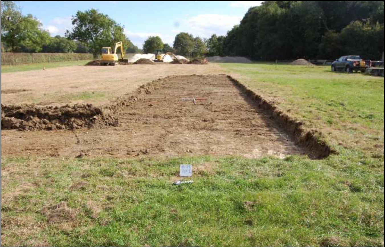
Plate 3: Stripped transect for manège, looking east
