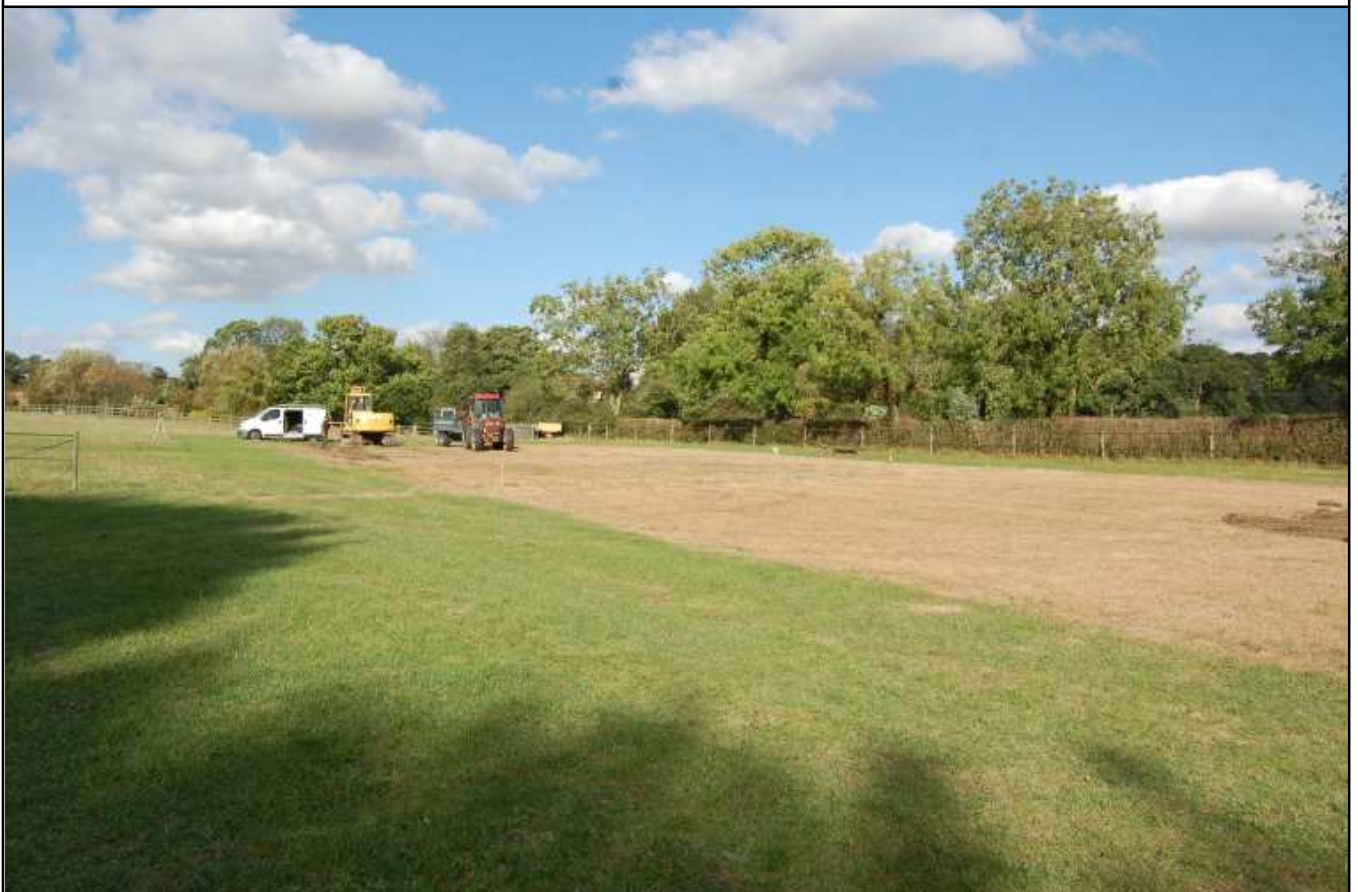
Plate 2: Pre-excitation view of area for manège, looking west
