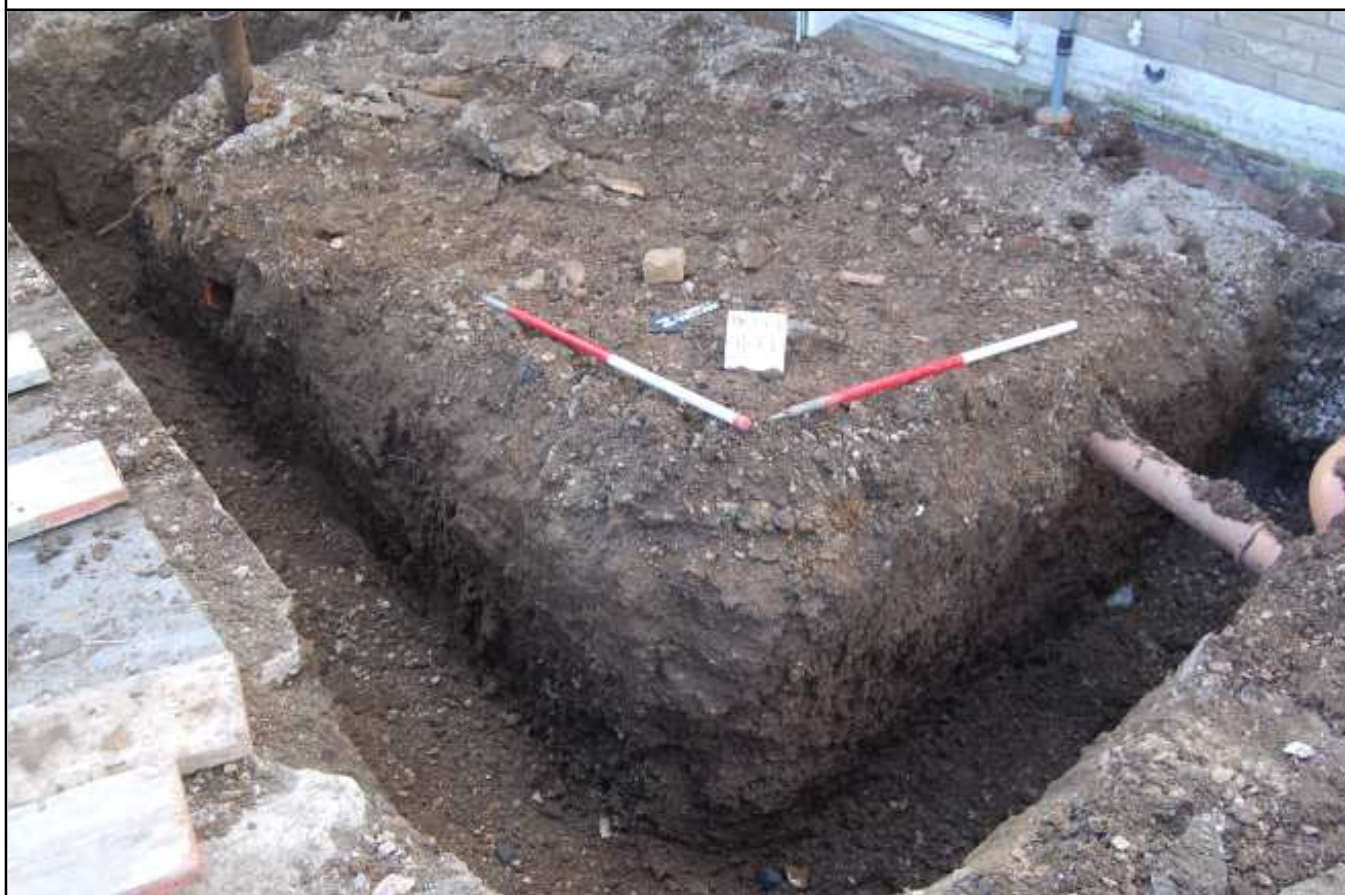
Plate 2: Footing trenches, looking SE
