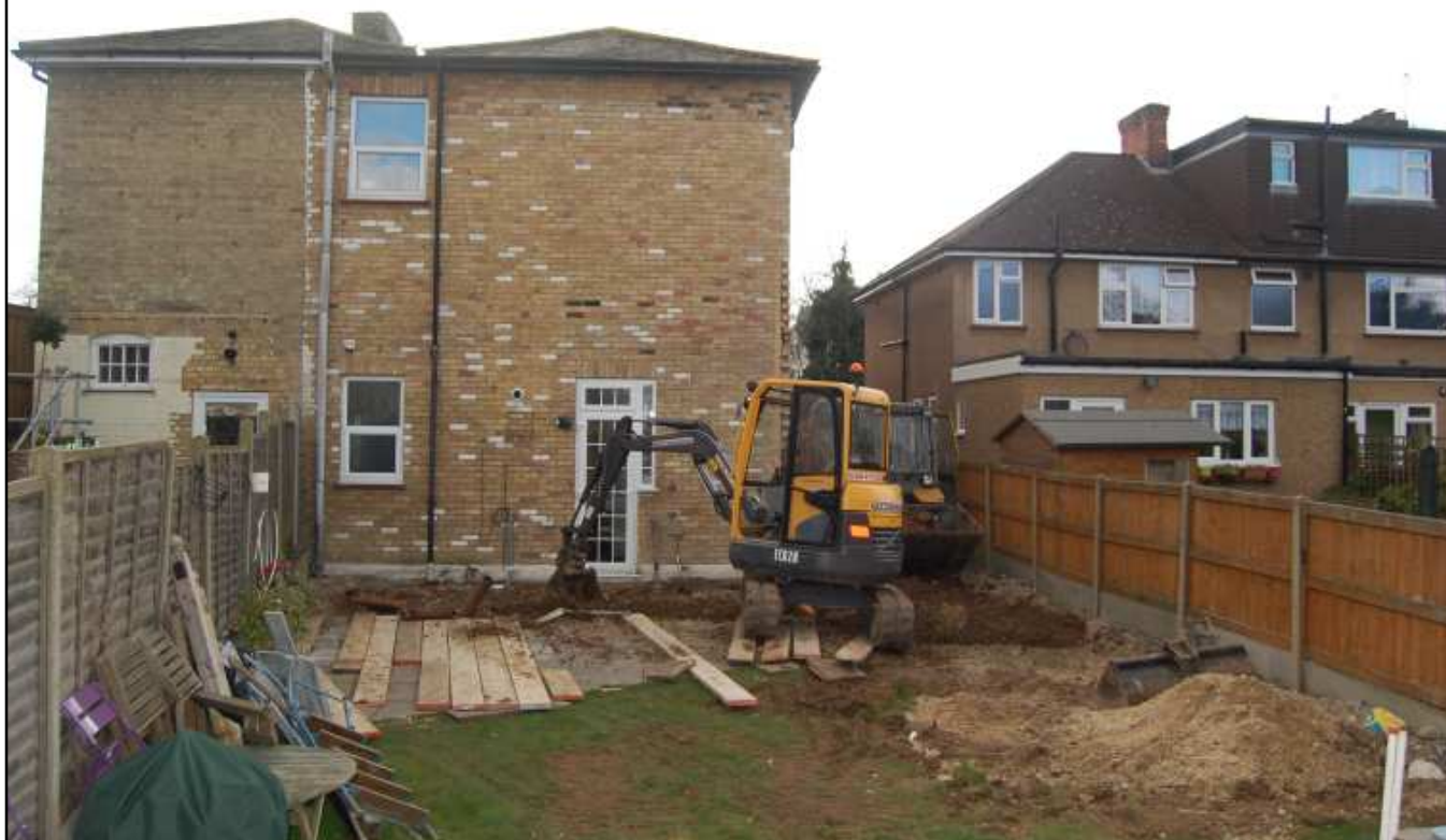
Plate 1: Development site, looking S
