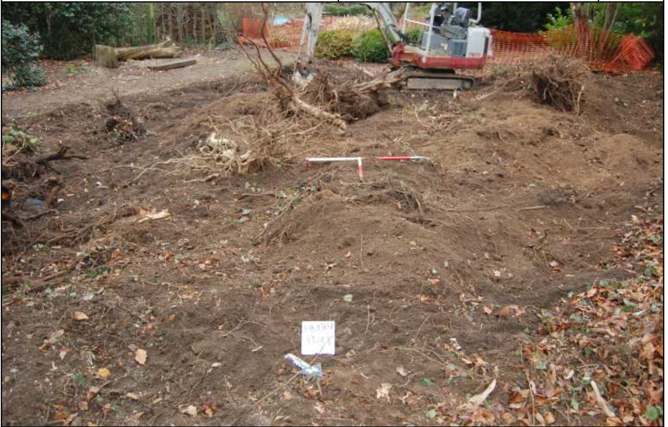
Plate 1: Area of tree removal, looking south-west
