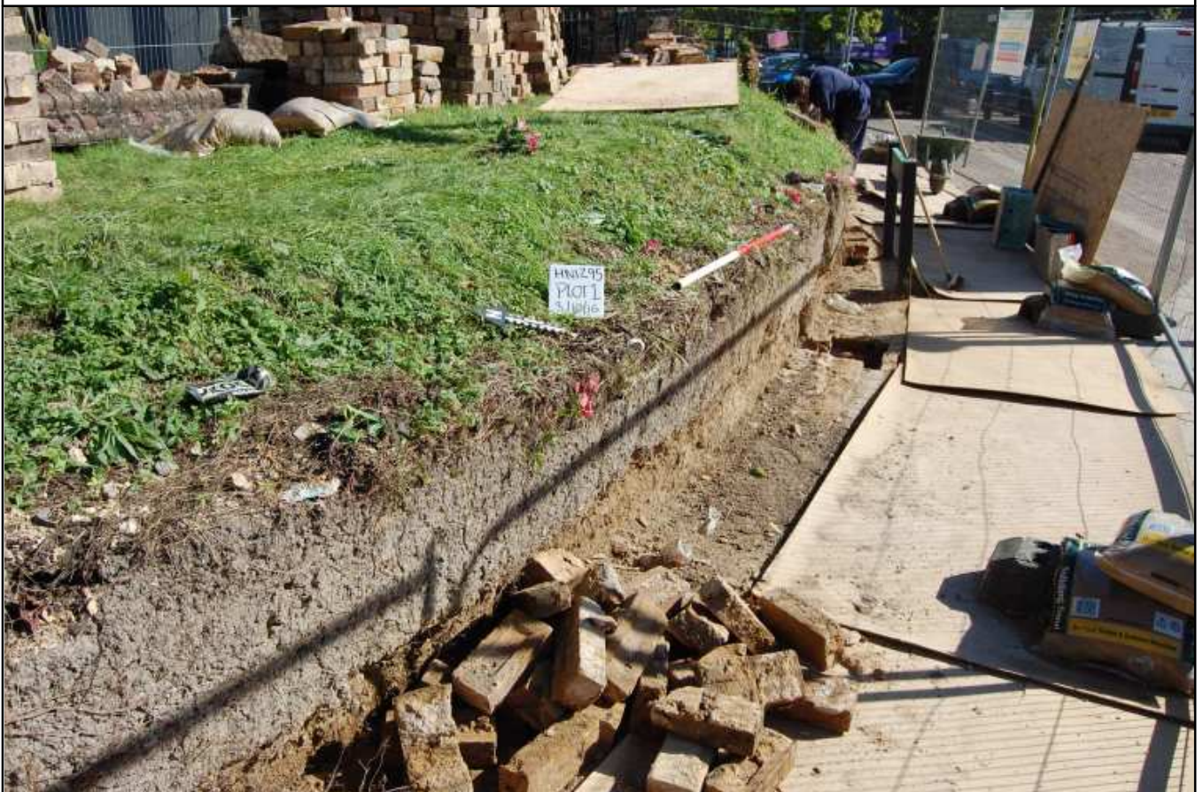
Plate 2: Soil face of graveyard after wall removal, looking east
