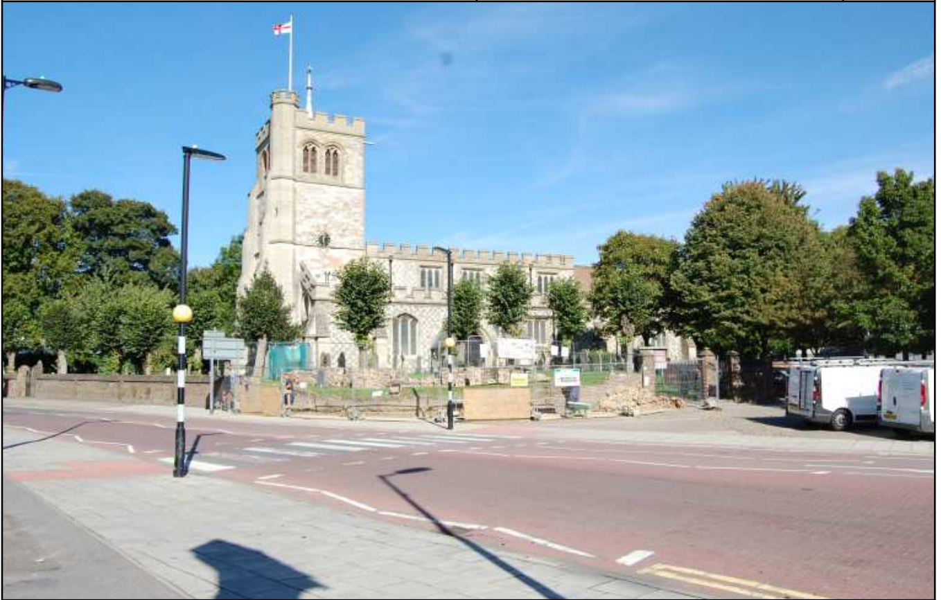
Plate 1: All Saints Church, showing removal of graveyard wall in foreground, looking north-east
