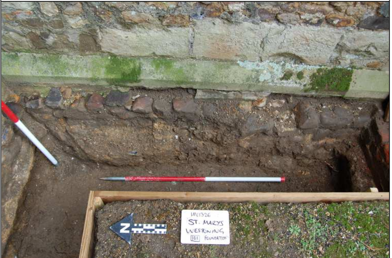
Plate 2: Wall foundations looking east
