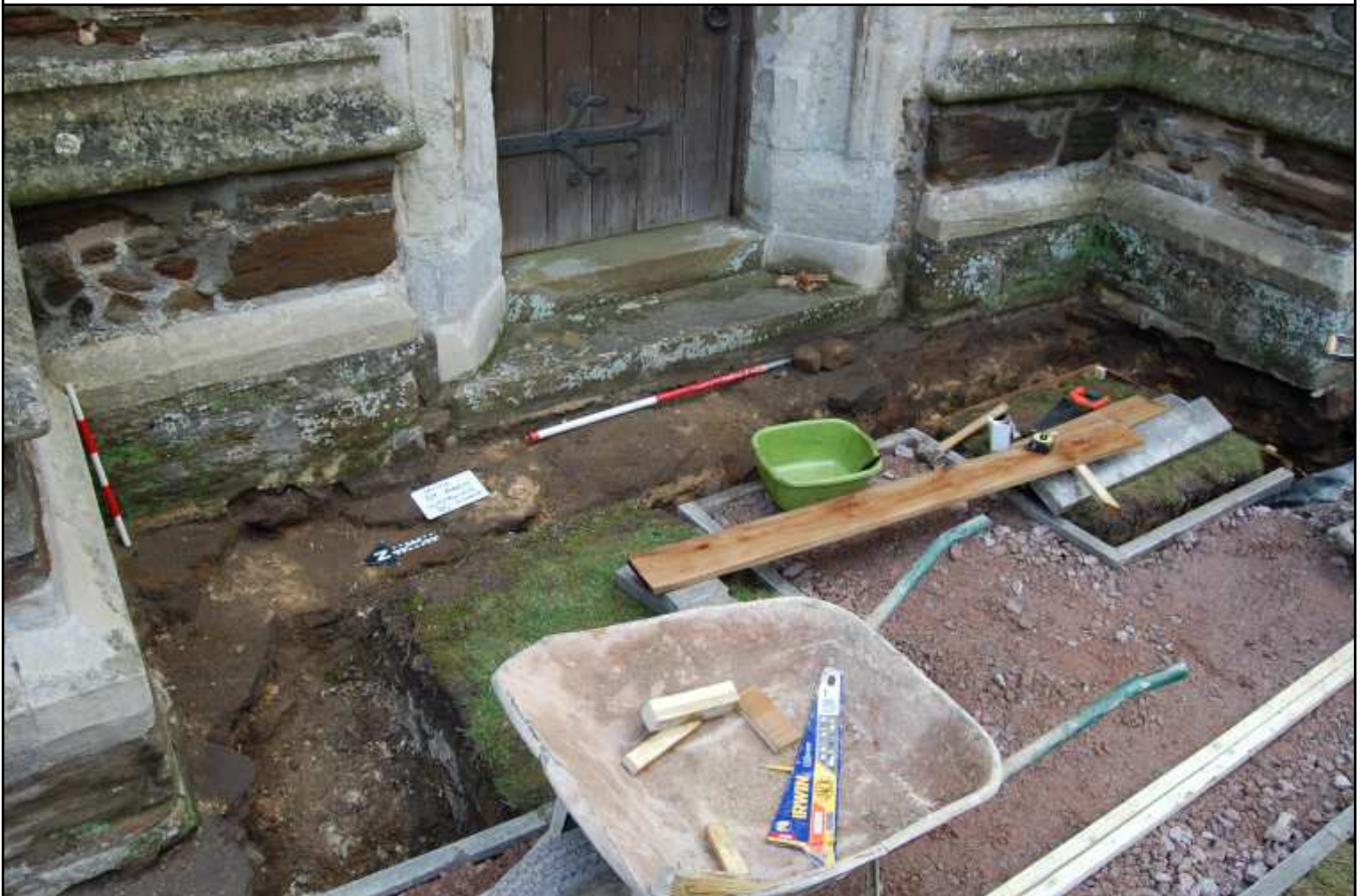
Plate 4: West entrance wall foundations looking southeast
