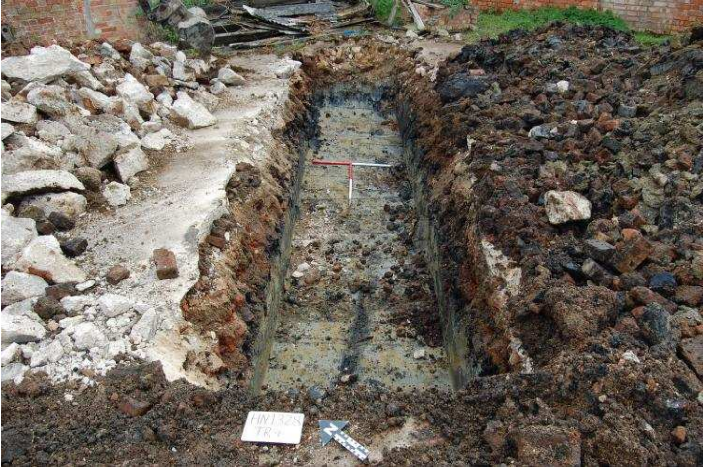
Plate 09 - Trench 4, looking NE
