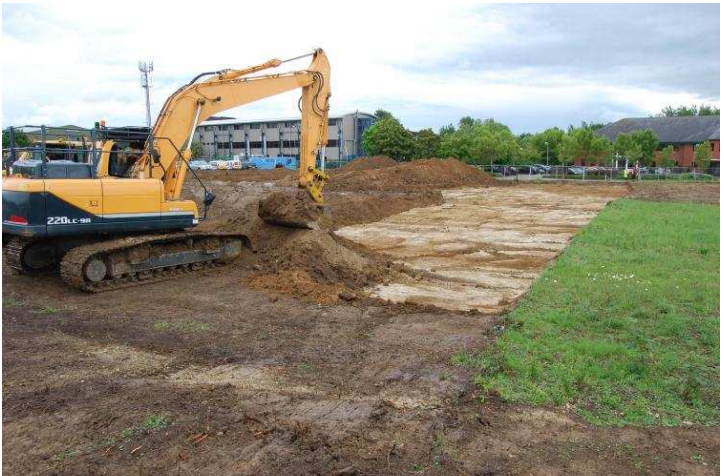
Plate 02 - Access road during ground reduction, looking SE
