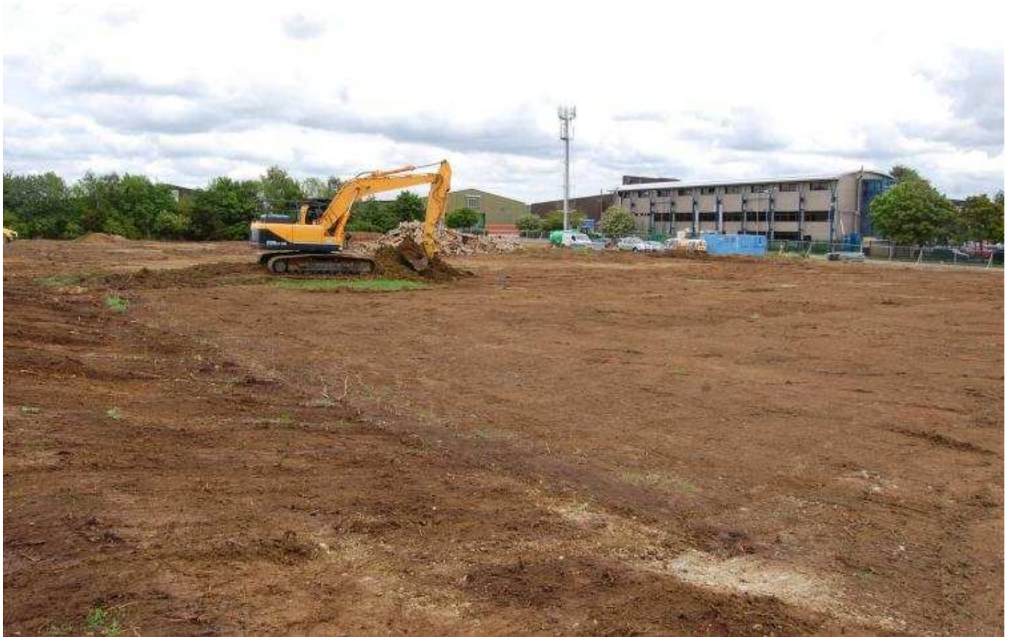
Plate 01 - Zone 5 during the vegetation strip, looking SE
