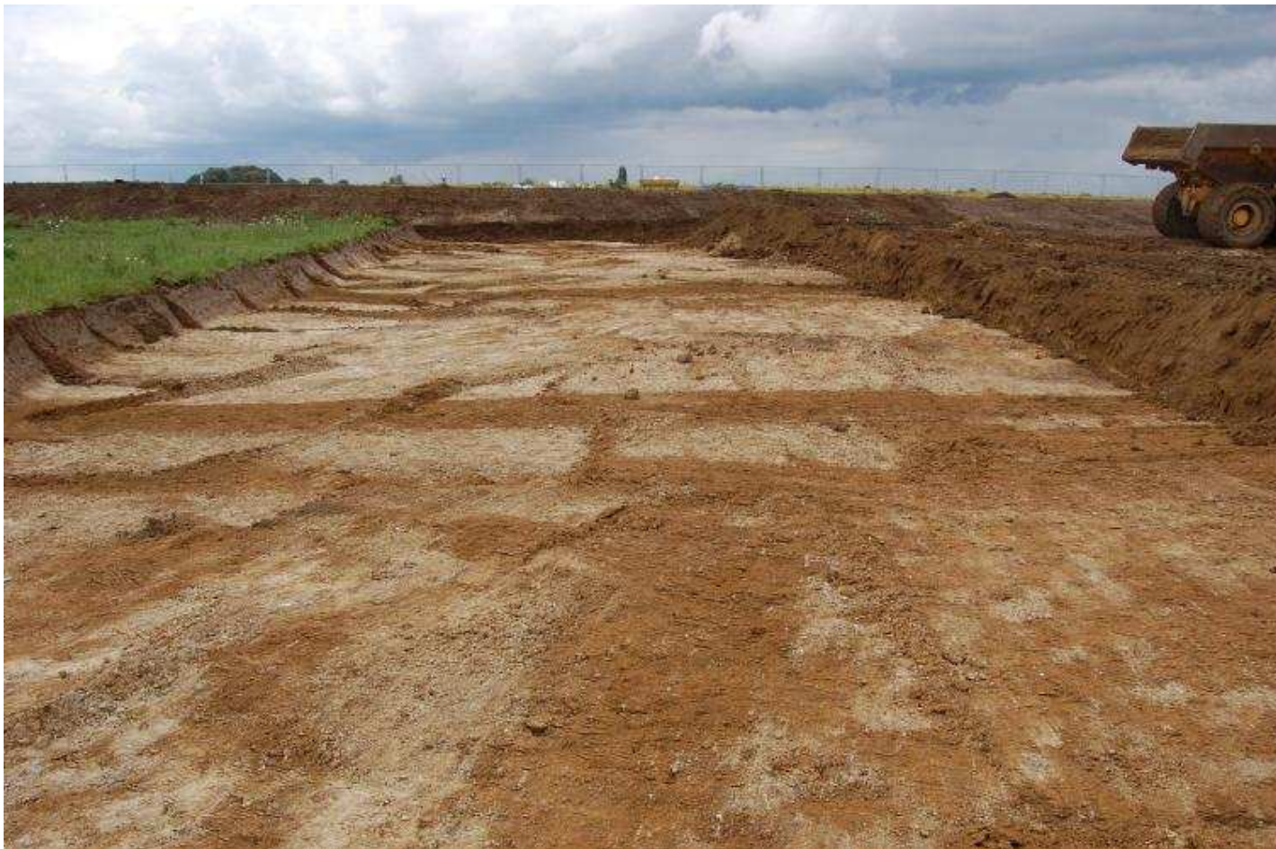
Plate 03 - Access road following ground reduction, looking NW
