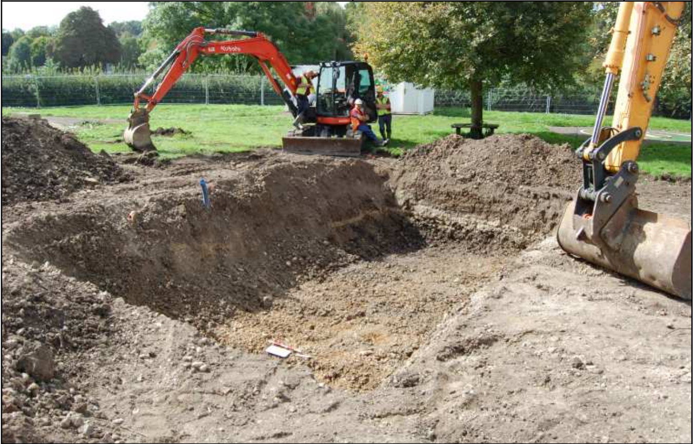
Plate 1: Water tank trench, looking SW
