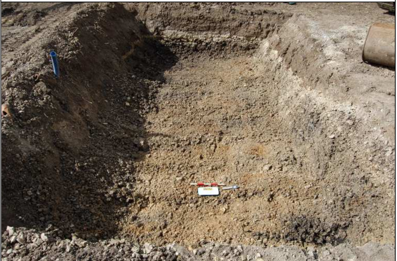
Plate 2: Water tank trench, looking W
