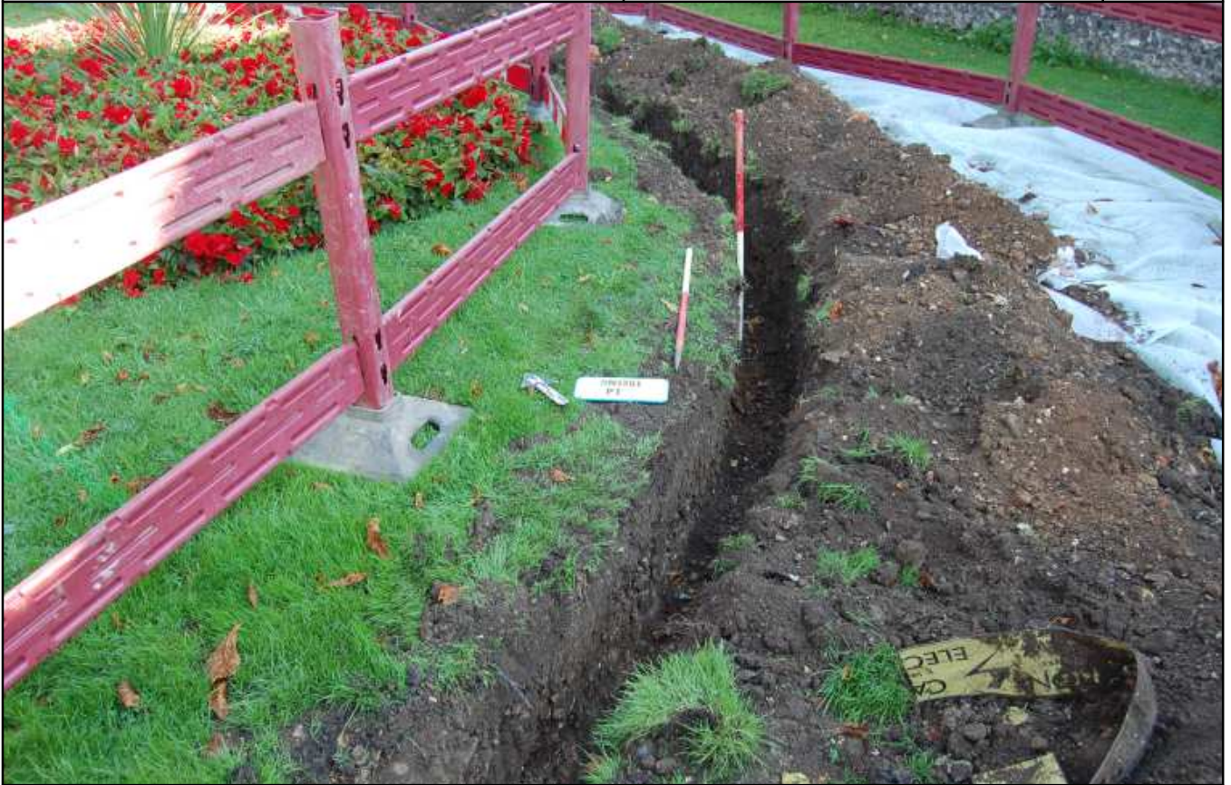
Plate 9: Electrical service trench, looking NE
