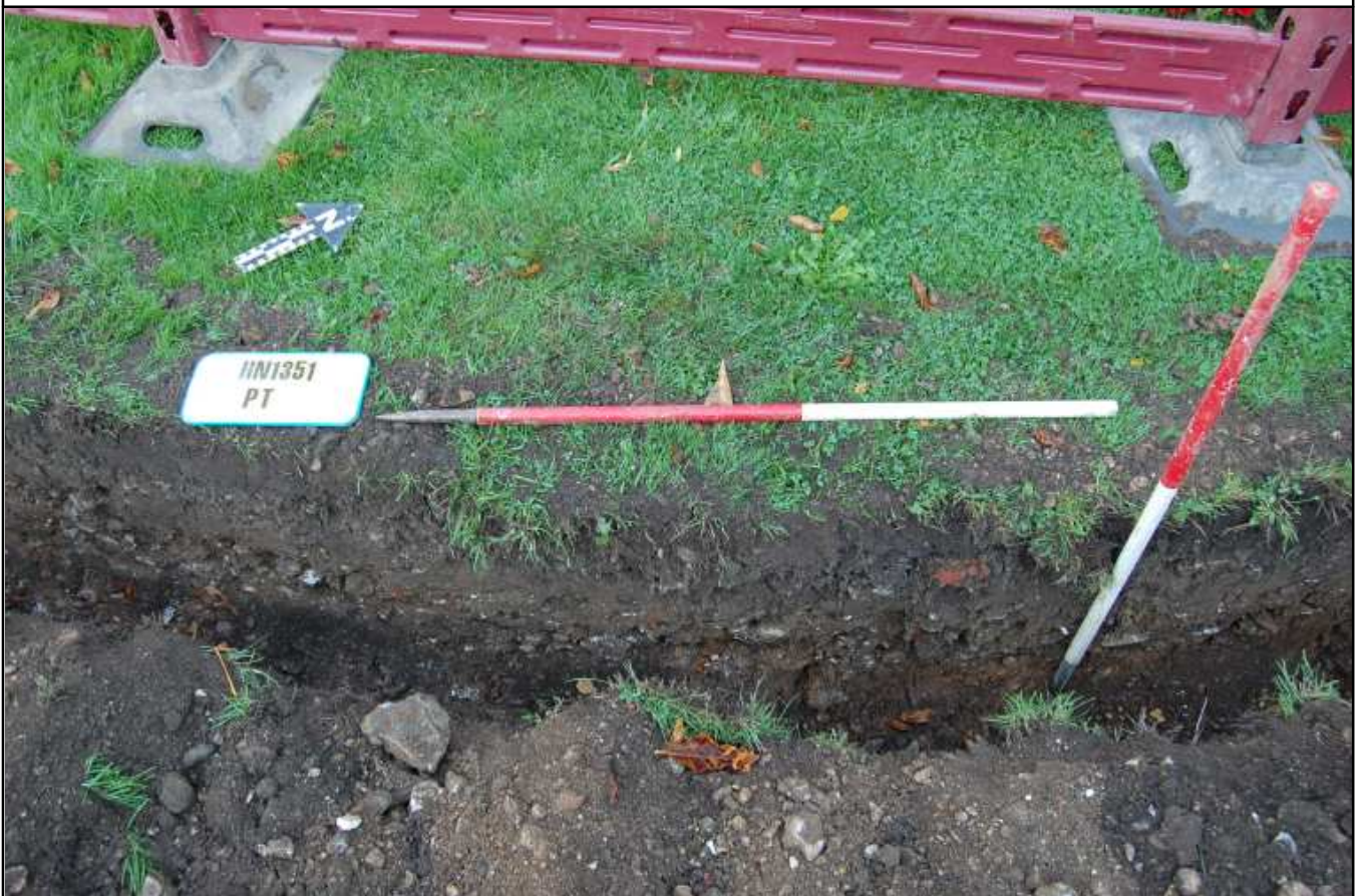
Plate 10: Electrical service trench stratigraphy, looking NW
