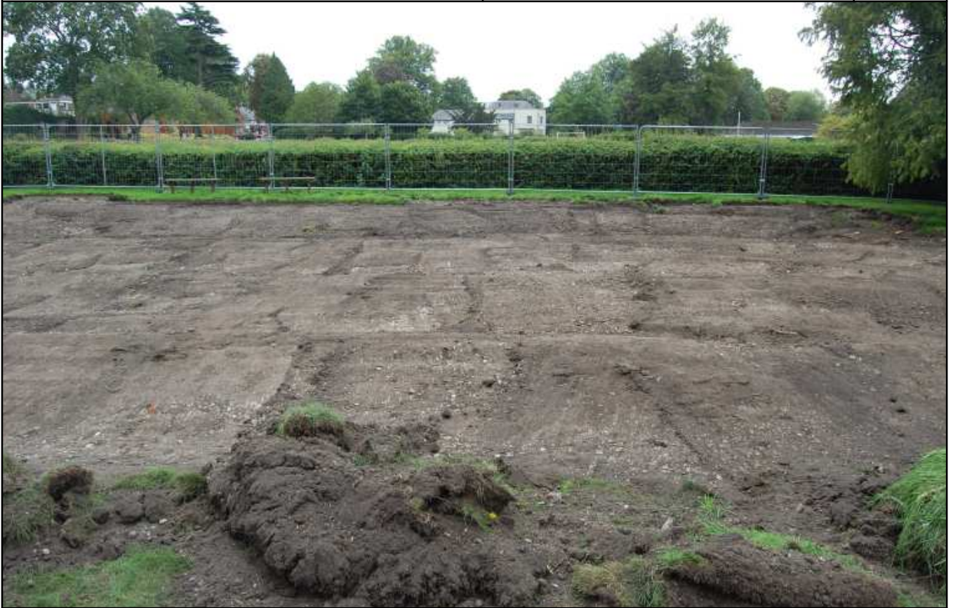
Plate 5: Turf strip on splash park footprint, looking S
