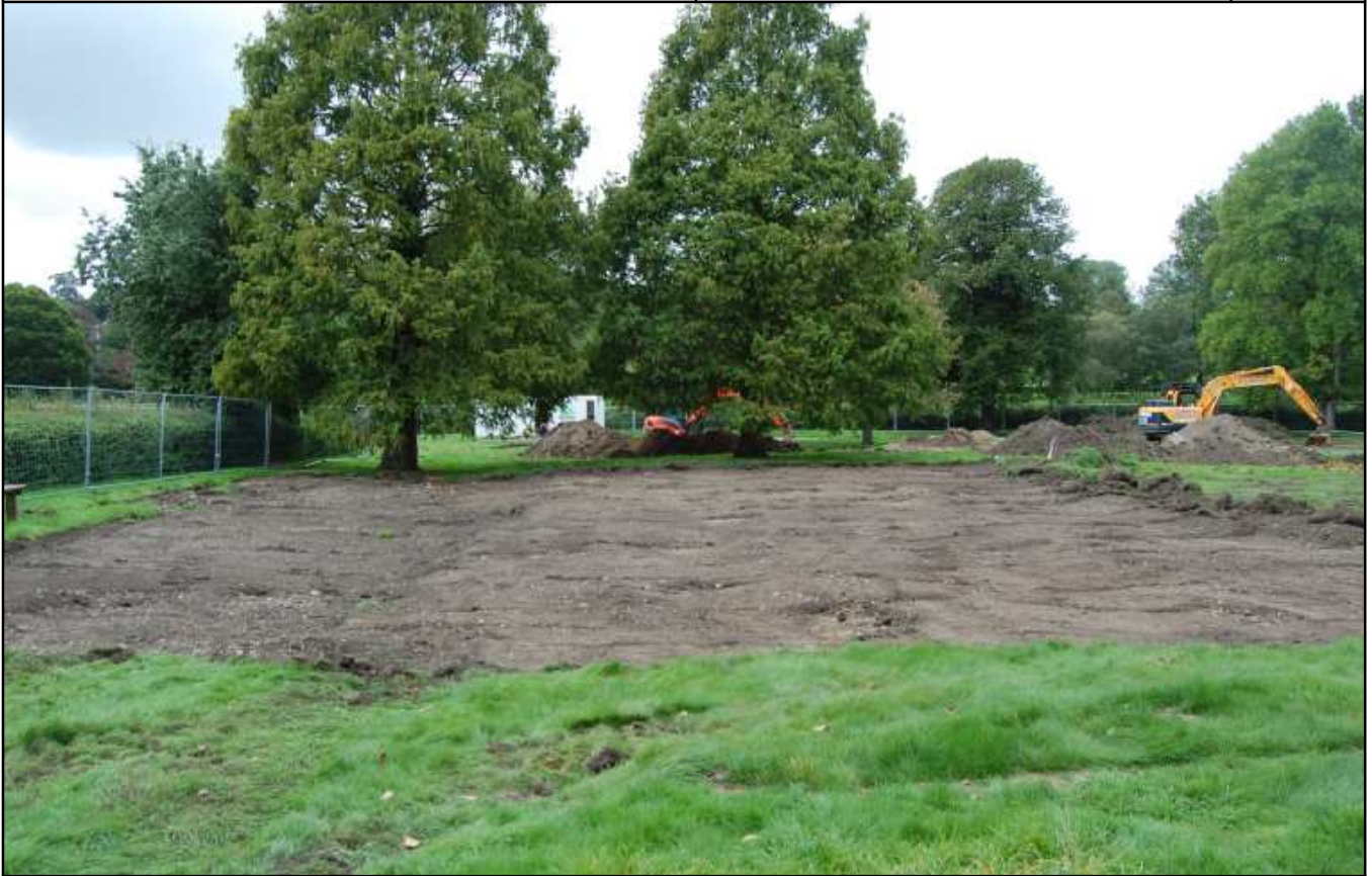
Plate 7: Turf strip on splash park footprint, looking W
