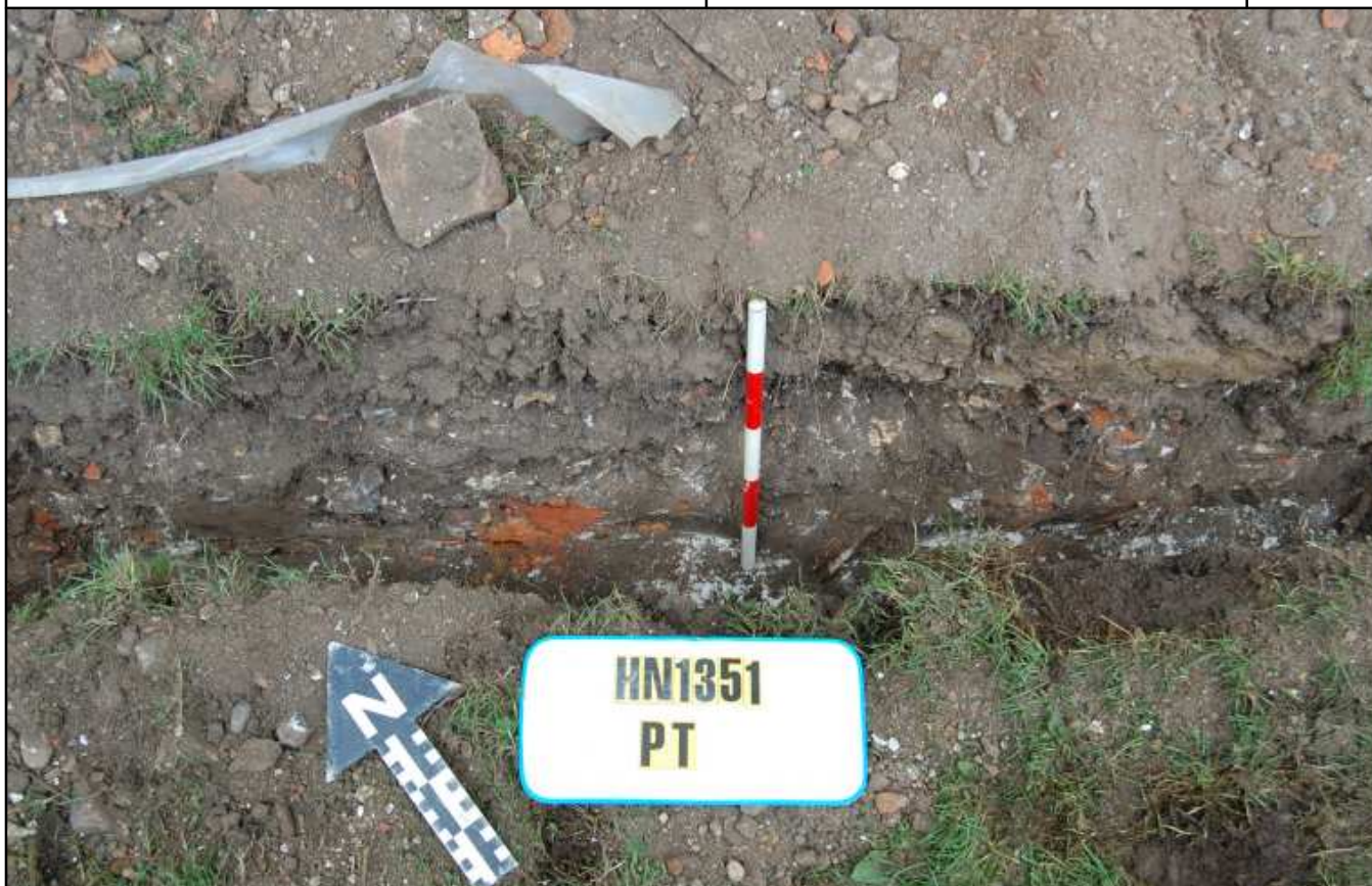
Plate 11: Electrical service trench stratigraphy, looking NE
