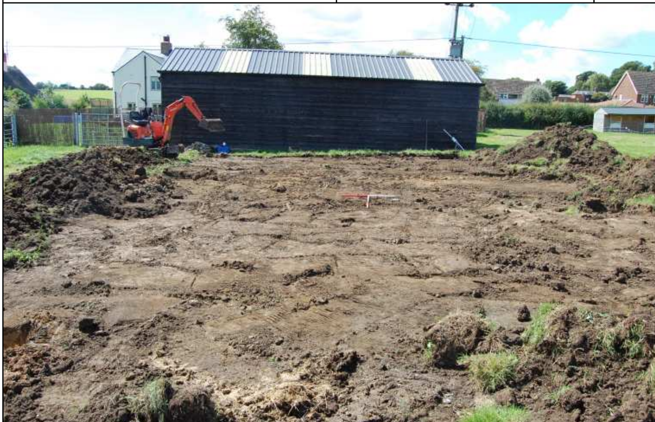
Plate 9: Building footprint following topsoil strip, looking SW
