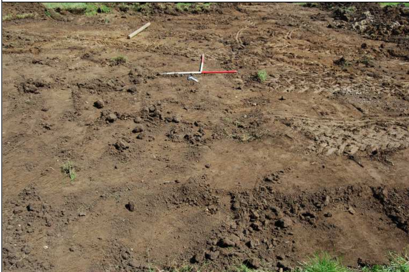
Plate 10: Building footprint following topsoil strip, looking NE
