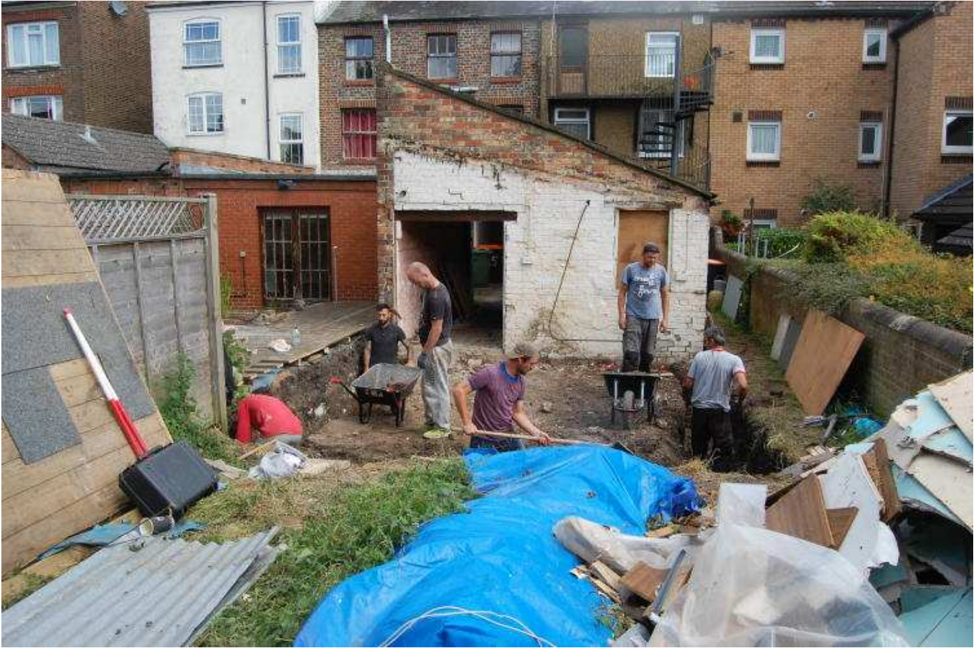
Plate 01 - working shot of footing trenches, looking NE
