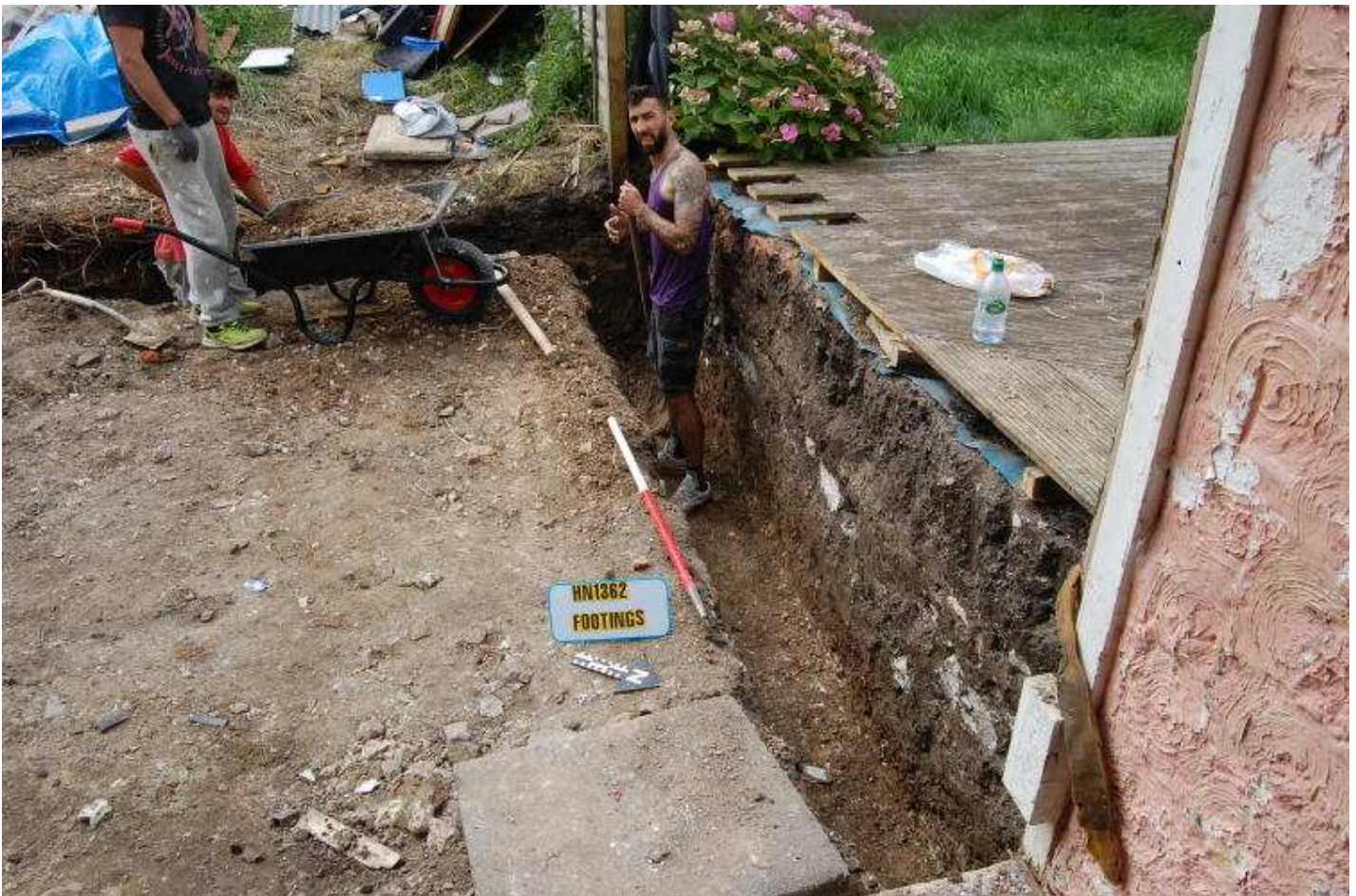
Plate 02 - Footing trench, looking SW
