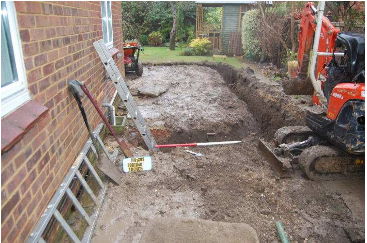
Plate 01 - Foundation trenches, looking SW
