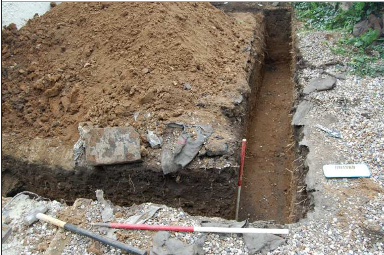
Plate 2: Foundation trenches looking SW
