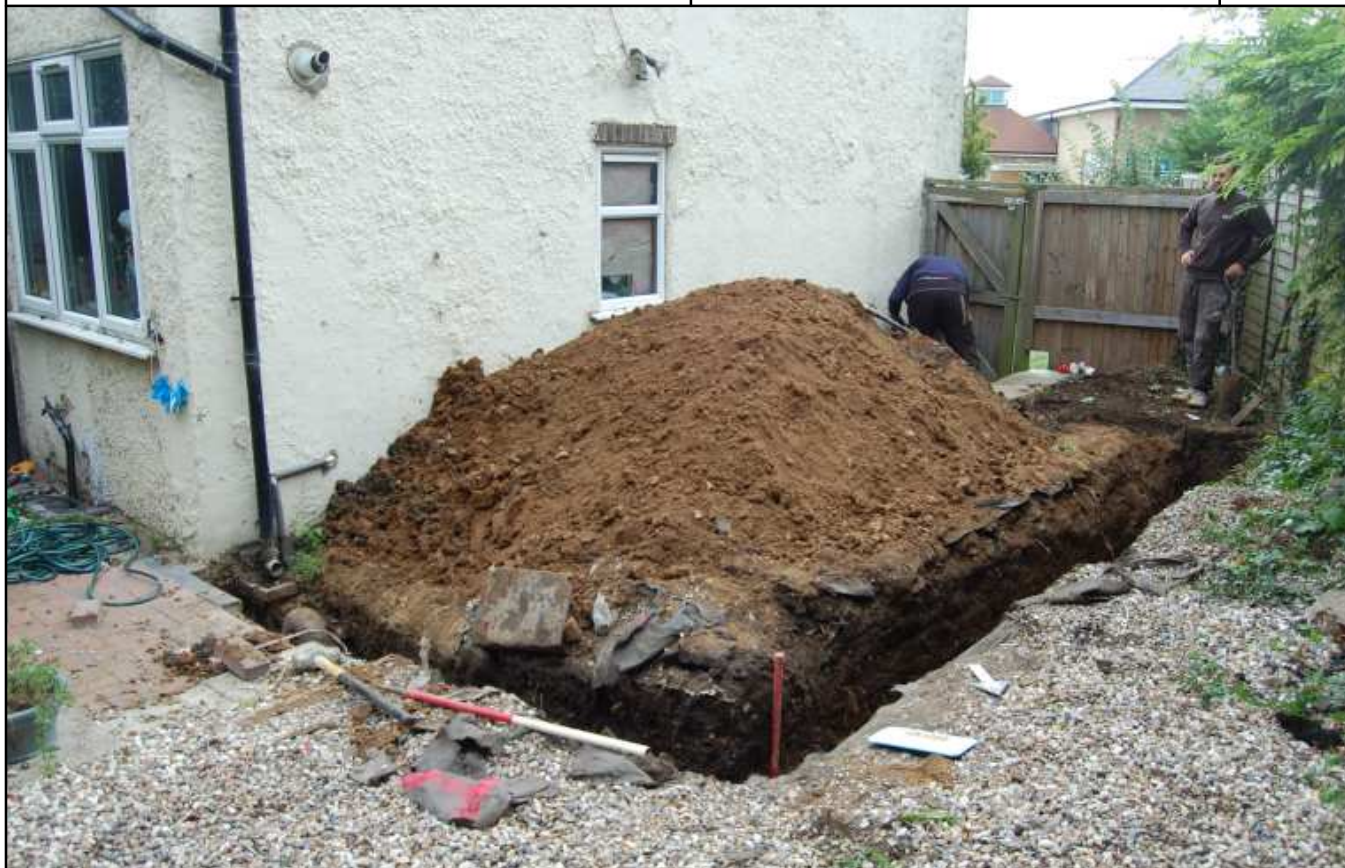
Plate 1: Extension footprint, looking S
