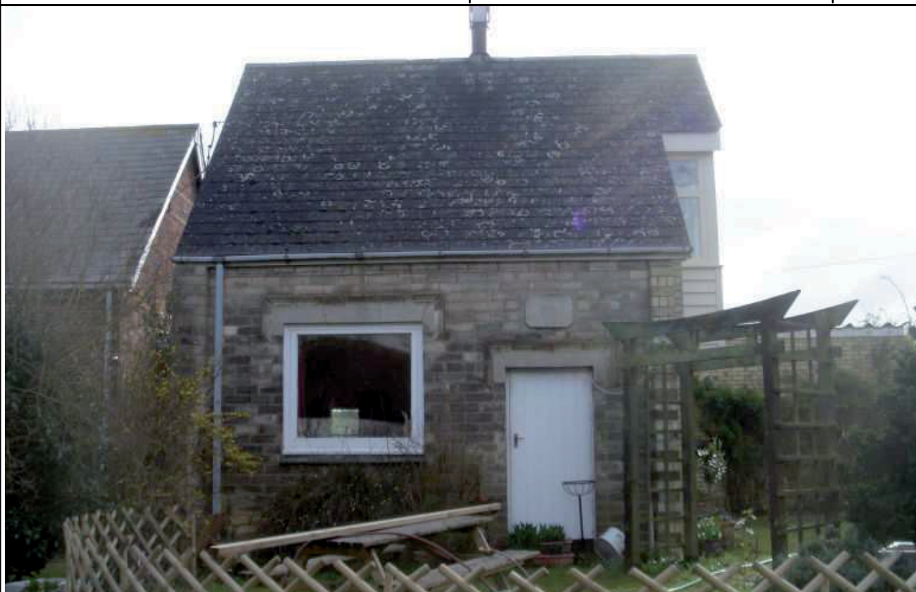
Plate 7: 1852 classroom, western elevation
