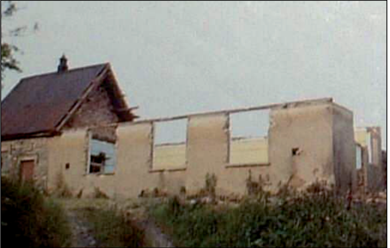
Plate 3: Schoolroom under demolition, looking north-east (client archive)
