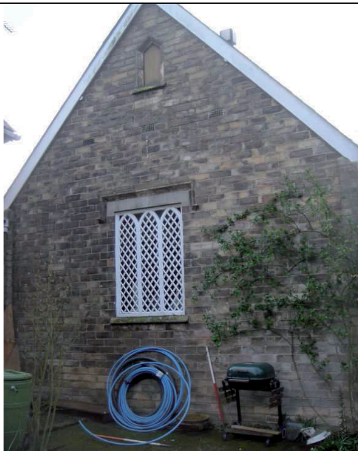
Plate 8: 1852 classroom, northern elevation
