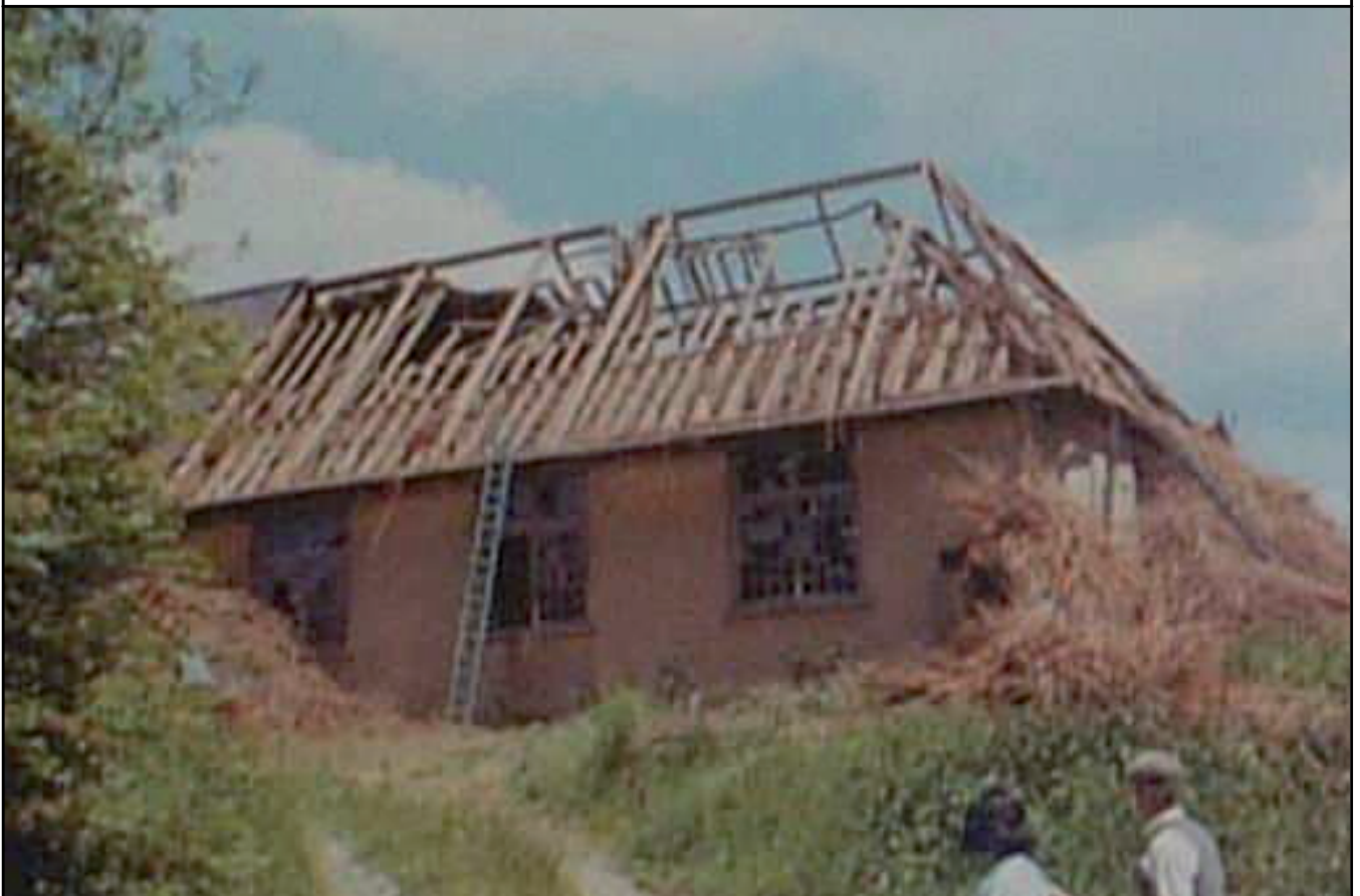
Plate 2: Schoolroom under demolition, looking north-east (client archive)
