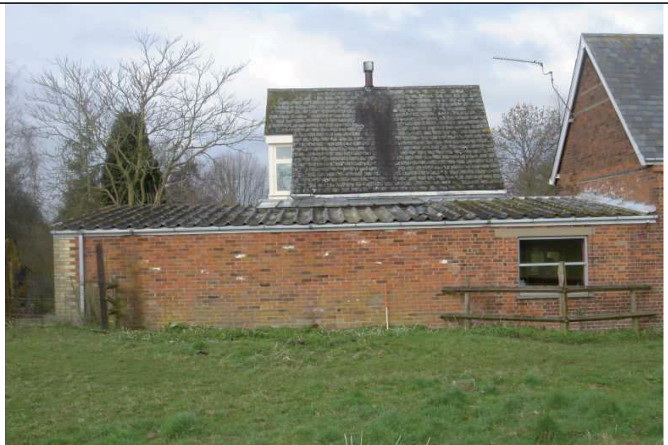
Plate 6: Garage block, looking west
