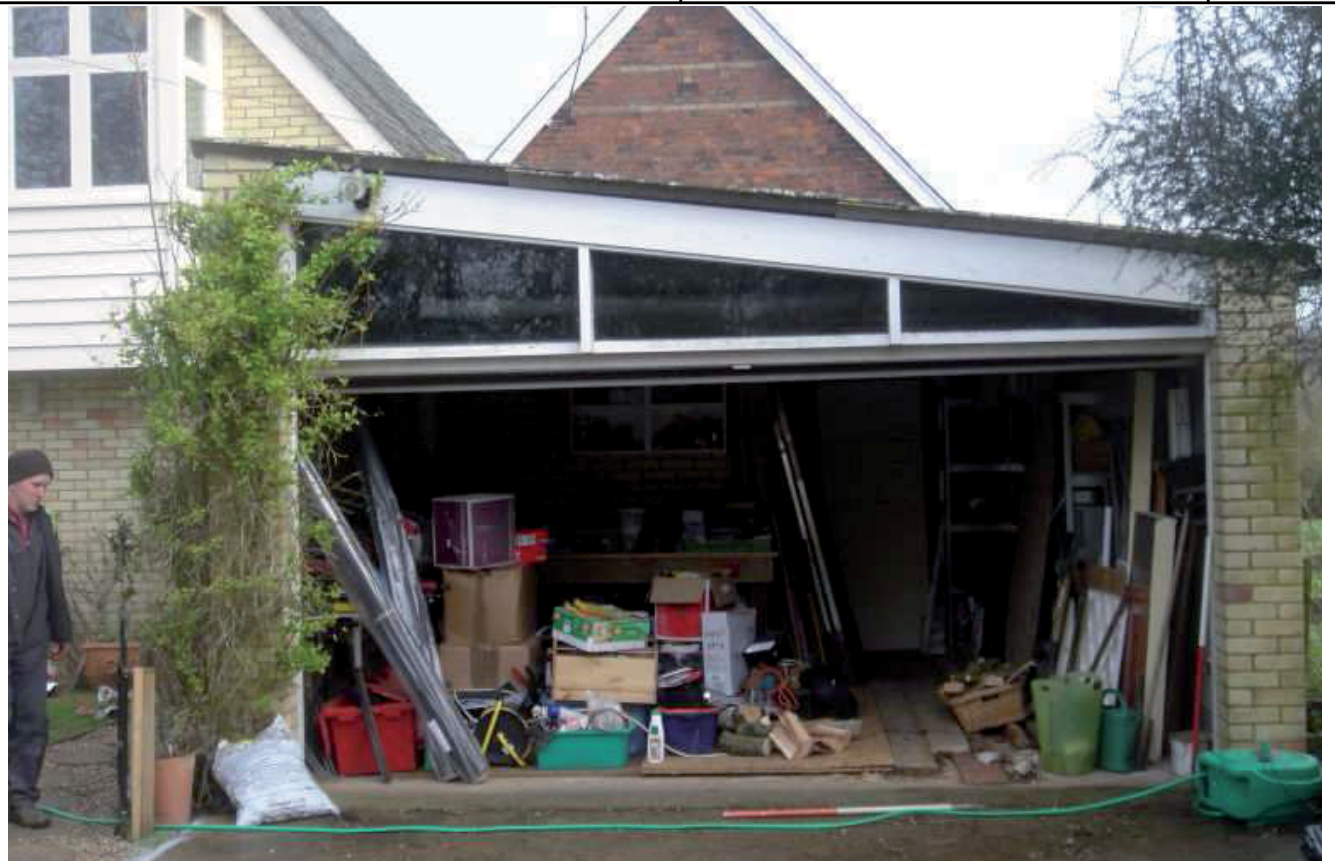
Plate 5: Garage block, looking north
