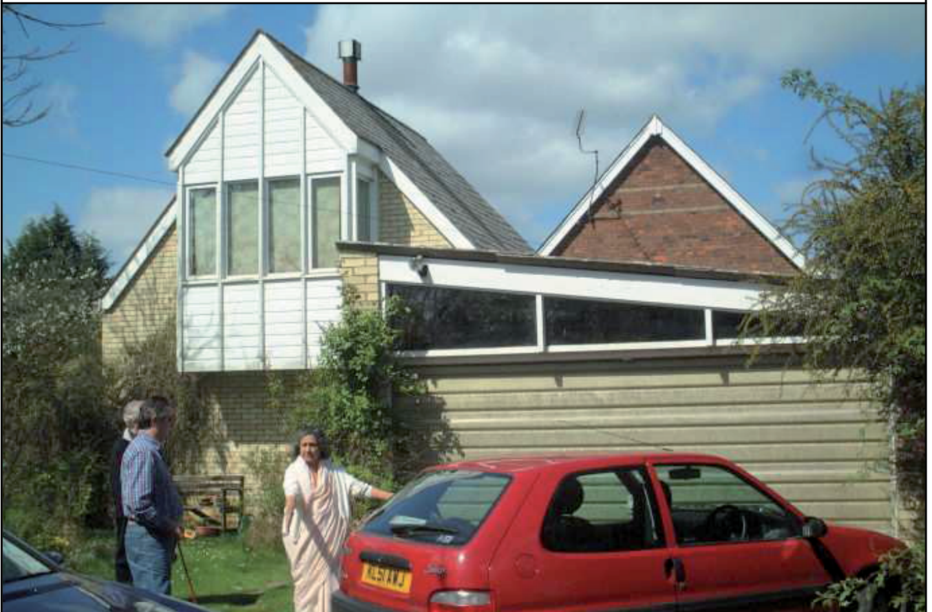
Plate 10: View of buildings before the start of development works, looking NW (client archive)
