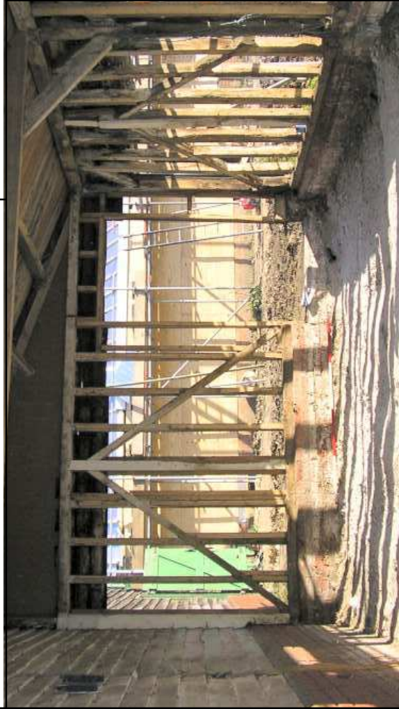
Plate 25: Lean-to, interior facing east
