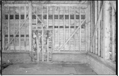
Frame 3: Barn 1, Bay 1, S elevation
