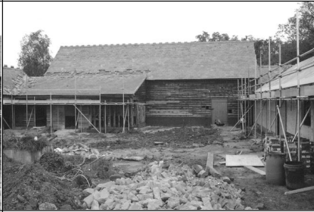
Frame 5: Barn 1 & lean-to, S exterior
