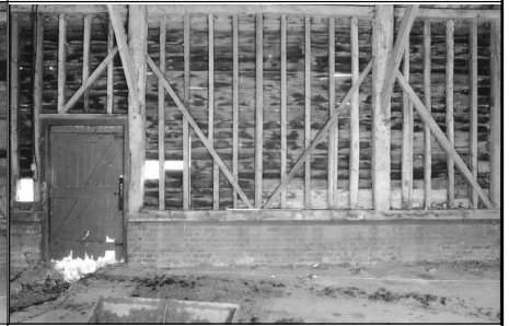
Frame 6: Barn 1, Bay 4, S elevation
