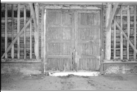
Frame 13: Barn 1, Bay 3, N elevation
