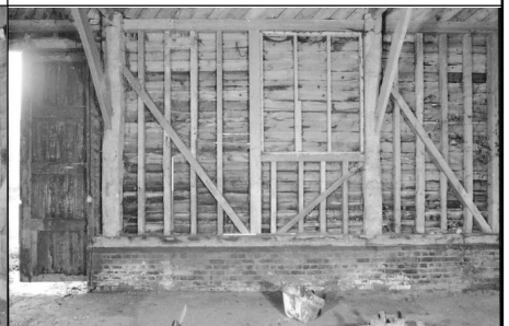
Frame 12: Barn 1, Bay 4, N elevation
