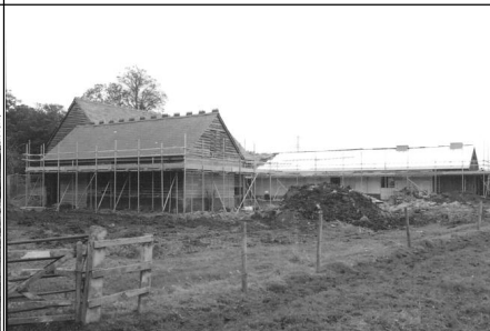
Frame 8: Barns 2 & 3, facing NE
