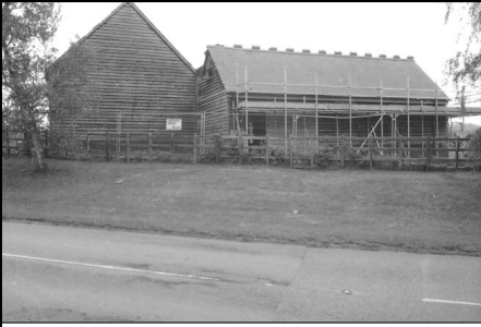
Frame 1: Barns 1 & 2, W exterior
