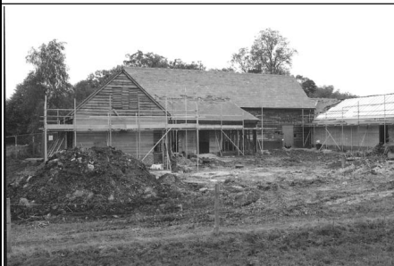
Frame 7: Barns 1 & 2, S exterior
