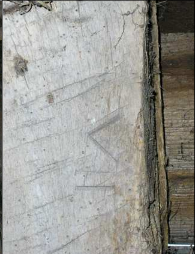
Plate 31: Barn 1, carpenter's mark (detail)
