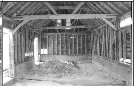
Frame 12: Barn 2, S elevation
