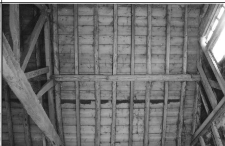
Frame 14: Barn 2, Bay 1, W roof
