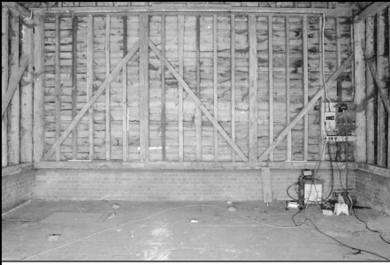
Frame 1: Barn 1, W elevation (bottom)
