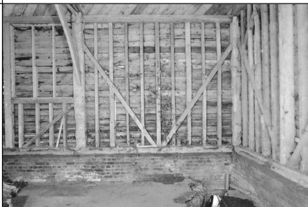
Frame 11: Barn 1, Bay 5, N elevation
