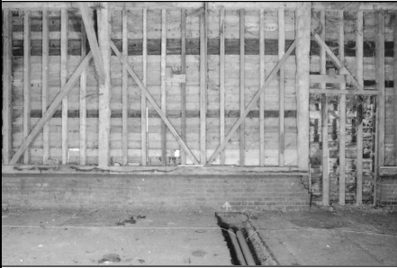
Frame 4: Barn 1, Bay 2, S elevation
