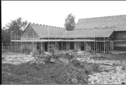
Frame 4: Barns 1, 2 & lean-to, facing NW
