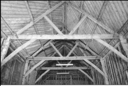
Frame 1: Barn 1, roof structure, facing E
