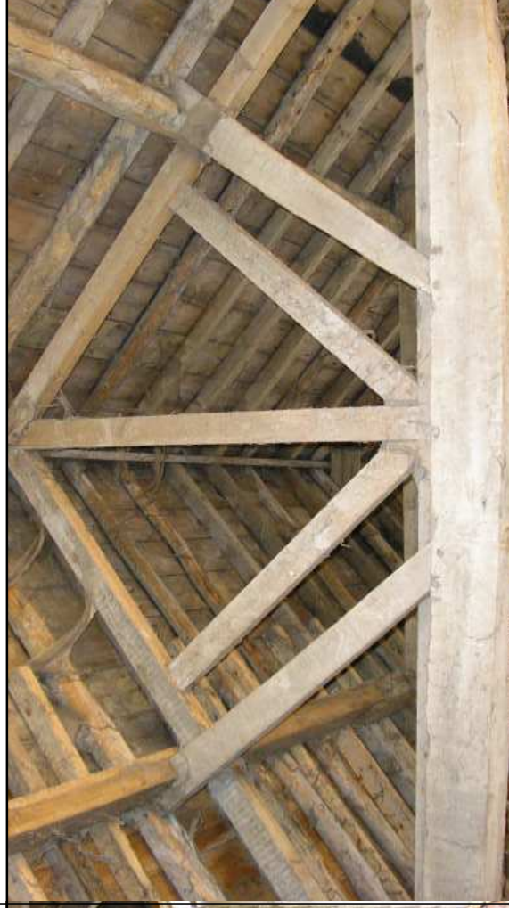
Plate 12: Barn 2, roof truss (detail)
