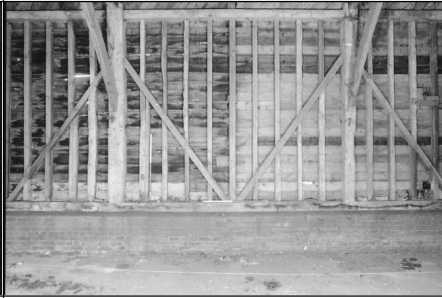
Frame 5: Barn 1, Bay 3, S elevation
