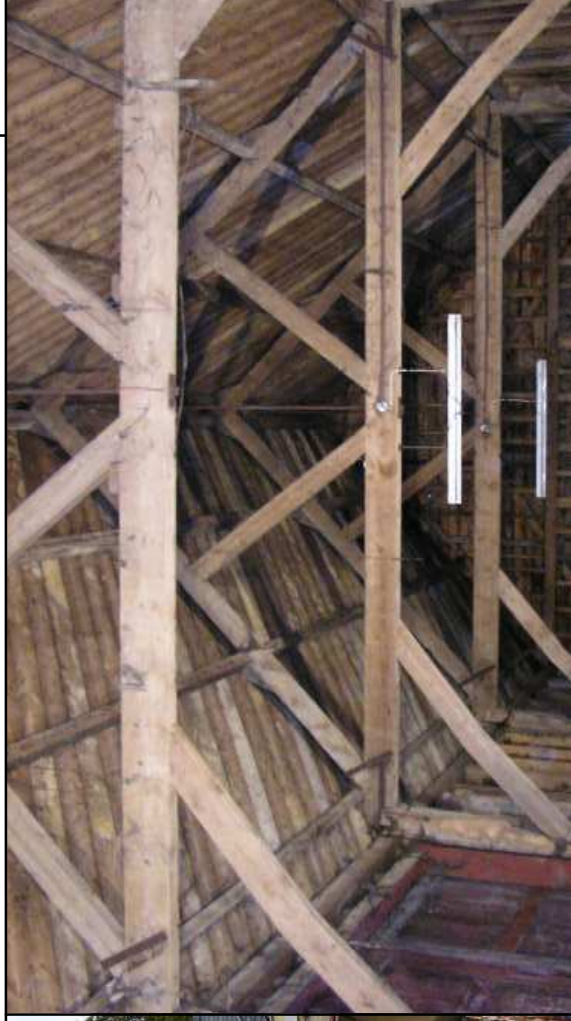
Plate 6: Barn 1 roof structure
