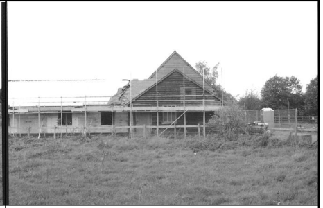
Frame 3: Barn 1 & Garage, E exterior
