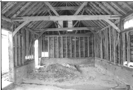
Frame 11: Barn 2, S elevation
