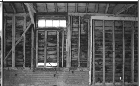
Frame 15: Barn 2, Bay 2, W elevation
