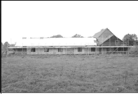
Frame 2: Barns 1 & 3, E exterior
