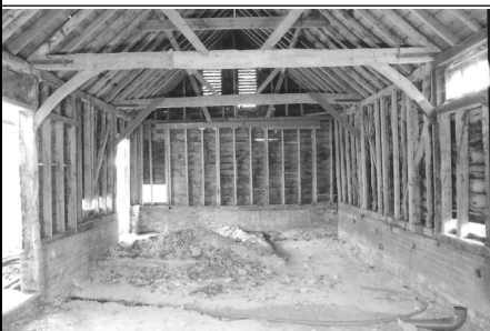
Frame 10: Barn 2, S elevation
