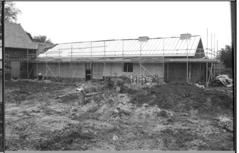
Frame 6: Barn 3, W exterior
