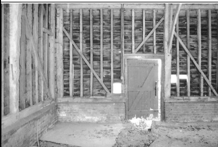
Frame 7: Barn 1, Bay 5, S elevation
