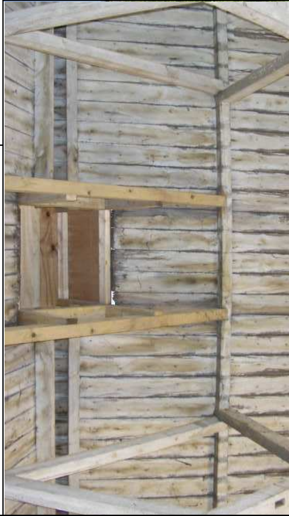
Plate 21: Barn 3, roof of bay 6 (detail)
