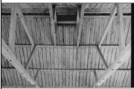
Frame 13: Barn 3, Bay 6, E roof
