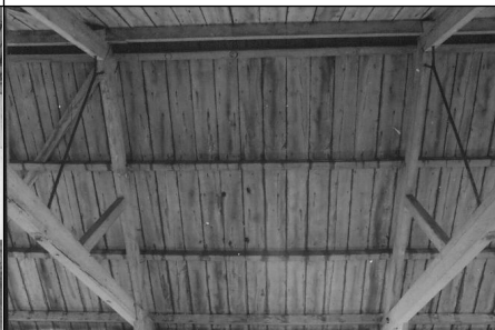
Frame 5: Barn 2, Bay 1, E roof
