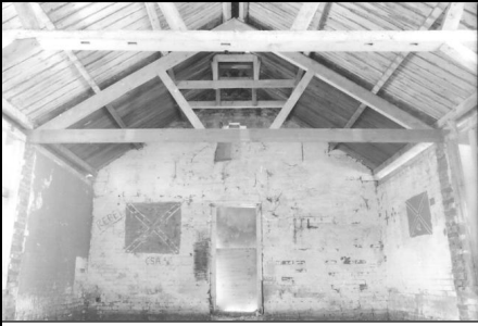
Frame 1: Barn 3, Bay 8, S elevation
