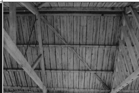
Frame 9: Barn 3, Bay 4, E roof
