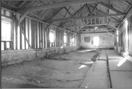
Frame 5: Barn 3, interior, facing S
