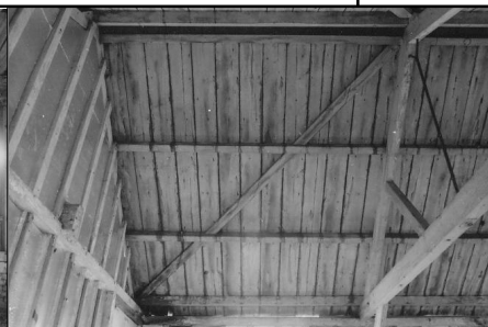
Frame 3: Barn 3, Bay 1, E roof
