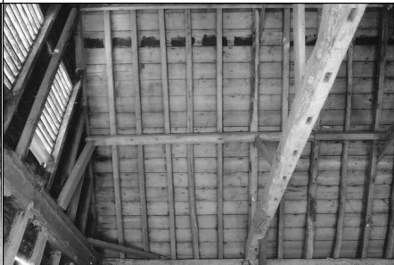
Frame 5: Barn 2, Bay 4, W roof
