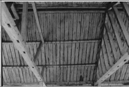
Frame 8: Barn 3, Bay 5, W roof
