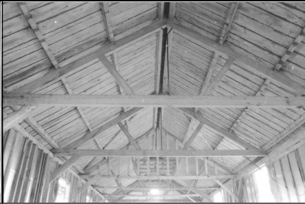
Frame 2: Barn 3, roof structure, facing S
