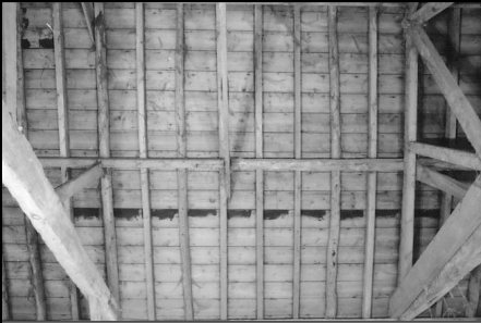
Frame 1: Barn 2, Bay 2, W roof
