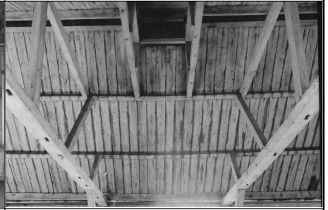
Frame 6: Barn 3, Bay 6, W roof
