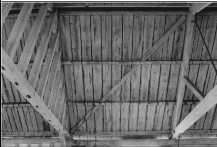
Frame 10: Barn 3, Bay 4, W roof
