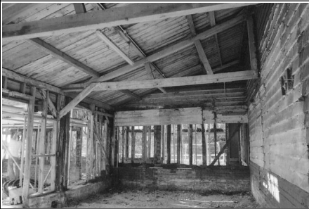
Frame 7: Lean-to, interior, facing W
