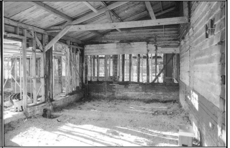
Frame 6: Lean-to, W elevation
