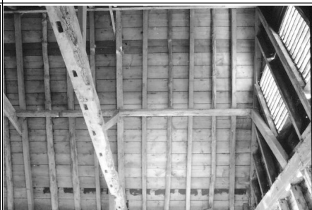
Frame 8: Barn 2, Bay 4, E roof
