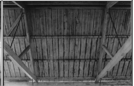
Frame 12: Barn 3, Bay 3, W roof
