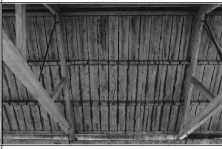
Frame 14: Barn 3, Bay 2, W roof
