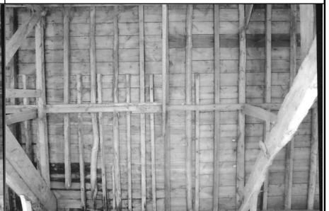
Frame 12: Barn 2, Bay 2, E roof
