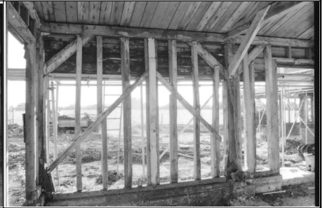
Frame 9: Lean-to, Bay 3, S elevation
