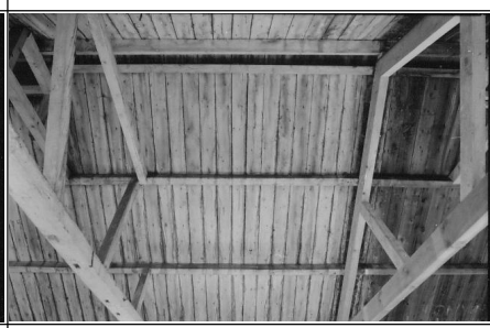
Frame 15: Barn 3, Bay 7, E roof
