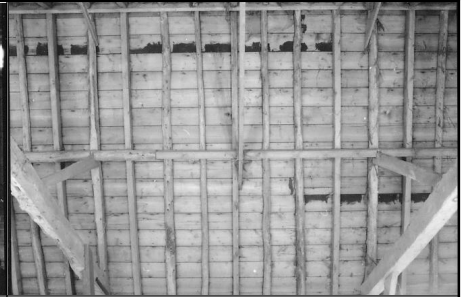
Frame 3: Barn 2, Bay 3, W roof
