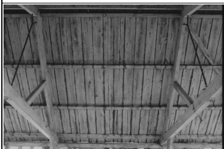
Frame 7: Barn 3, Bay 3, E roof
