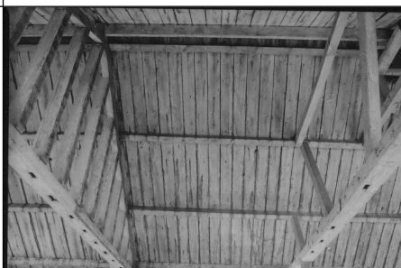
Frame 11: Barn 3, Bay 5, E roof
