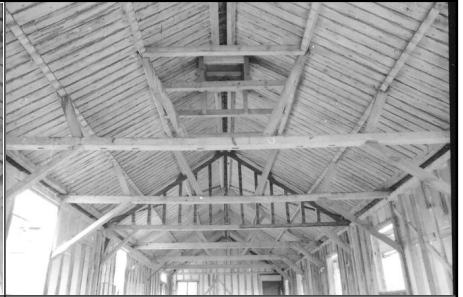
Frame 3: Barn 3, roof structure, facing N
