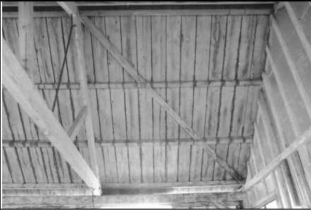
Frame 1: Barn 3, Bay 1, W roof
