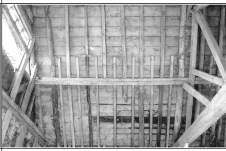
Frame 14: Barn 2, Bay 1, E roof
