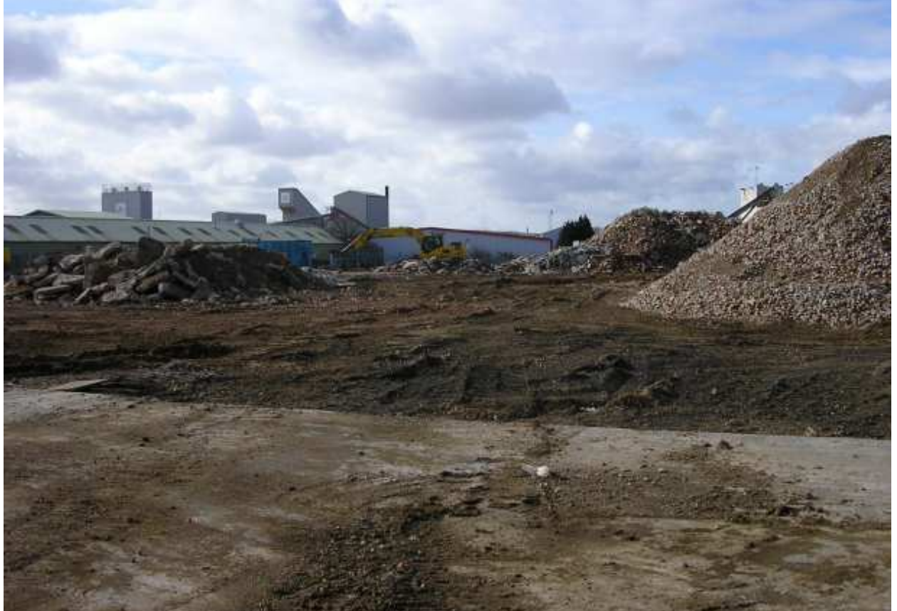
Plate 1: Area of tarmac removal
