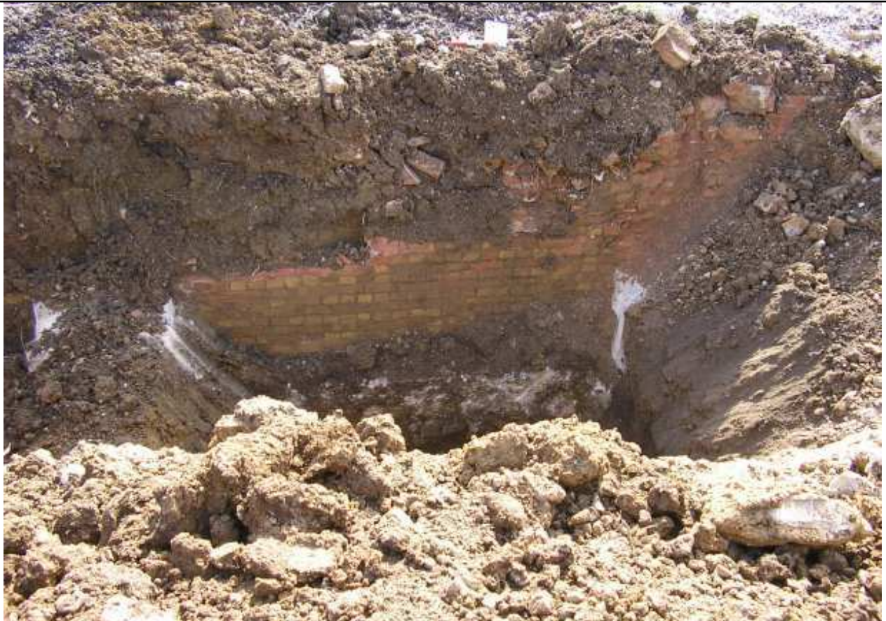
Plate 2: South wall, former M/A-Com building, under demolition
