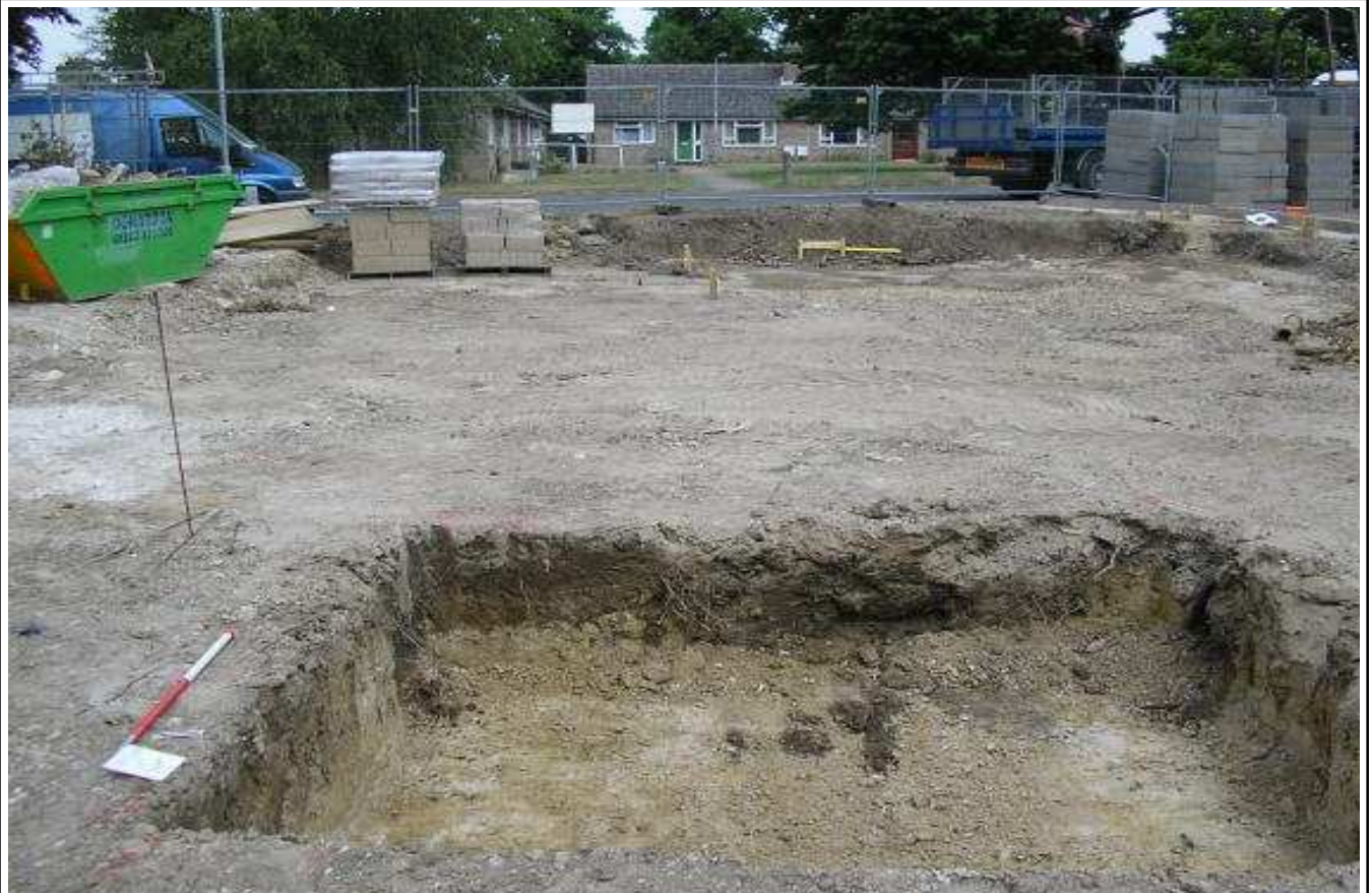
Plate 2: Lift shaft, large bedroom block, looking west
