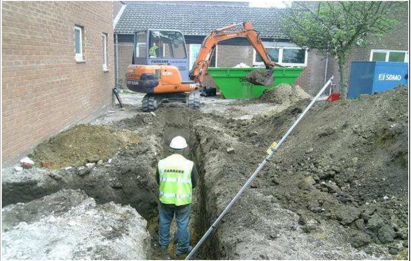
Plate 1: Footings trench, small bedroom block, looking east
