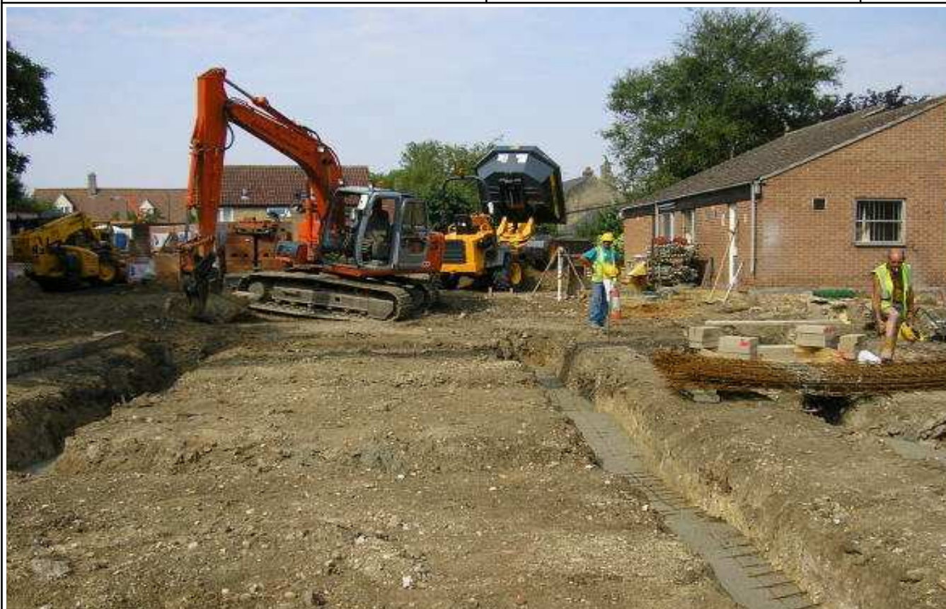
Plate 3: Footings trenches, large bedroom block, looking east
