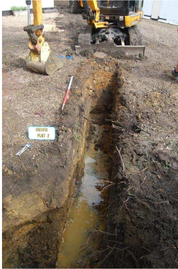
Plate 11 - Plot 2 (drainage trench), looking N
