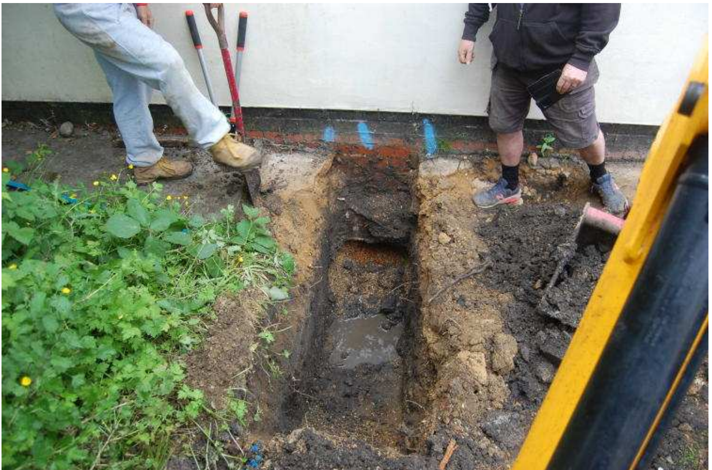
Plate 10 - Excavated footings trench, looking SE
