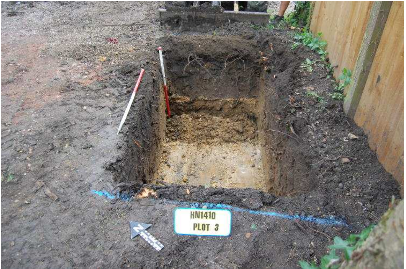
Plate 13 - Plot 3 (septic tank), looking NE
