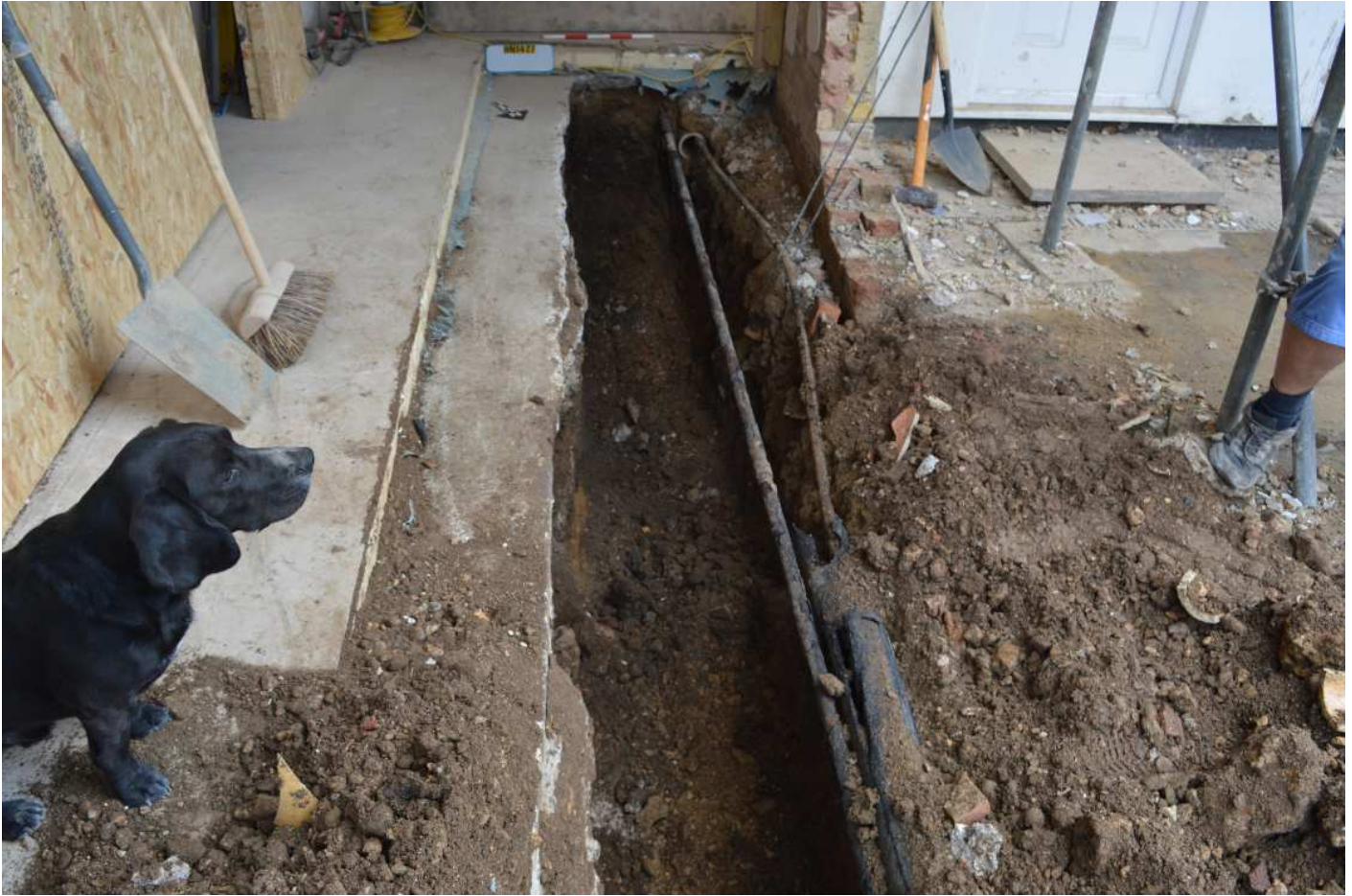
Plate 01 - Service trench, looking S
