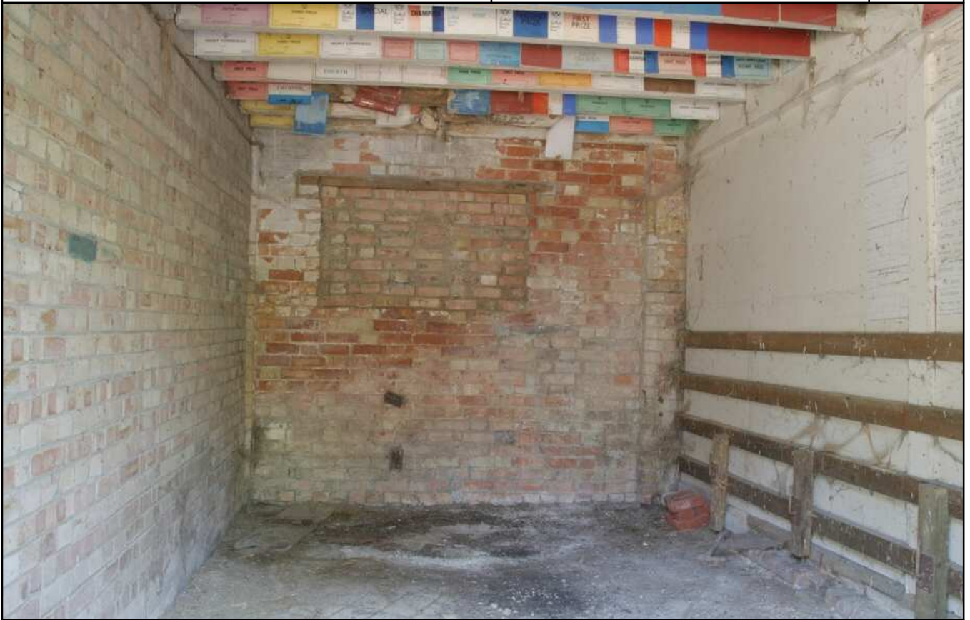
Plate 15 - Bay 4, eastern interior elevation, facing E
