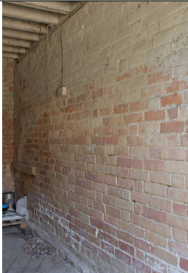
Plate 08 - Bay 1, southern interior elevation, facing SE
