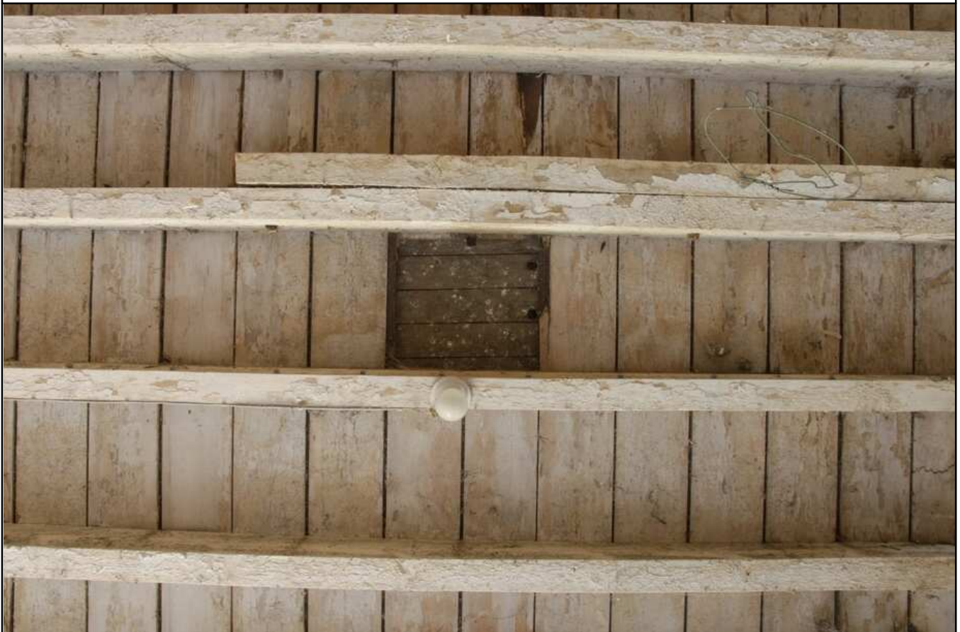
Plate 10 - Bay 1, ceiling structure and trapdoor
