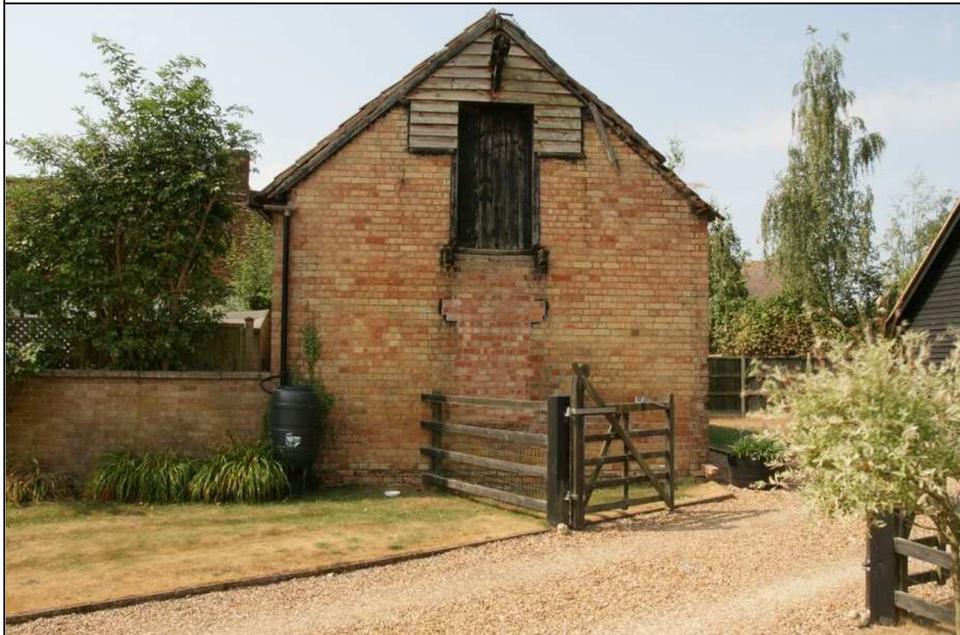
Plate 02 - Northern exterior elevation, facing S
