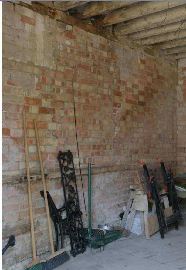
Plate 06 - Bay 1, northern interior elevation, facing NE
