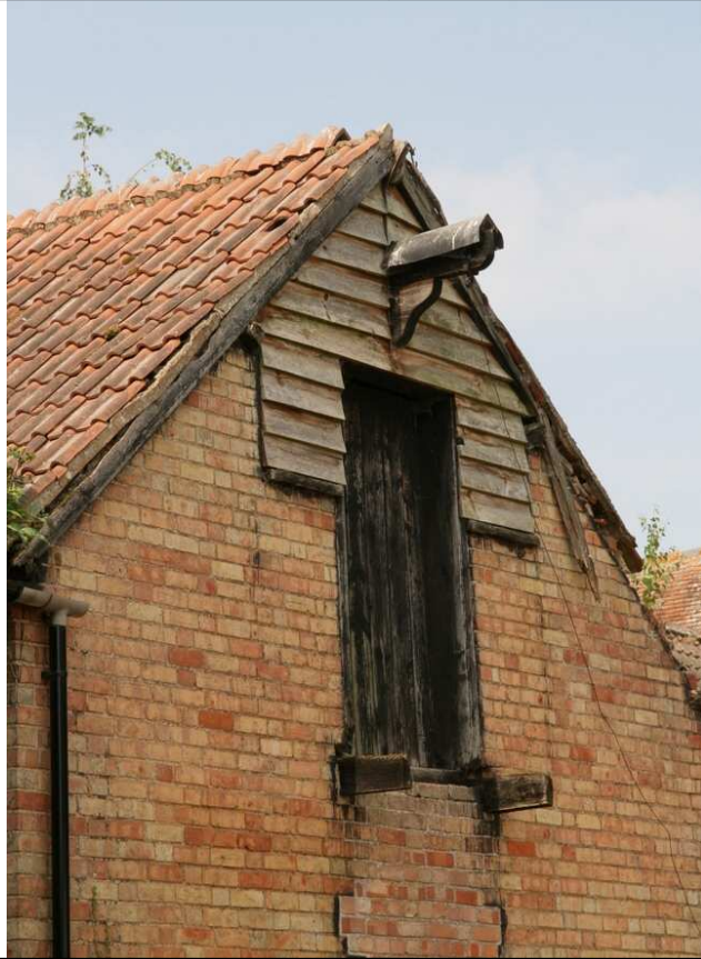
Plate 03 - Loft access and hoist, facing SW
