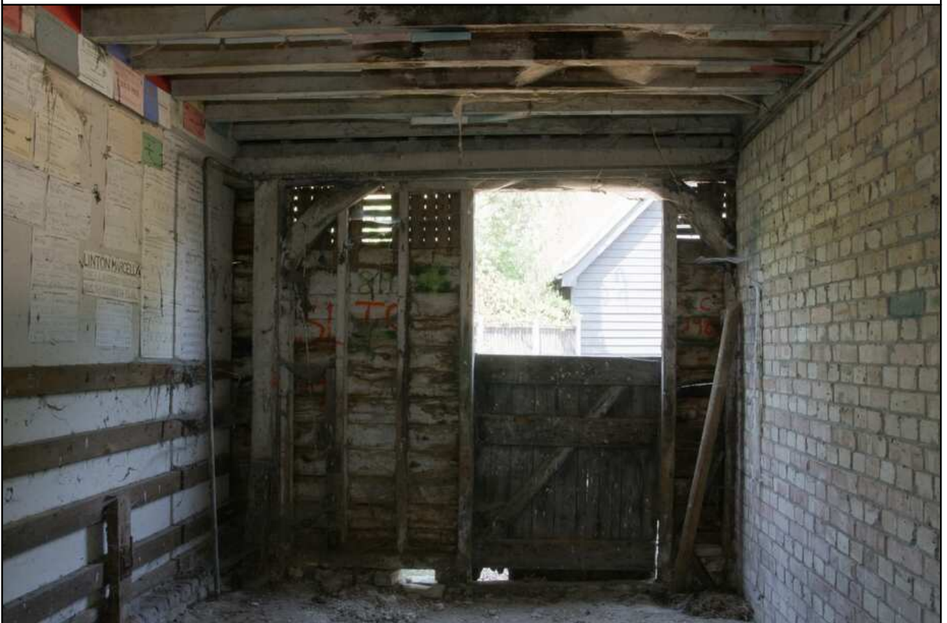
Plate 16 - Bay 4, western interior elevation, facing W
