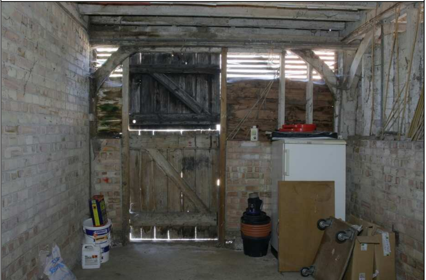
Plate 14 - Bay 3, western interior elevation, facing W
