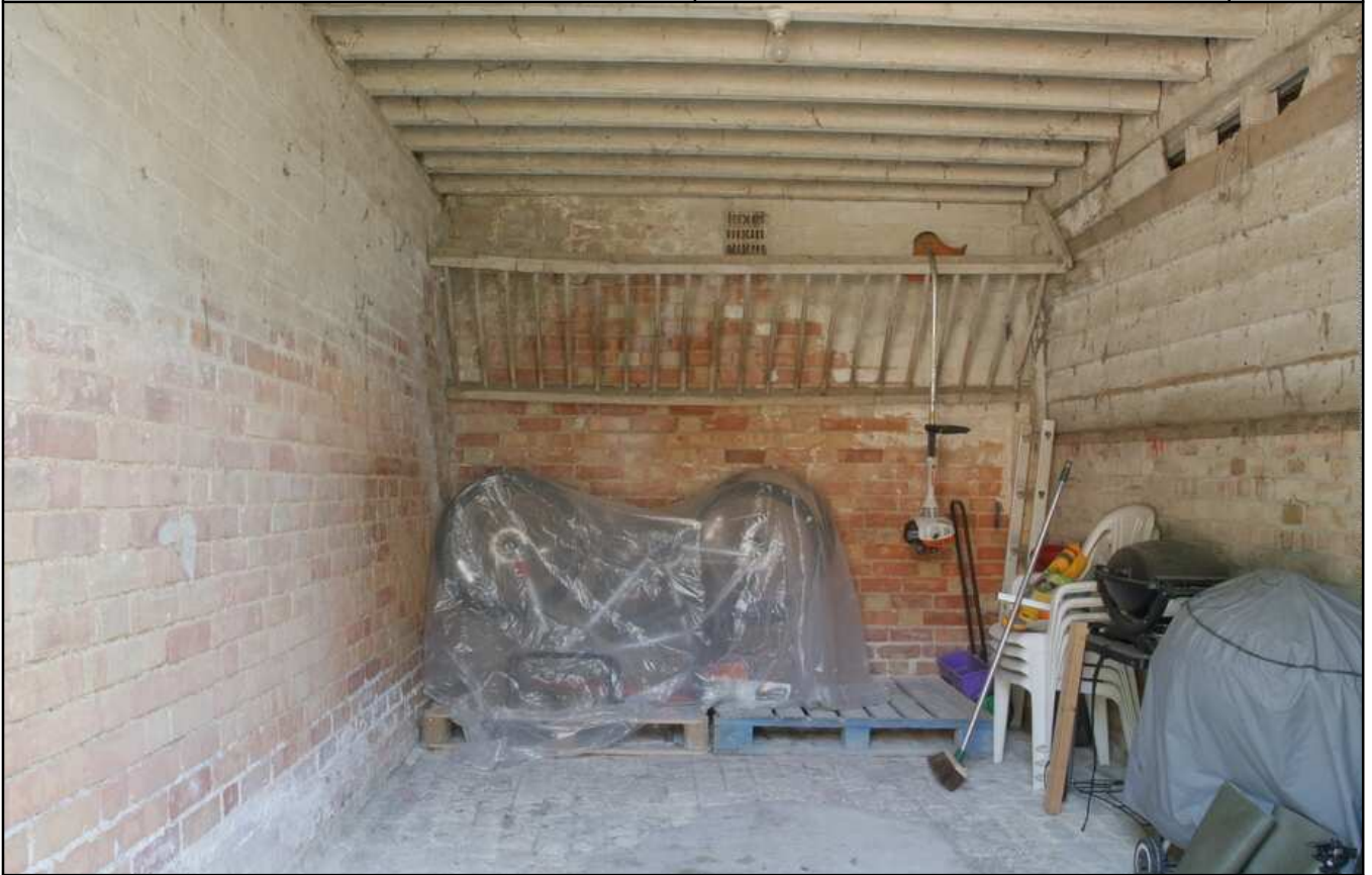
Plate 11 - Bay 2, eastern interior elevation, facing E
