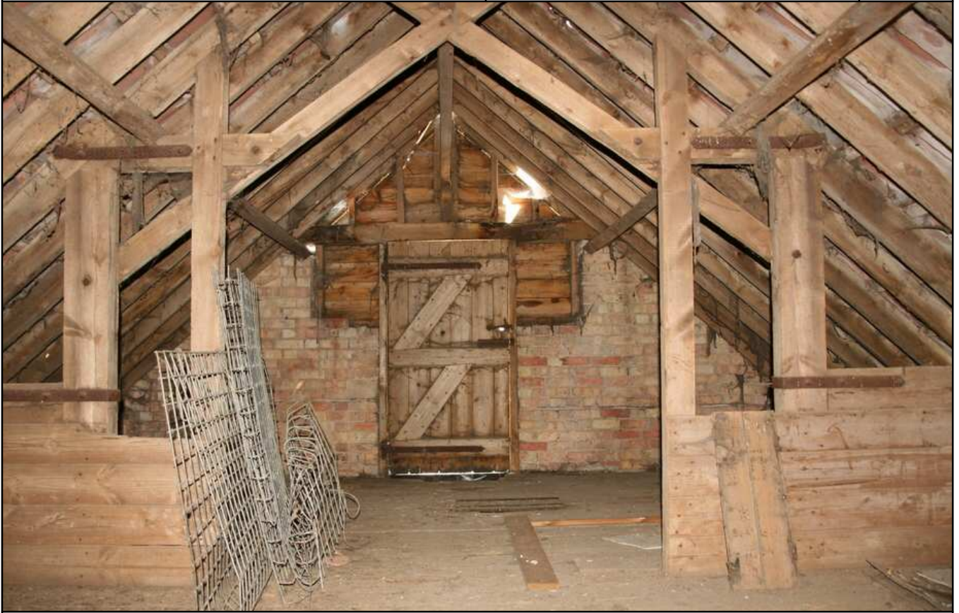
Plate 23 - Loft, roof and hoist structure, facing N
