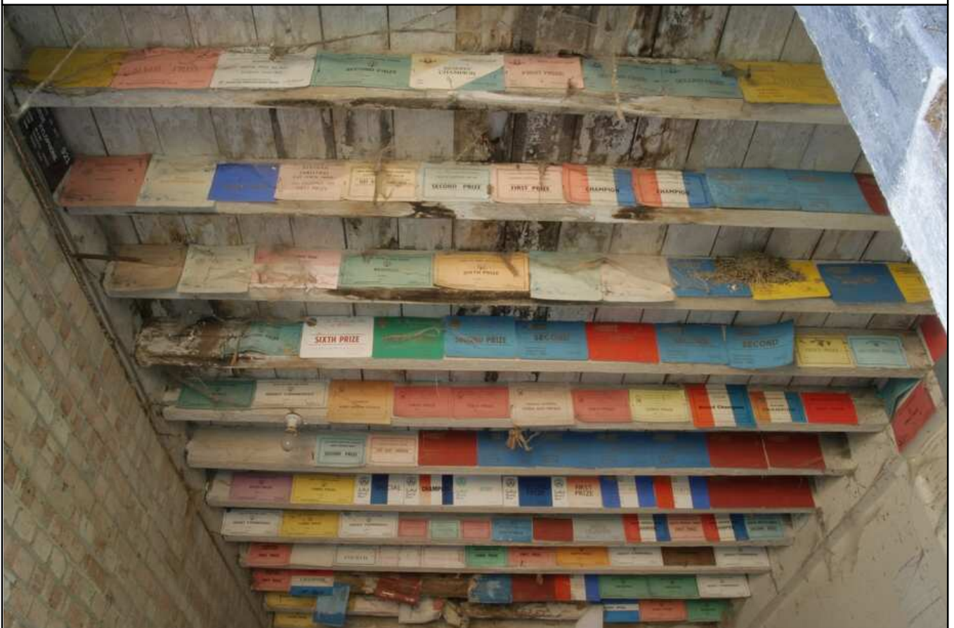
Plate 18 - Bay 4, prize certificates on joists, facing E
