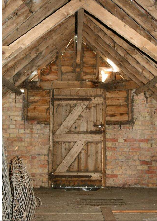
Plate 19 - Loft, northern interior elevation, facing N
