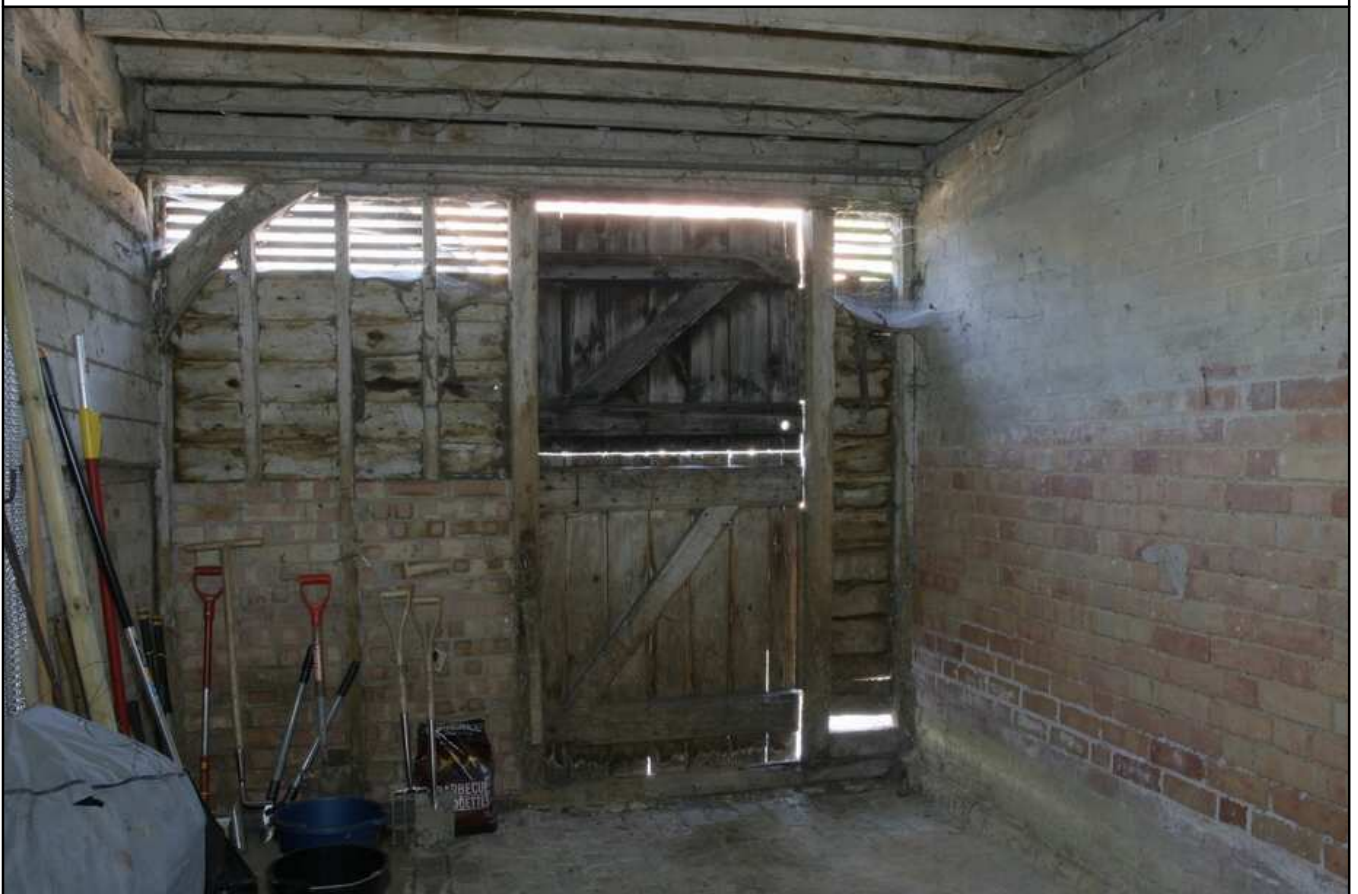
Plate 12 - Bay 2, western interior elevation, facing W
