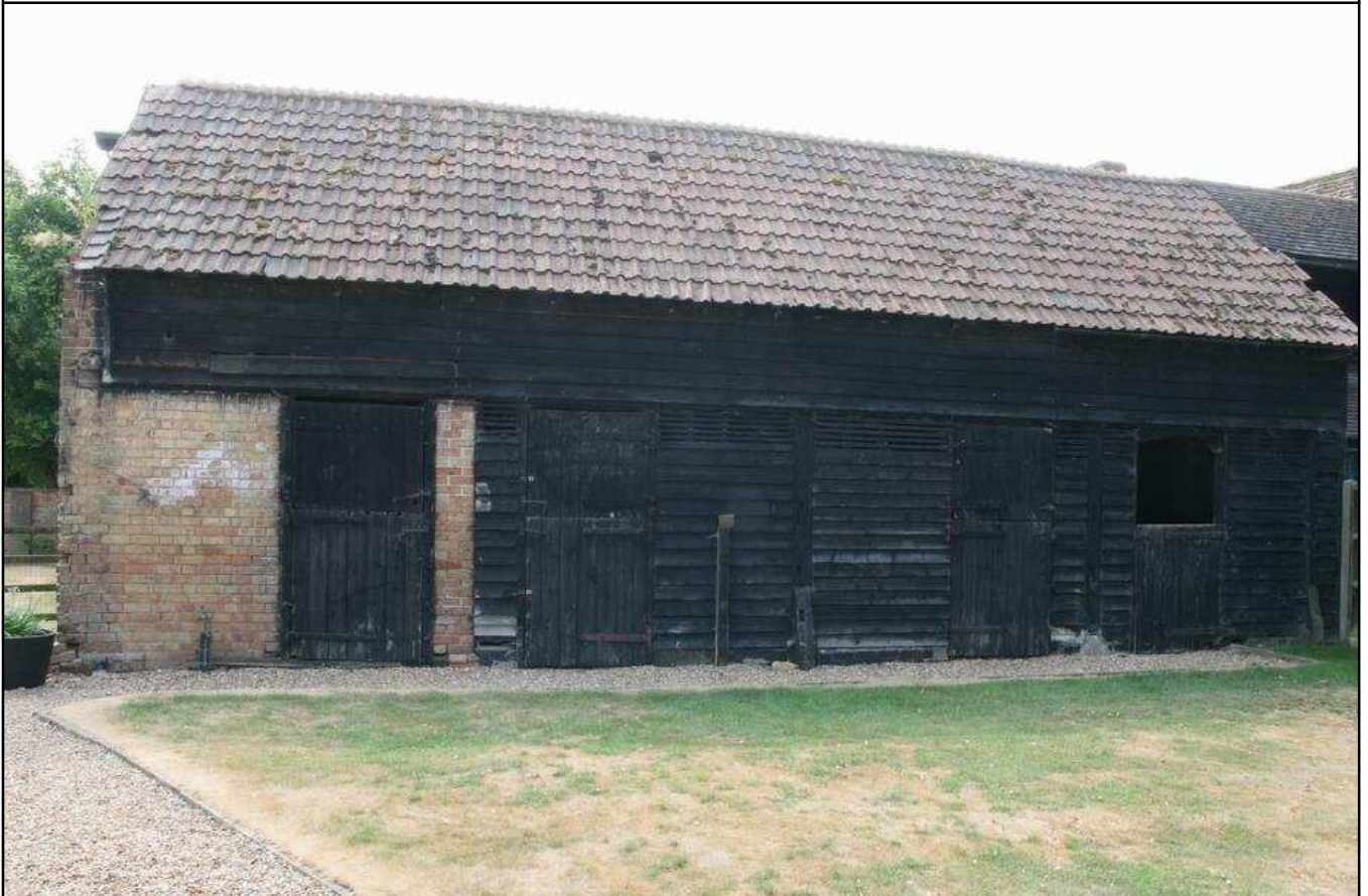
Plate 04 - Western exterior elevation, facing E
