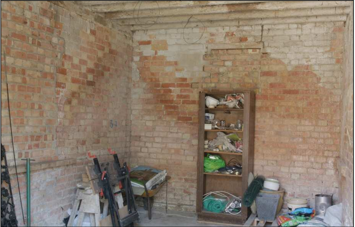
Plate 07 - Bay 1, eastern interior elevation, facing E
