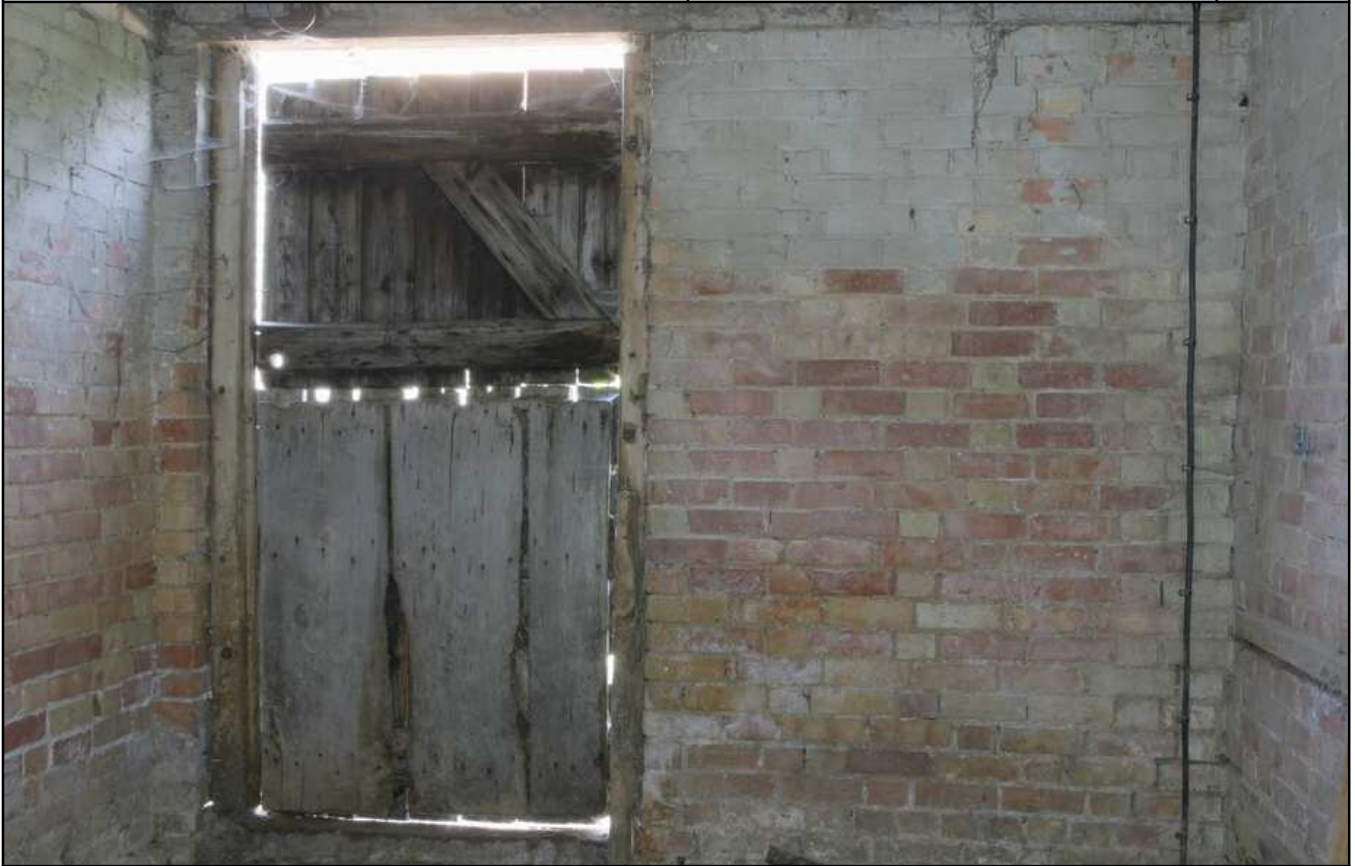
Plate 09 - Bay 1, western interior elevation, facing W
