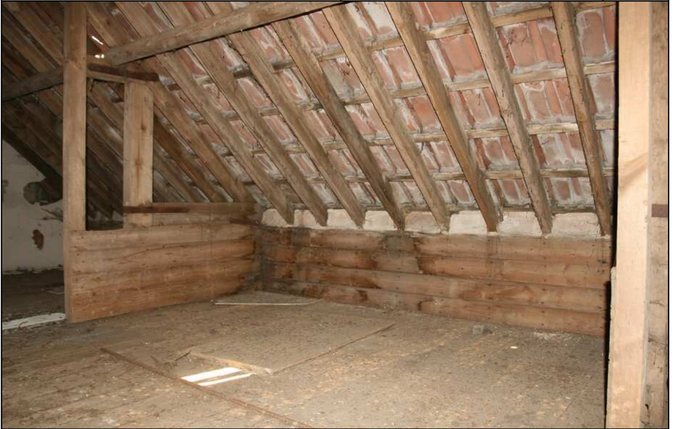
Plate 21 - Loft, western interior elevation, facing SW
