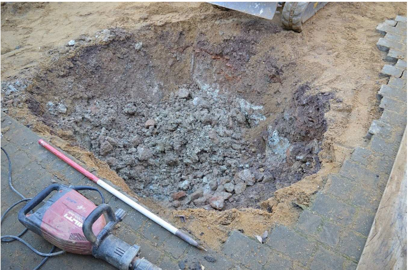
Plate 06 - Soakaway, looking NW
