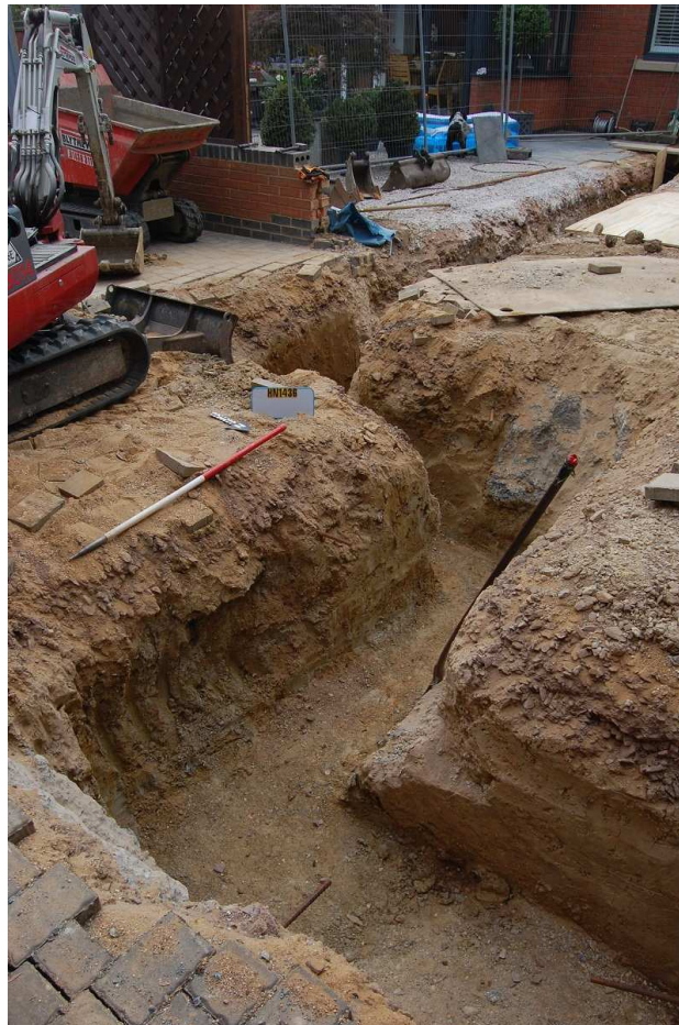
Plate 04 - Junction between Trenches D & E, looking SW
