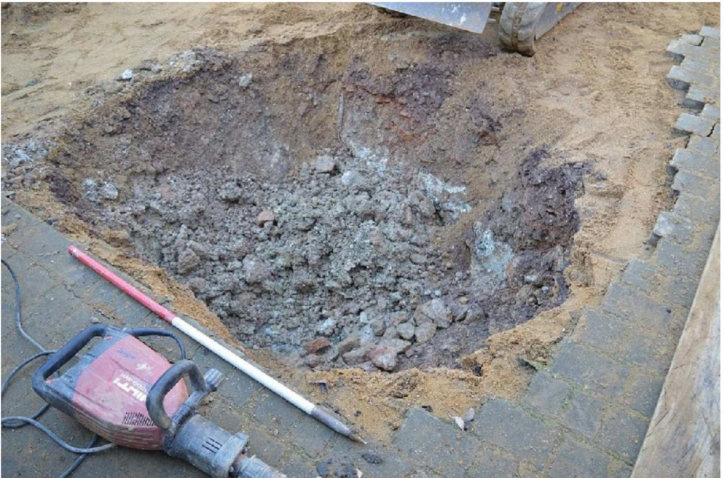
Plate 06 - Soakaway, looking NW
