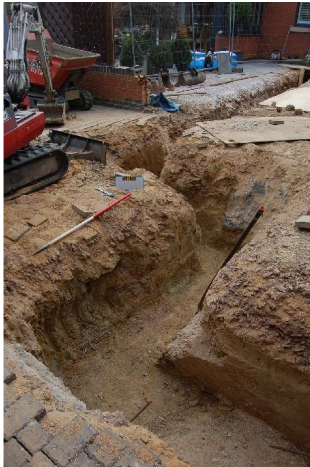
Plate 04 - Junction between Trenches D & E, looking SW
