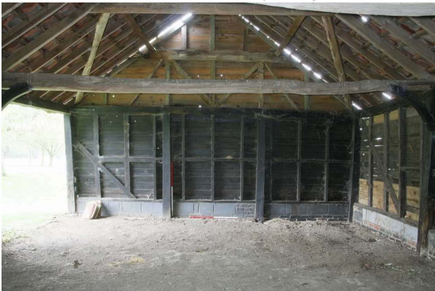
Plate 12 - Northern interior elevation, looking N
