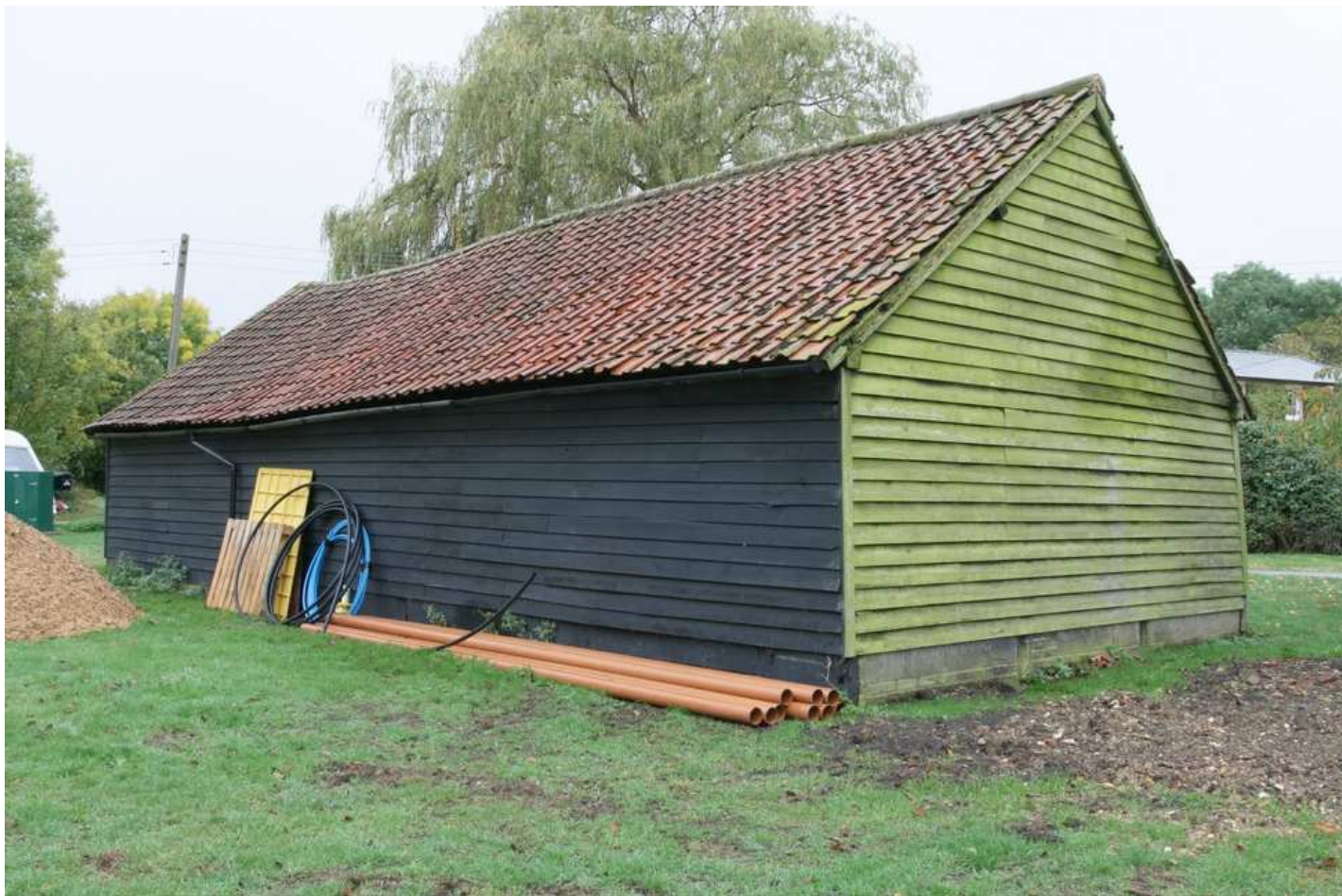
Plate 03 - Eastern exterior elevation, looking SW
