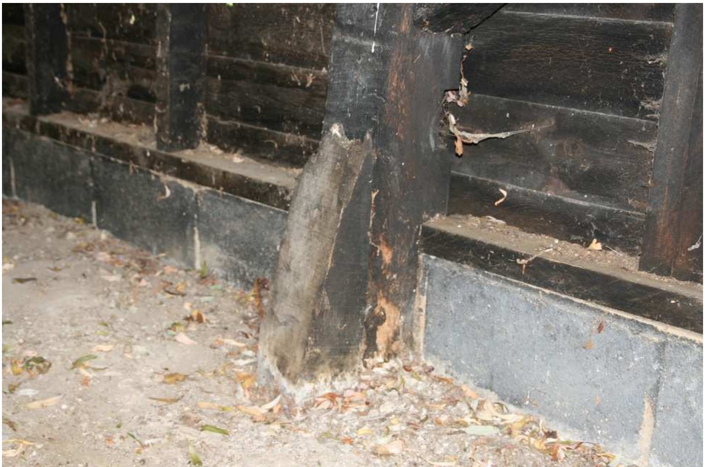
Plate 16 - Protective bumper on post in southern elevation, looking SE
