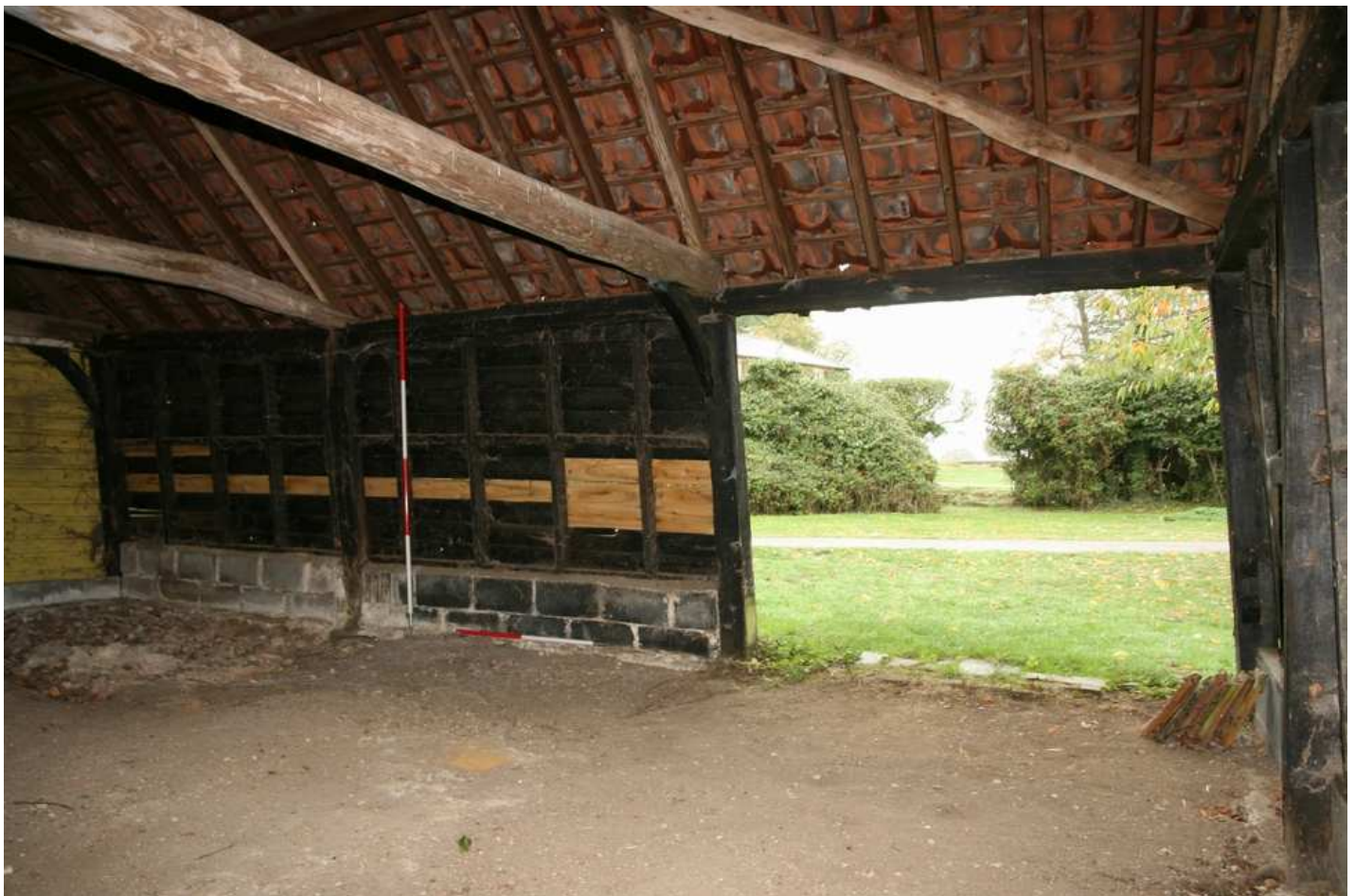
Plate 10 - Western interior elevation, Bays 1-3, looking W
