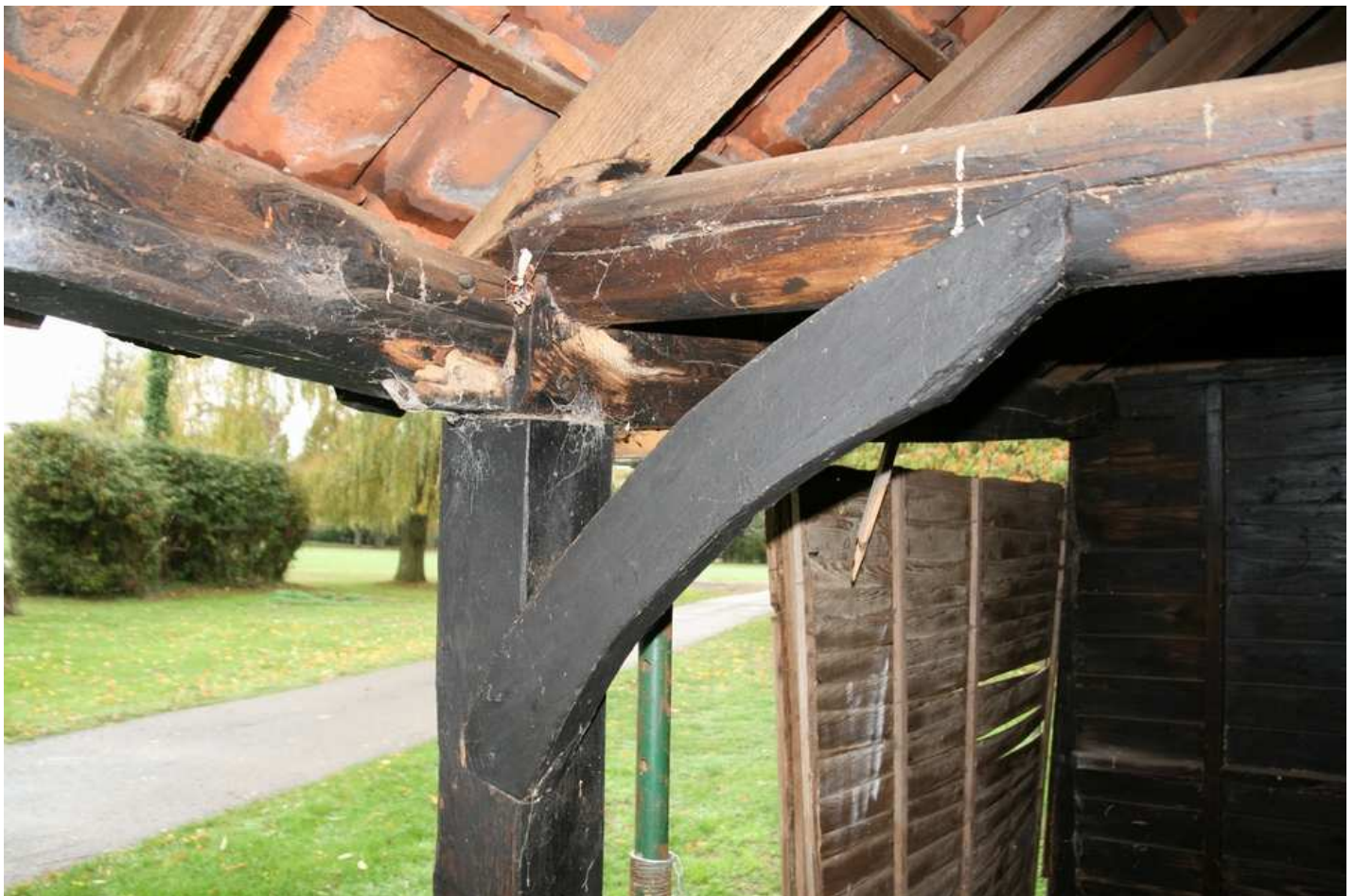
Plate 06 - Bracing to principal post between Bays 4 & 5, looking NW
