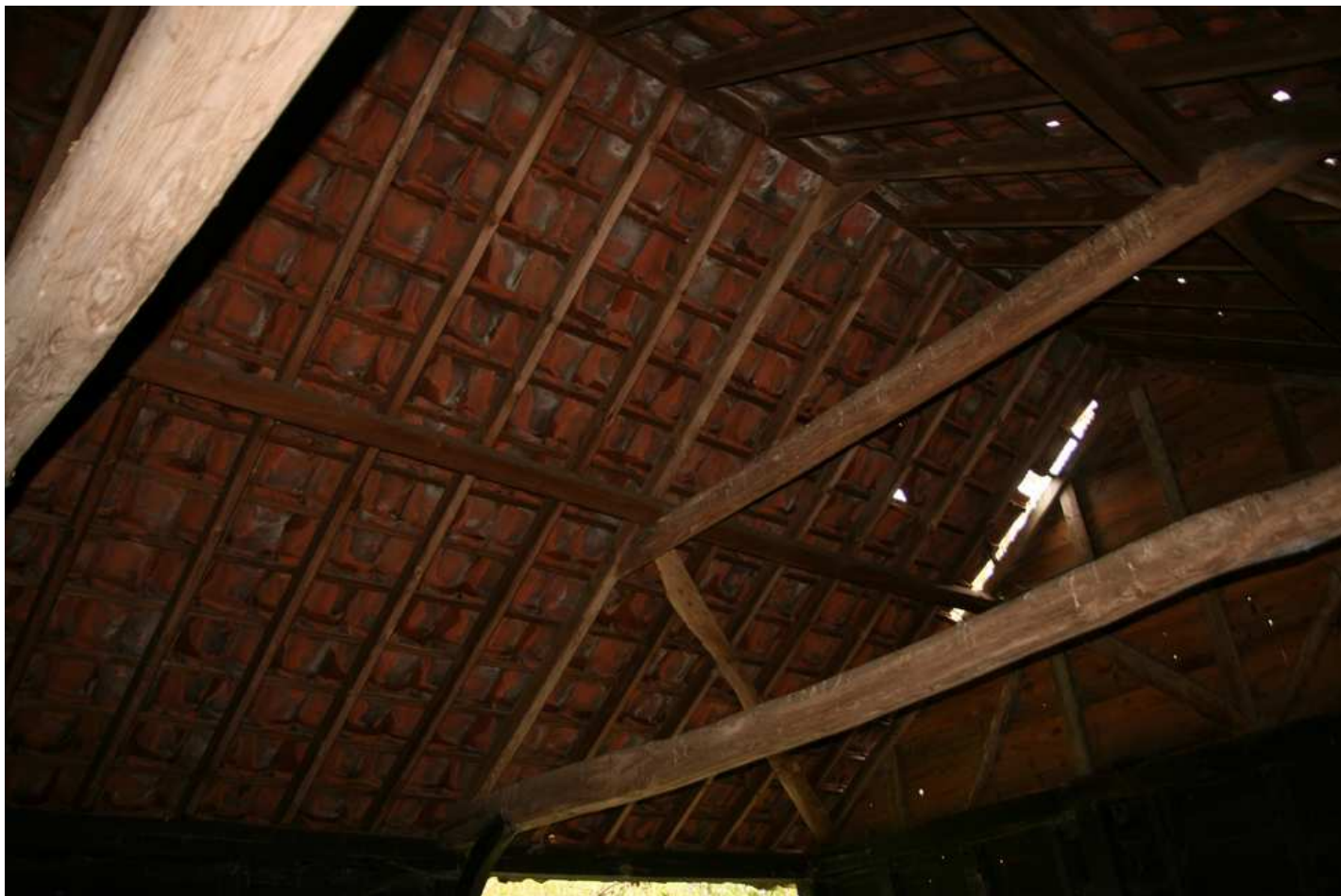
Plate 07 - Roof structure at northern end, looking NW
