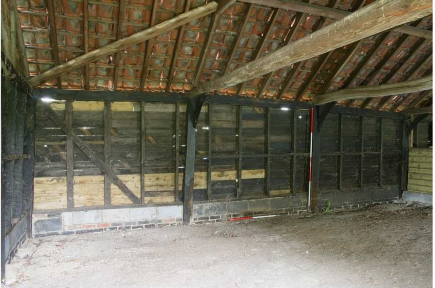
Plate 13 - Eastern interior elevation, Bays 1-3, looking E
