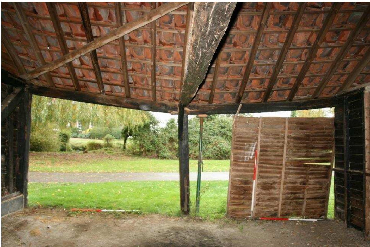
Plate 11 - Western interior elevation, Bays 4-5, looking W
