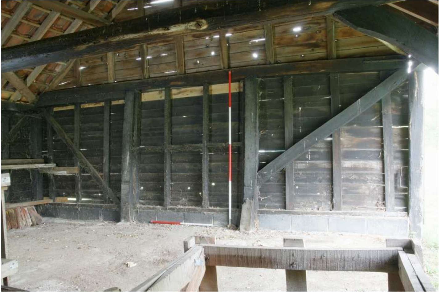
Plate 15 - Southern interior elevation, looking S
