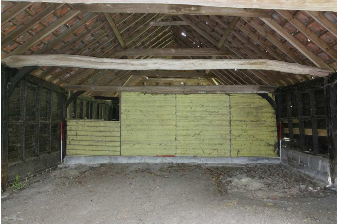
Plate 05 - Partition between Bays 3 & 4, looking S
