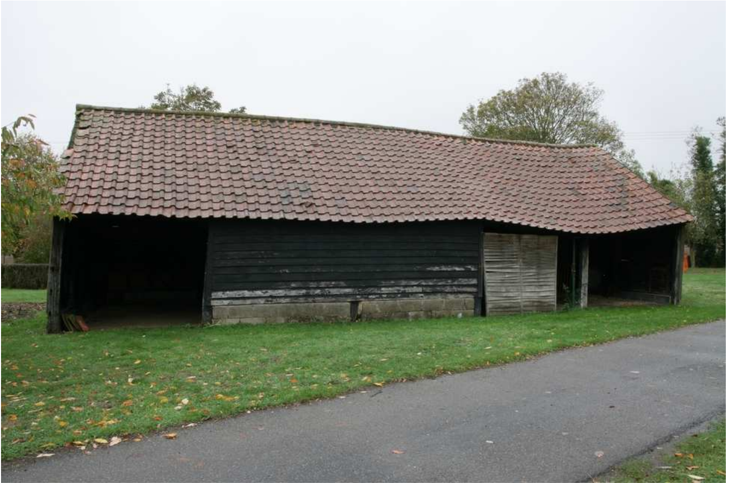
Plate 01 - Western exterior elevation, looking E
