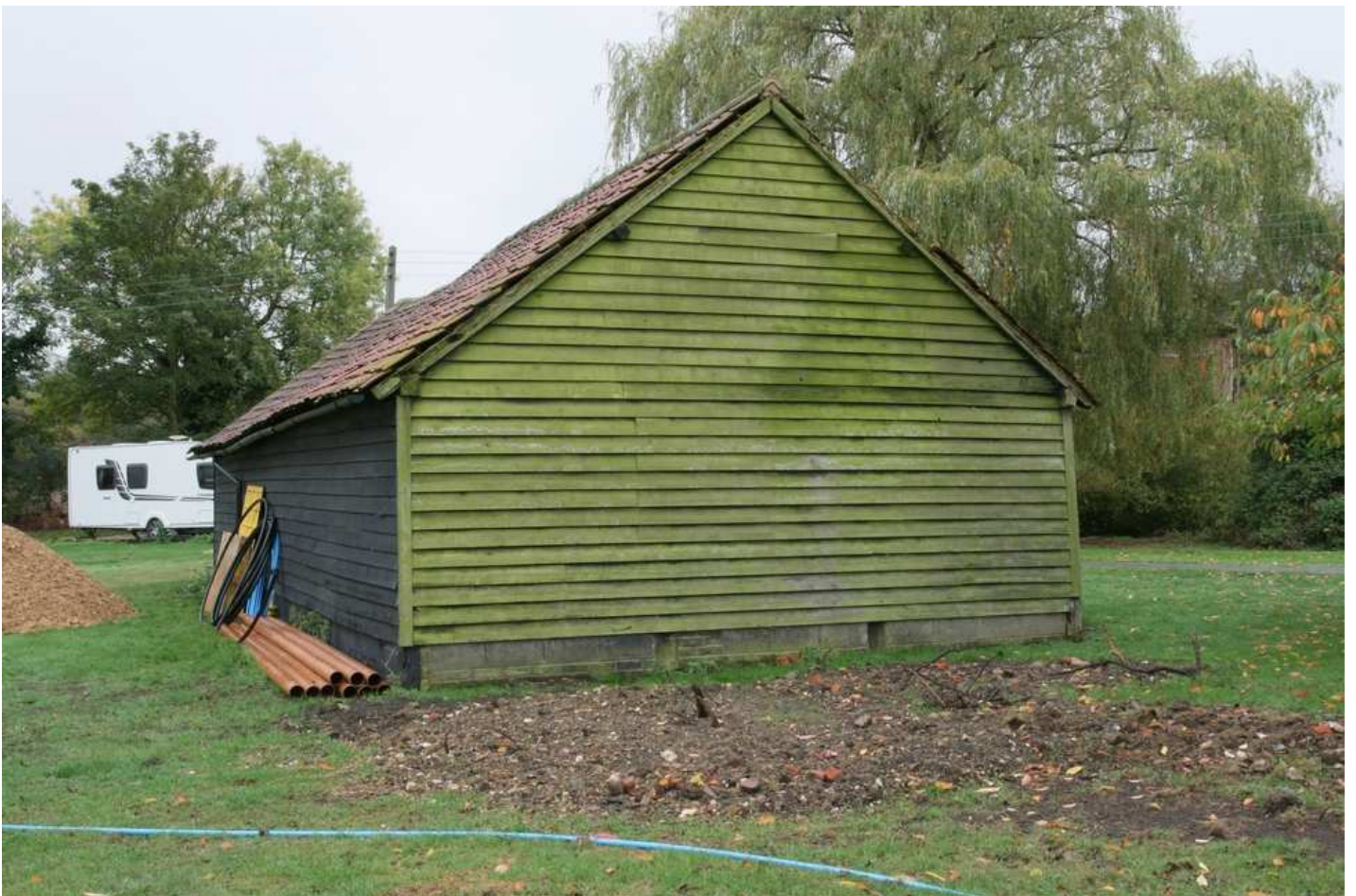
Plate 02 - Northern exterior elevation, looking S
