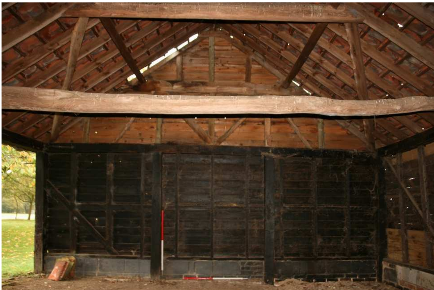
Plate 08 - Northern gable end, looking N
