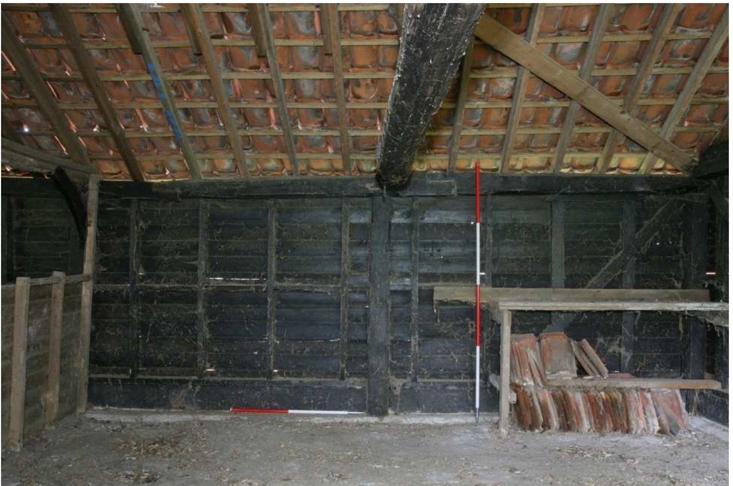
Plate 14 - Eastern interior elevation, Bays 4-5, looking E
