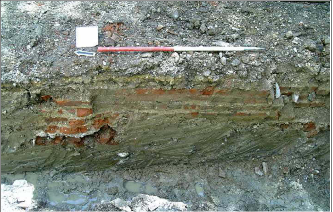
Plate 1: Foundation to demolished eastern extension
