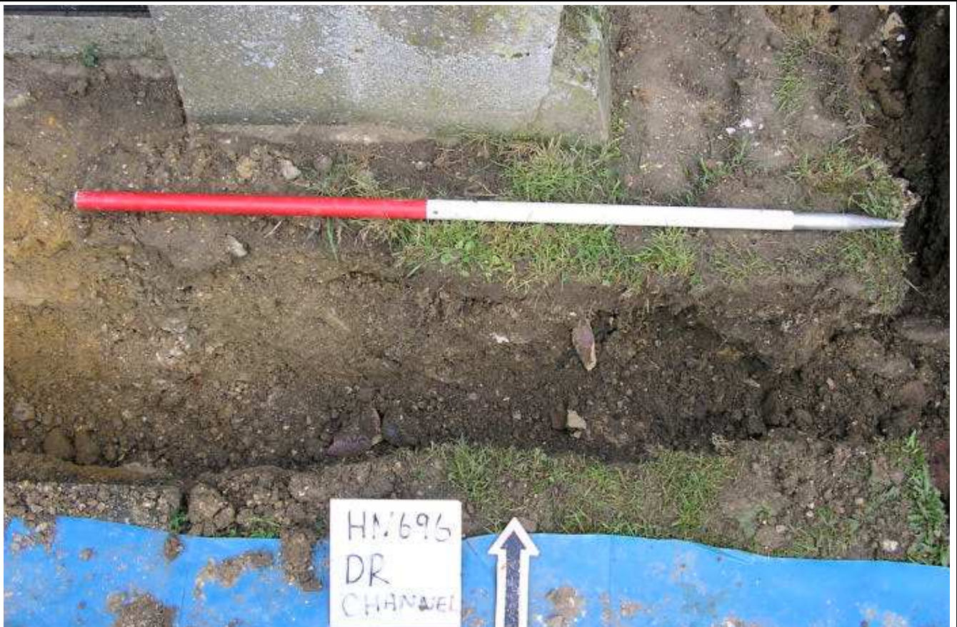
Plate 2: Drainage trench at base of porch, looking north
