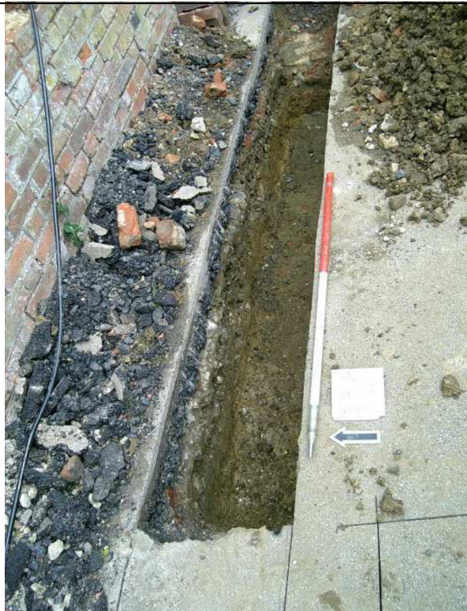
Plate 2: South western service trench looking northeast
