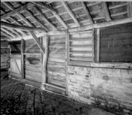
Barn 1, Bays 1 and 2, looking SE
