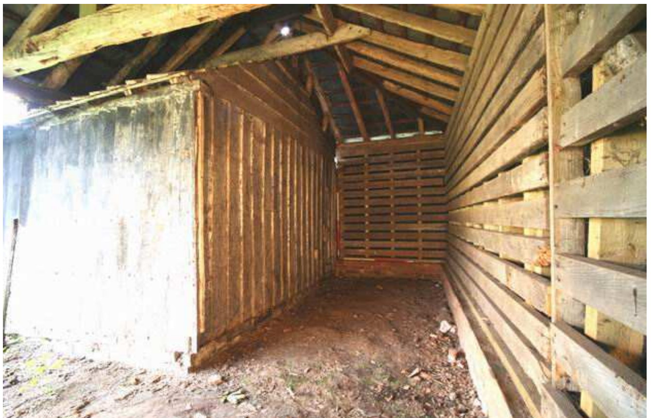
Plate 6: Junction between Barns 1 and 2, looking S
