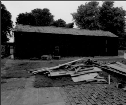
Barn 3, E elevation, looking W
