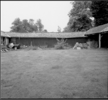
Barn 1, N elevation, looking S
