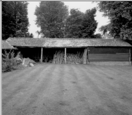
Barn 2, E elevation, looking W
