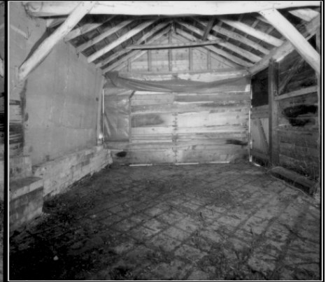
Barn 1, Bays 1 and 2, looking E
