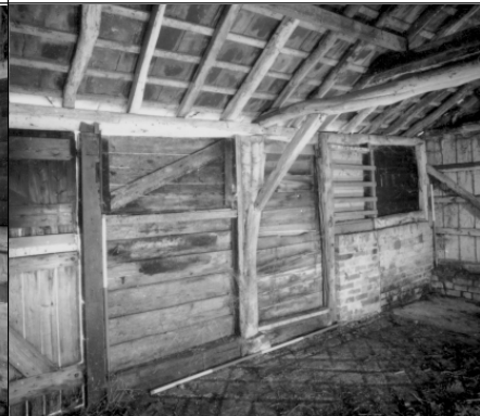
Barn 1, Bays 1 and 2, looking SW
