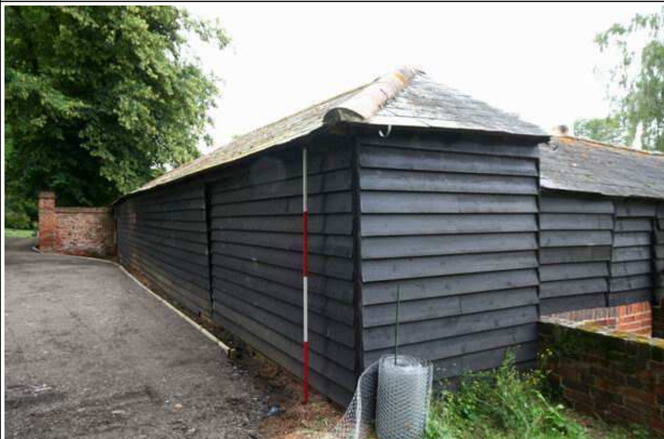
Plate 8: Barn 2, south and west elevations looking NE
