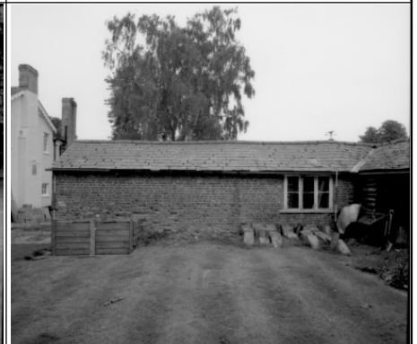
Barn 3, W elevation, looking E
