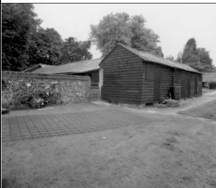
Barn 3, S and E elevations, looking NW
