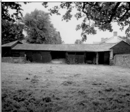
Barn 1, S elevation, looking N
