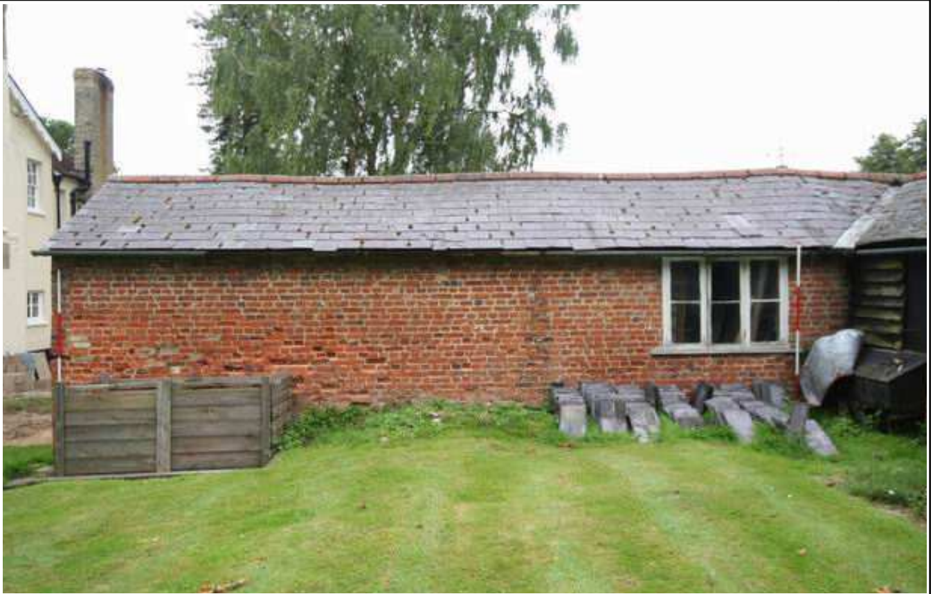
Plate 9: Barn 3, west elevation, looking E
