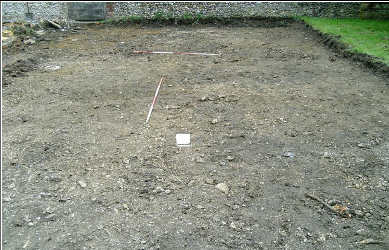
Plate 12: Ground reduction to the south of Barn 1, looking E
