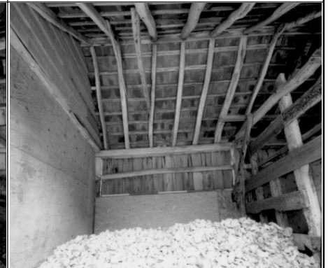
Barn 1, Bay 3, looking N
