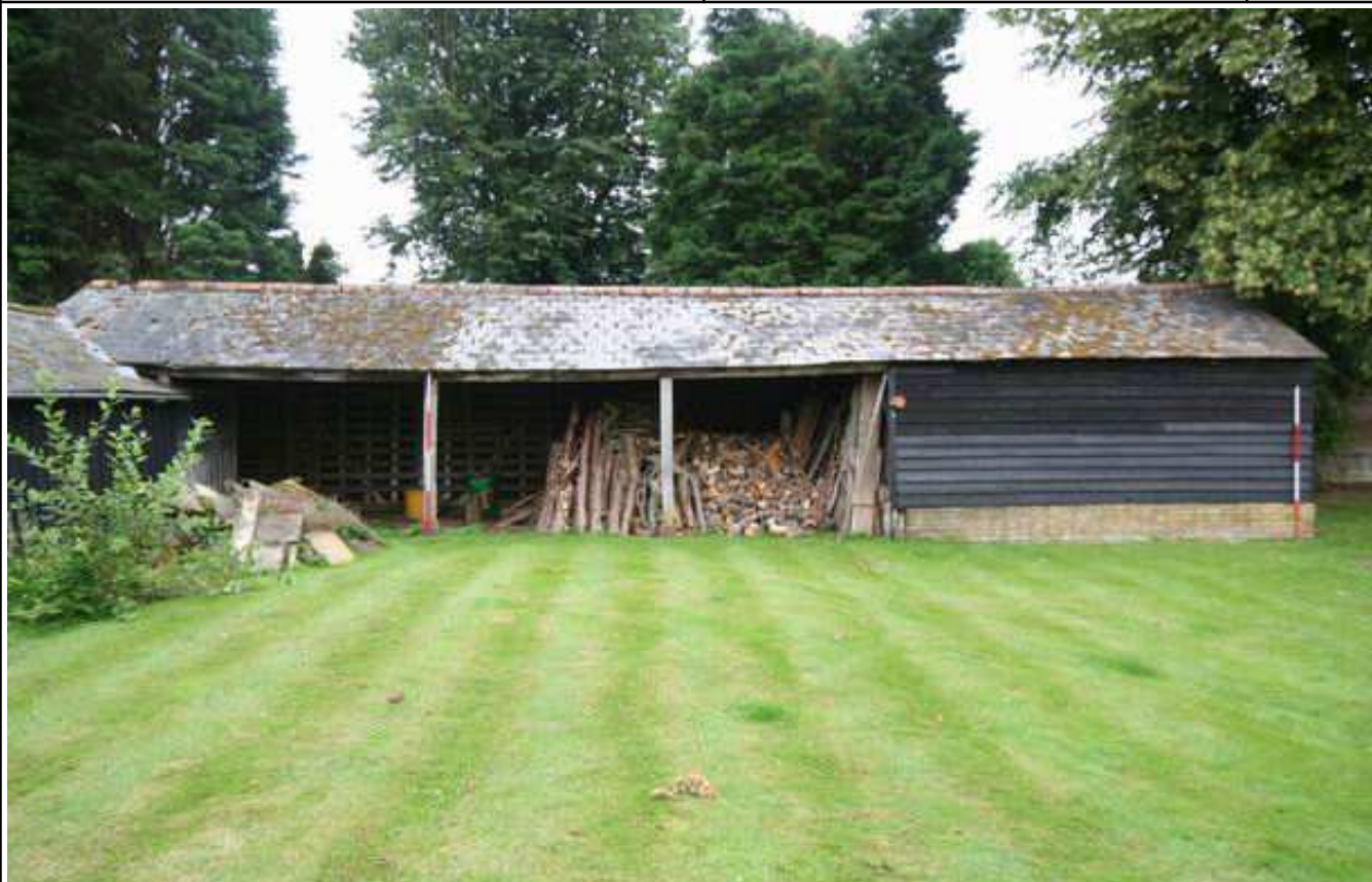
Plate 7: Barn 2, east elevation, looking W
