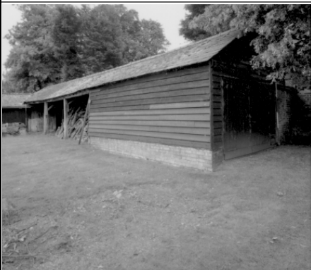
Barn 2, N and E elevations, looking SW
