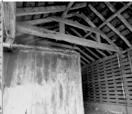
Barn 2 roof truss, looking SW
