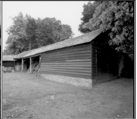
Barn 2, N and E elevations, looking SW
