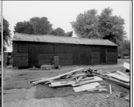
Barn 3, E elevation, looking W
