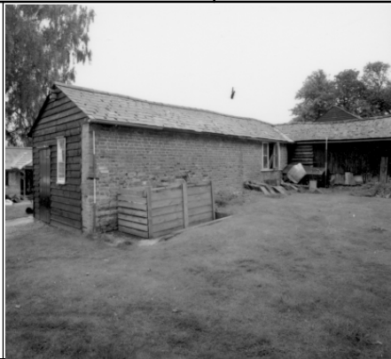
Barn 3, N and W elevations, looking SE
