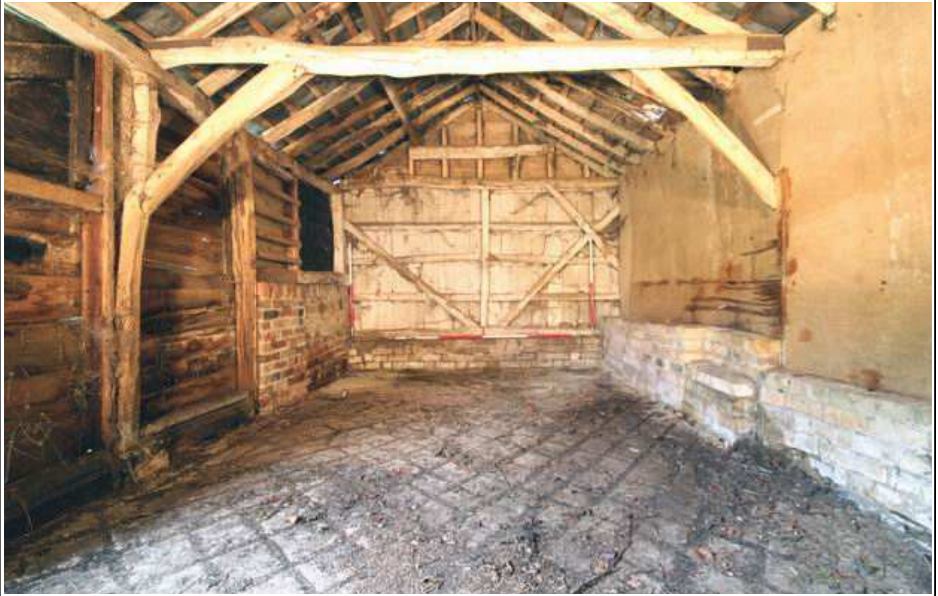
Plate 3: Barn 1, Bays 1 and 2, looking west
