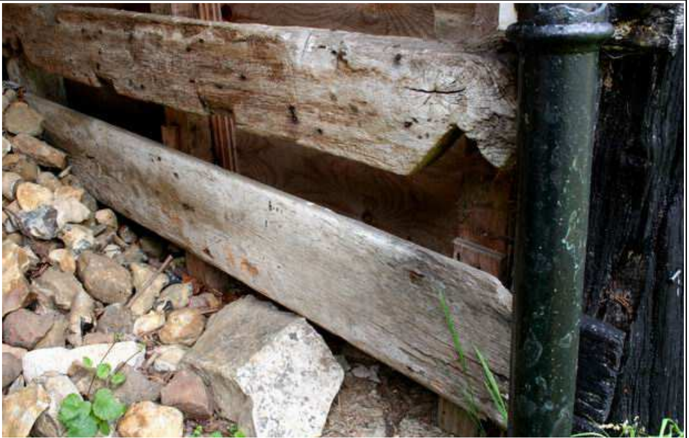
Plate 5: Re-used timbers in Barn 1, detail
