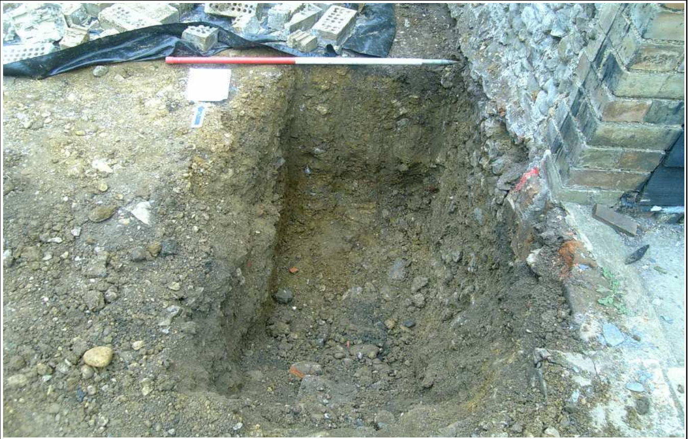
Plate 14: Pad 1, looking north
