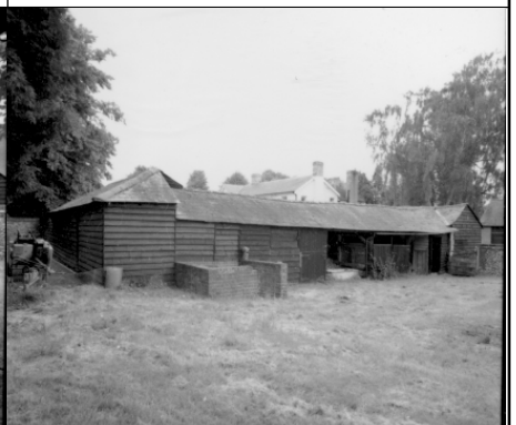
Barns 1 & 2, S & W elevations, looking NE
