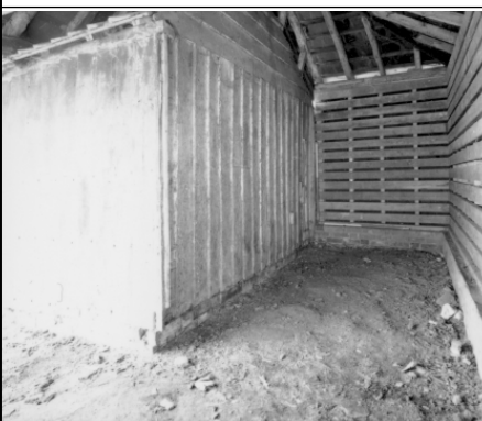
Junction, Barns 1 and 2, looking S
