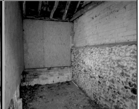
Barn 1, Bay 5 E elevation, looking N
