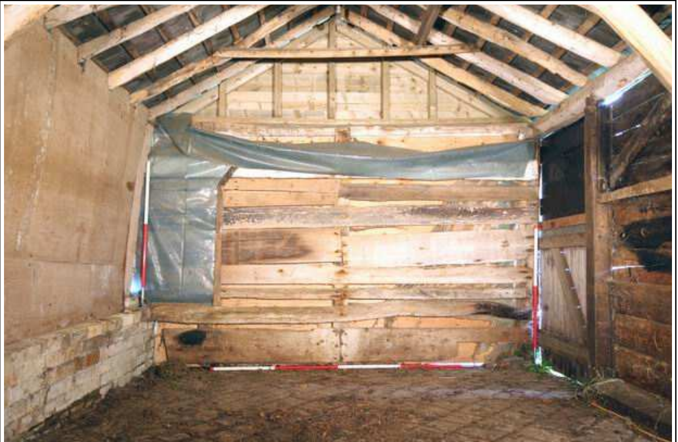
Plate 4: Barn 1, Bays 1 and 2, looking east
