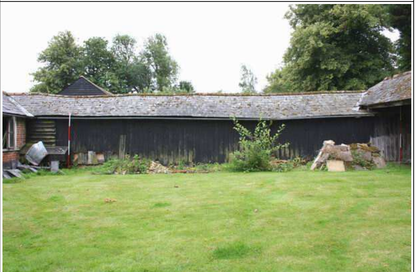
Plate 2: Barn 1, north elevation
