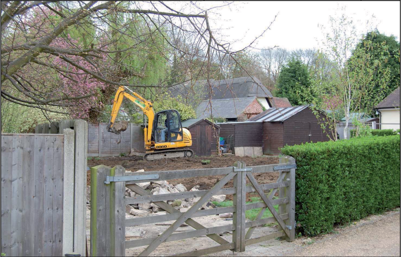
Plate 1: Site, looking south-east
