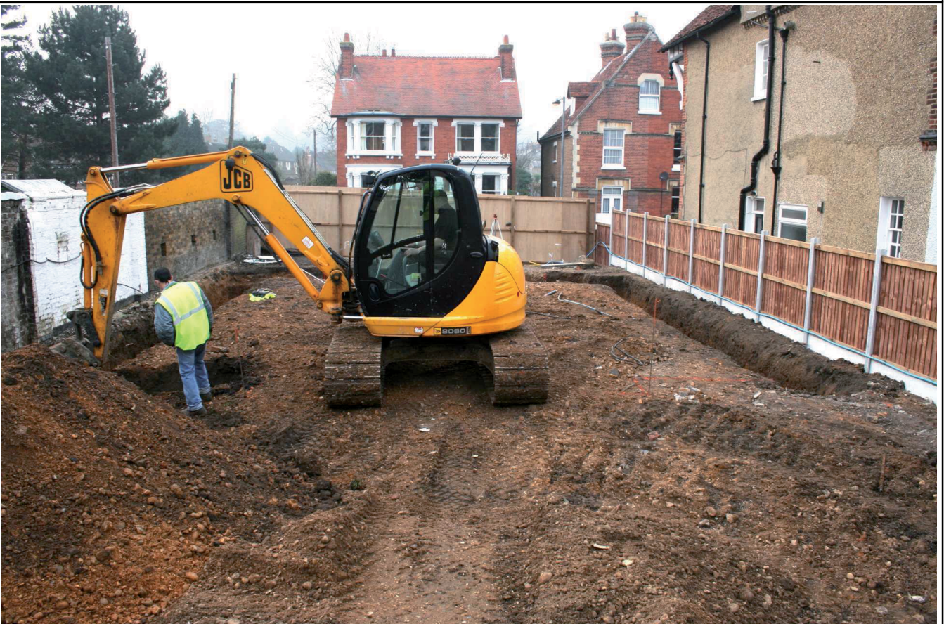
Plate 4: View east to west after demolition of Meadow Cottage
