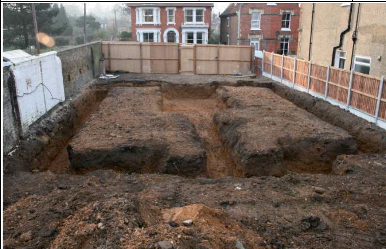
Plate 5: Construction footings
