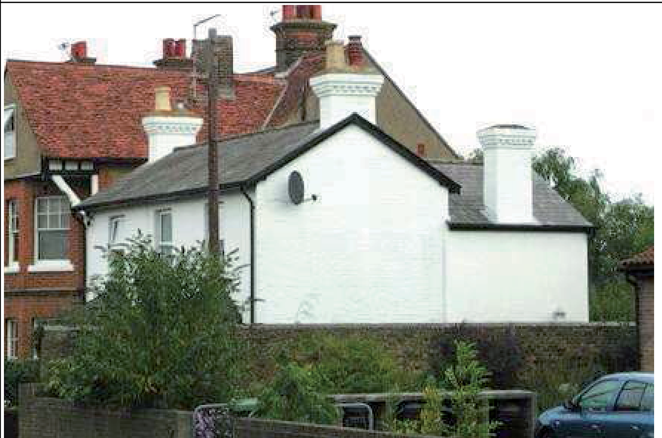
Plate 2: West and south elevation (Photo courtesy of Bayhill Homes)
