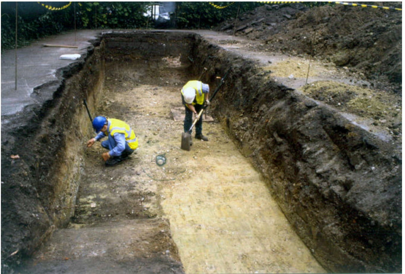
Fig 19: Working shot looking south-east in trench 2
