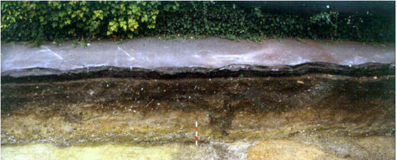
Fig 21: View looking north-east in trench 2 showing, showing the north-east section (figs 10-12). Scale 0.5m
