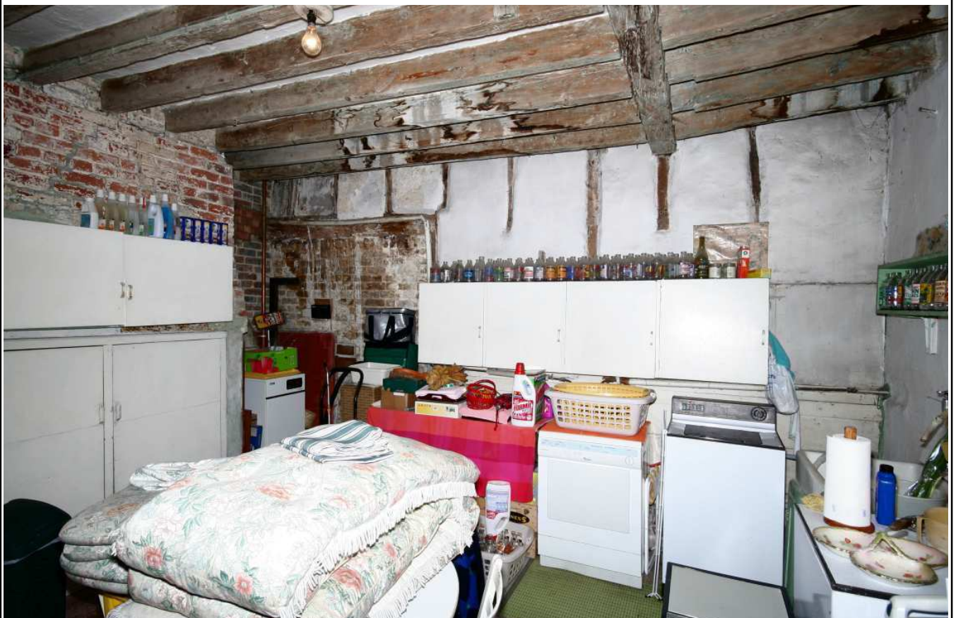
Plate 58: Rear range, Pantry, north elevation
