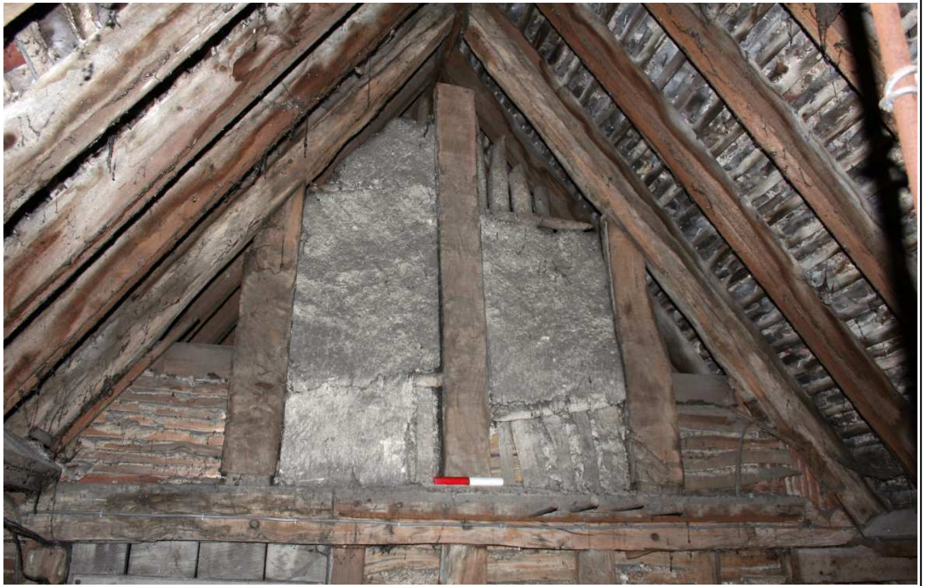
Plate 39: Attic, detail of wattle and daub in partition between Bays 4 & 5
