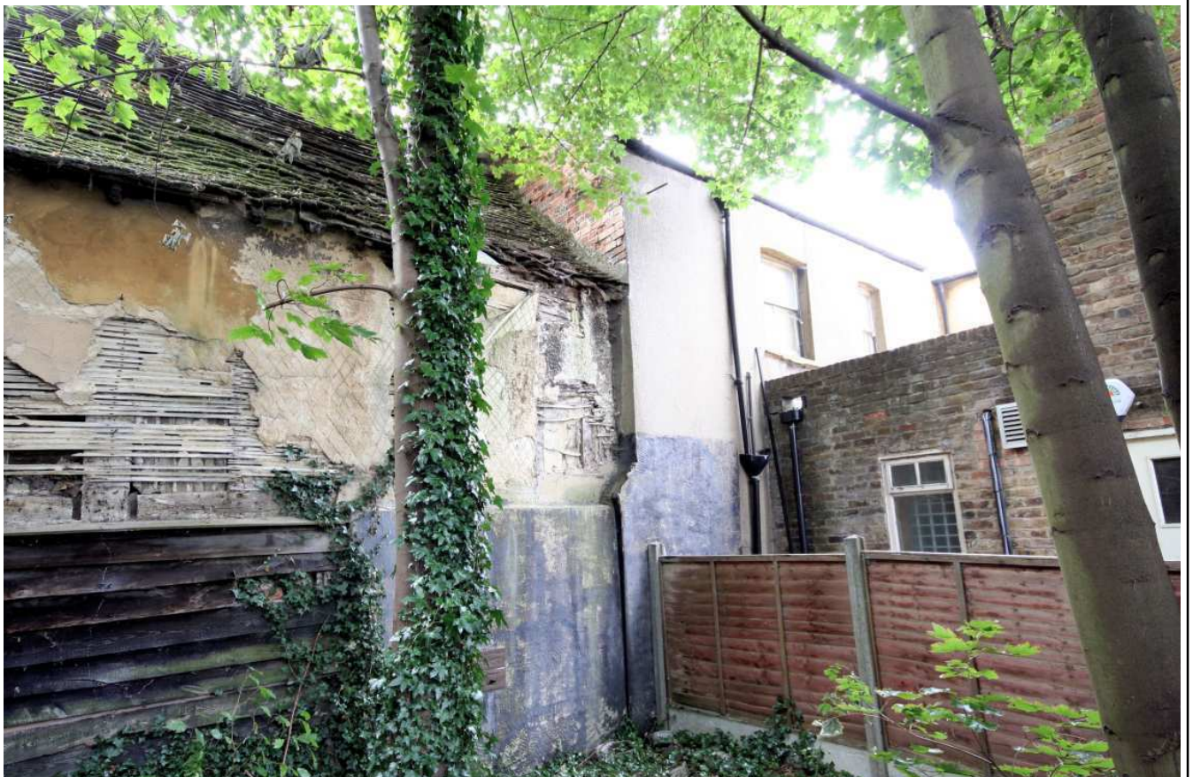
Plate 48: Former kitchen wing, north exterior elevation
