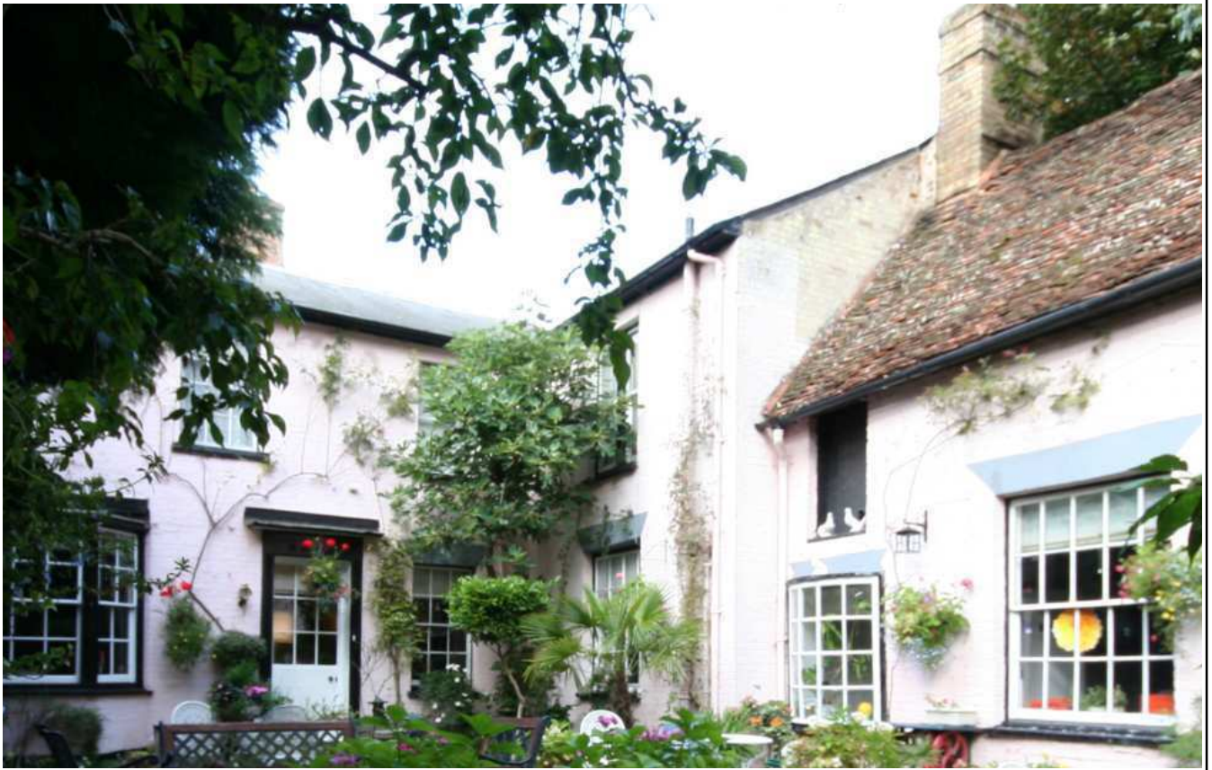
Plate 47: Former kitchen wing, south and east exterior elevations
