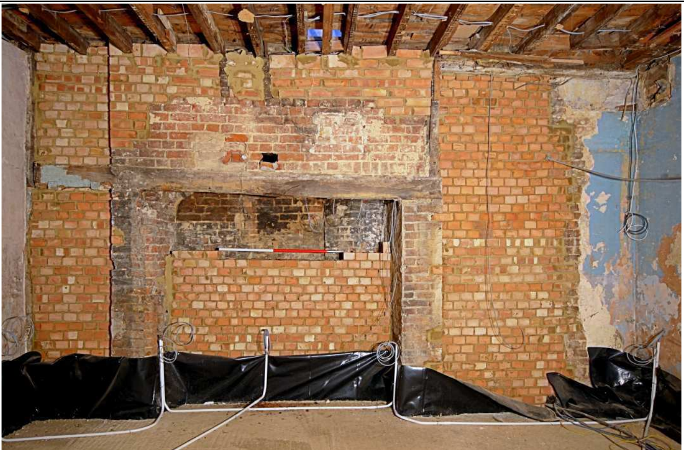
Plate 50: Former kitchen wing, ground floor, east elevation (during works)
