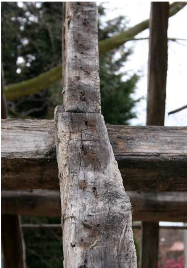
Plate 54: Carpenter's marks on rafters in the roof of the Store
