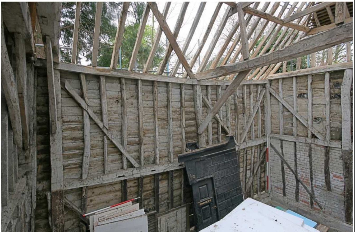
Plate 62: Rear range, the Store, interior north elevation
