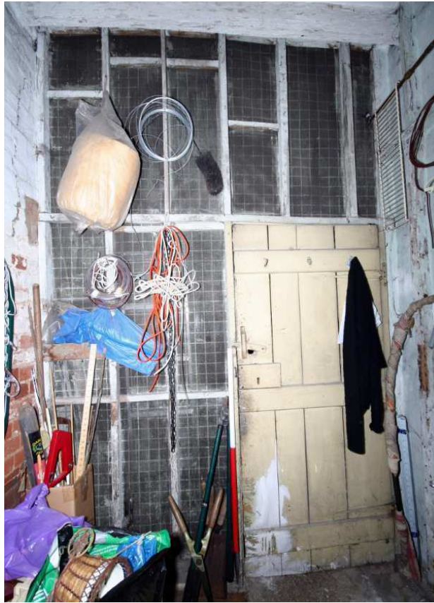
Plate 61: Well Room, south elevation, looking south
