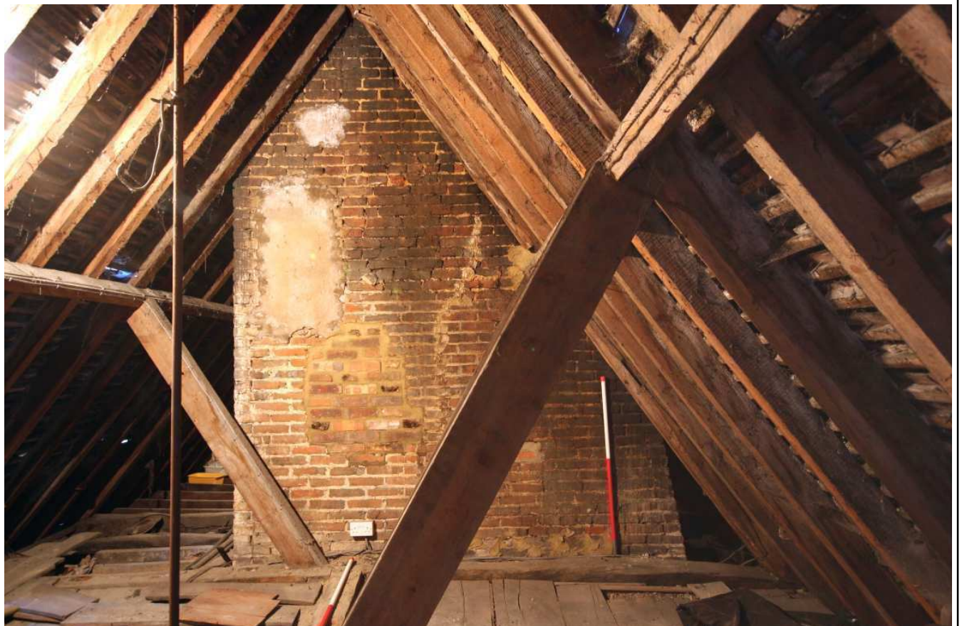
Plate 40: Attic, chimney in Bay 2, looking north
