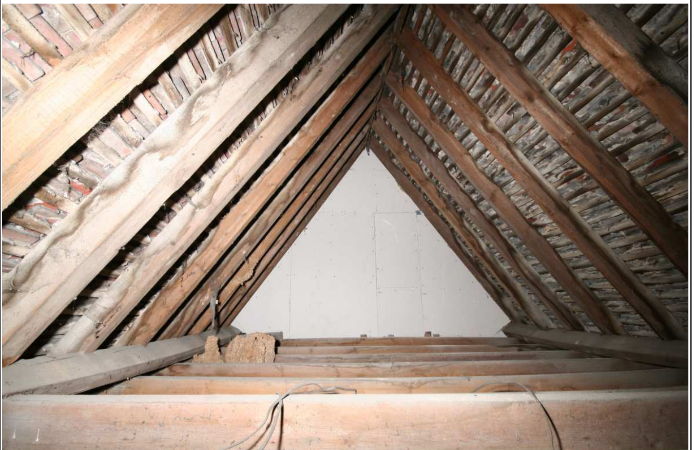
Plate 46: Attic, above the room over the carriageway
