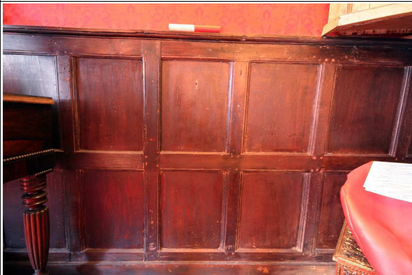
Plate 14: Room 1, detail of Jacobean panelling on the north elevation
