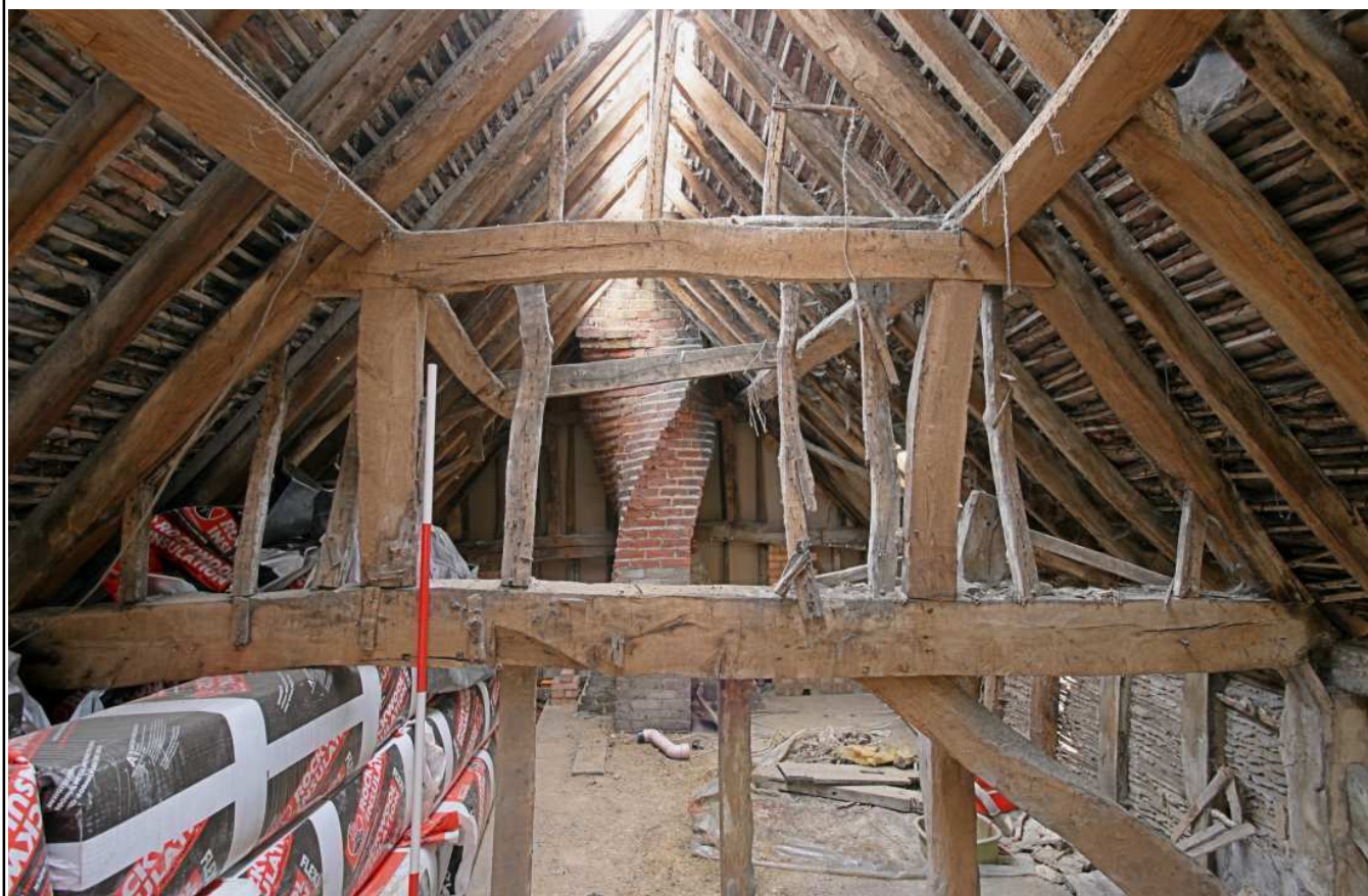
Plate 68: Rear range, roof structure, looking west
