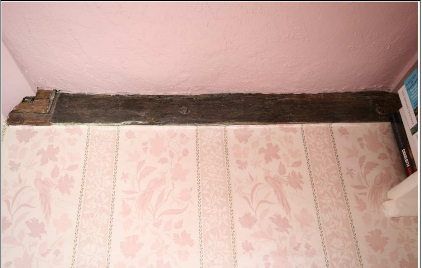
Plate 27: Room 5, exposed wall plate in east elevation
