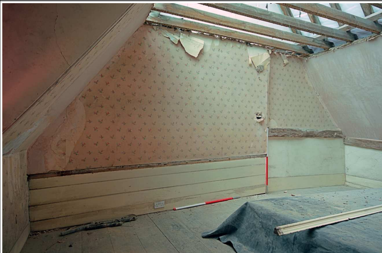
Plate 36: Room above the carriageway, south elevation
