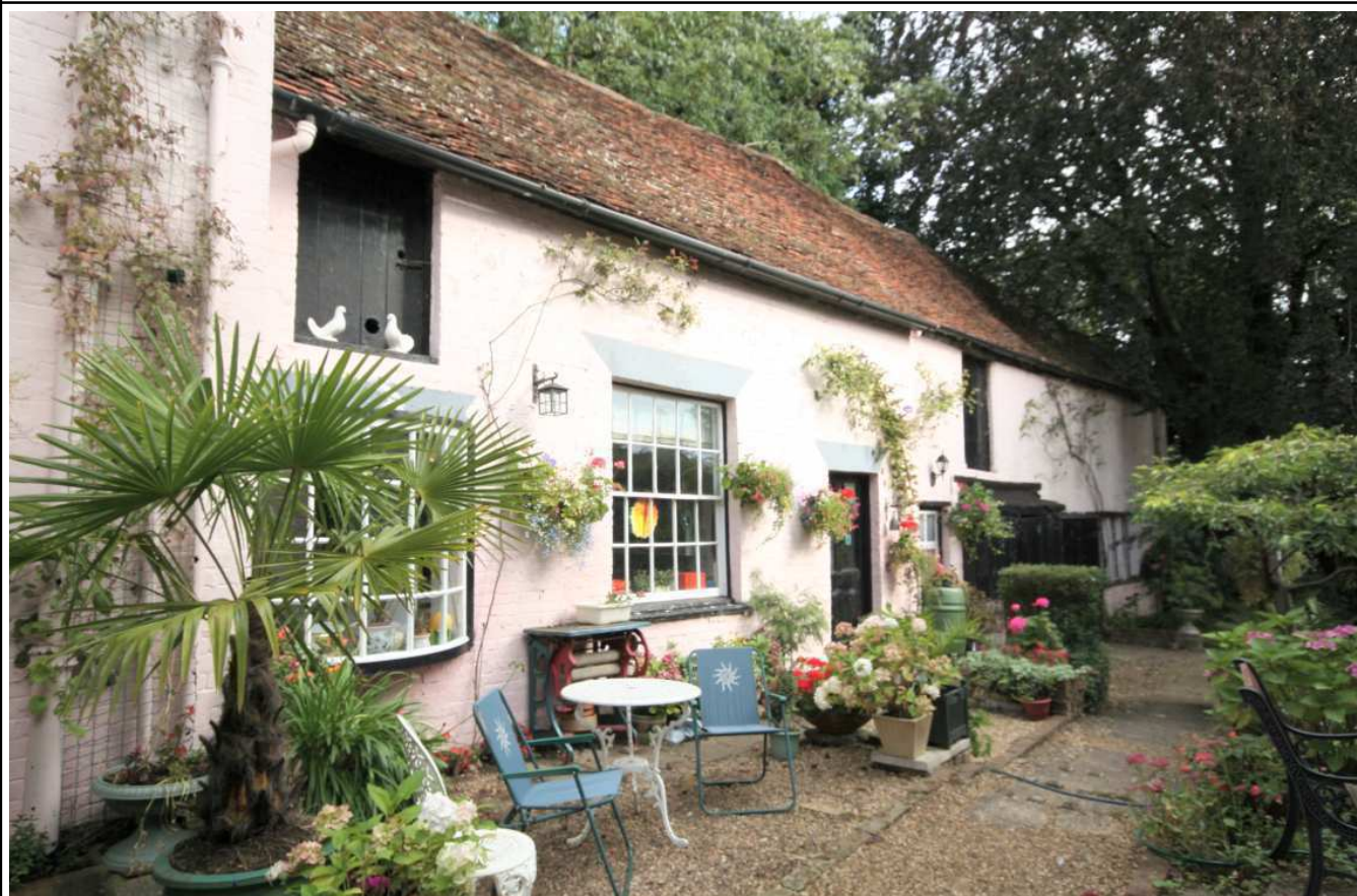
Plate 52: Rear range, south exterior elevation, west end
