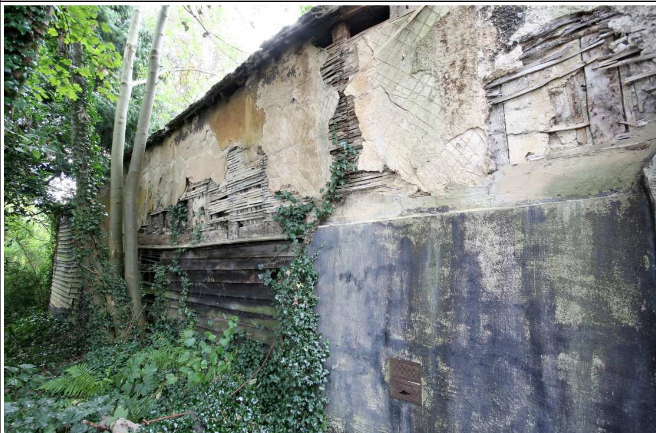
Plate 56: Rear range, north exterior elevation, west end
