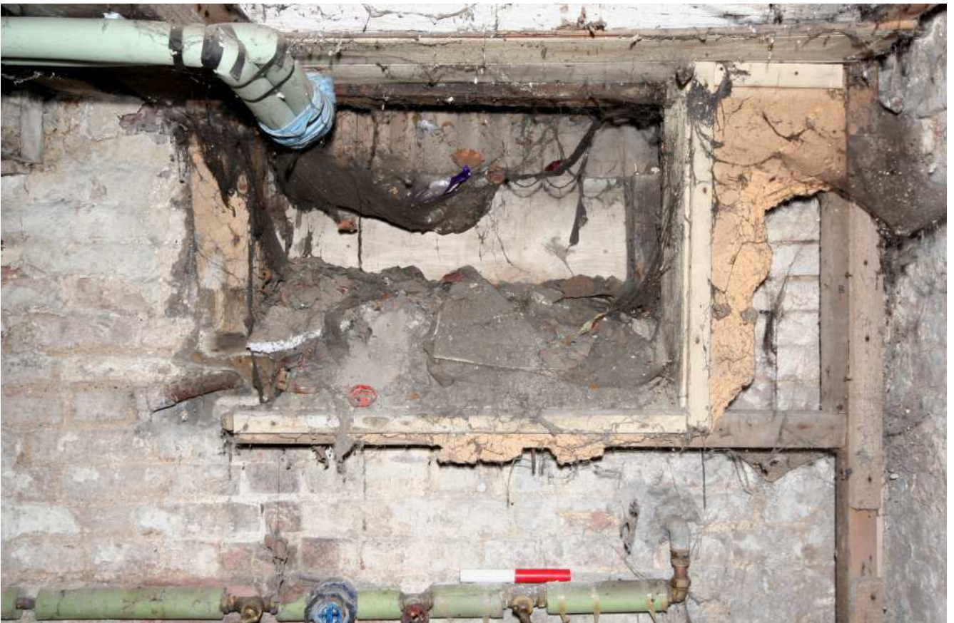
Plate 6: Cellar 2 - coal chute in south elevation
