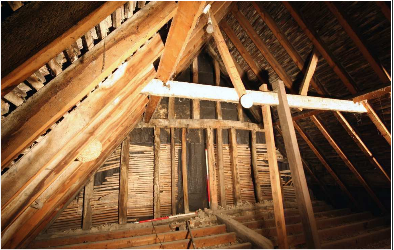
Plate 45: Attic, north gable, looking north
