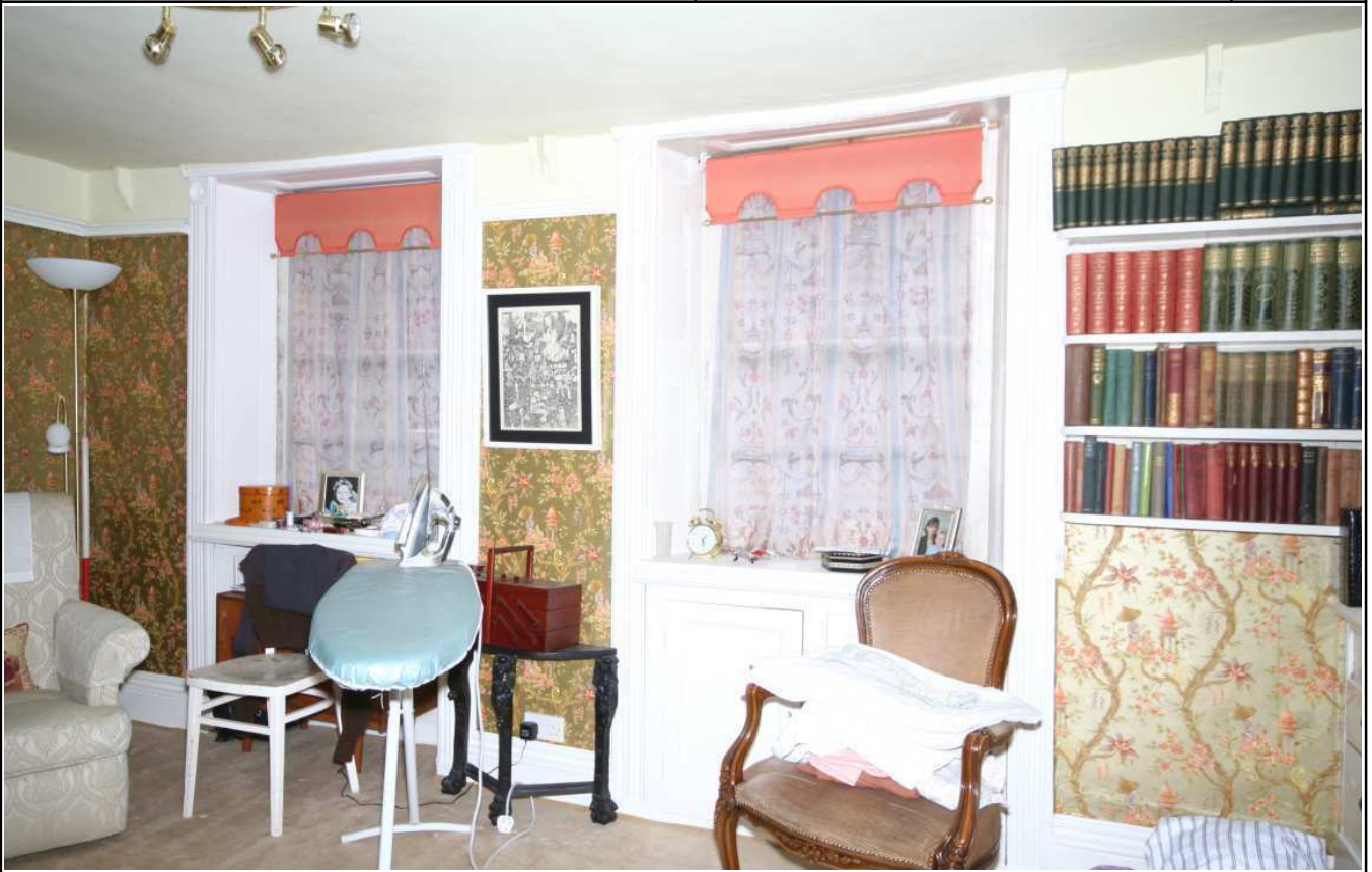
Plate 17: Room 2, west elevation
