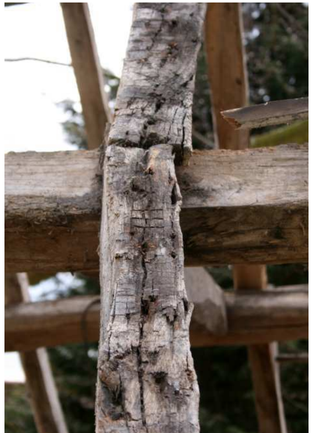
Plate 54: Carpenter's marks on rafters in the roof of the Store
