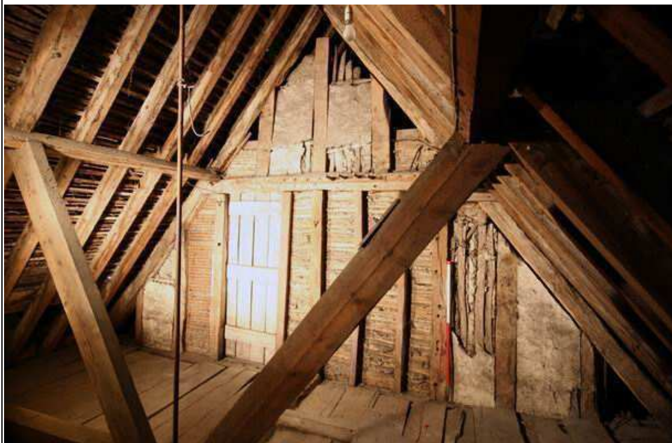
Plate 38: Attic, partition between Bays 4 and 5, looking south
