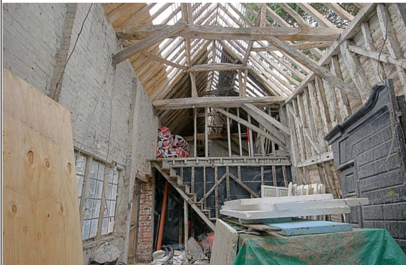
Plate 64: Rear range, the Store, interior west elevation
