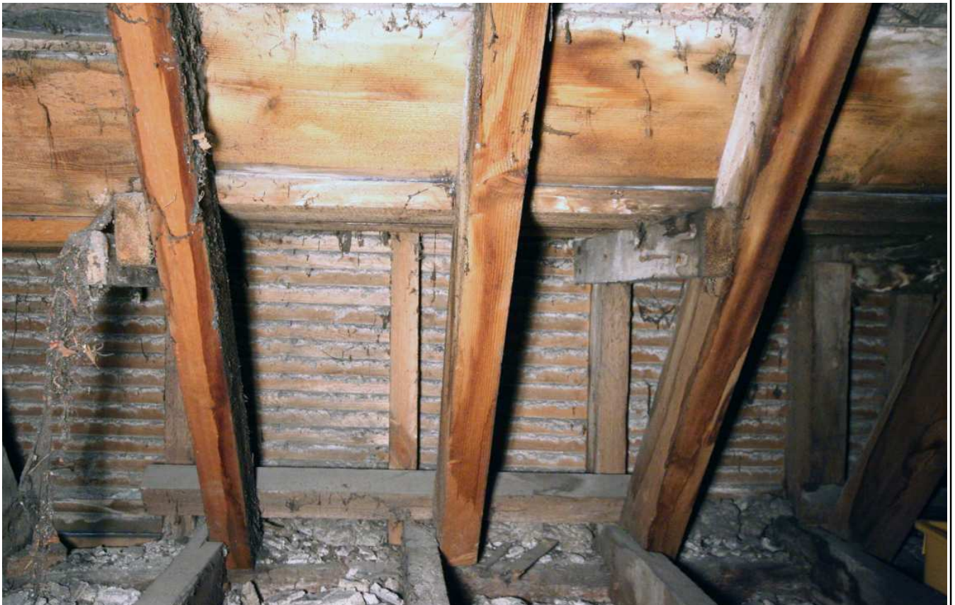
Plate 43: Attic, timber framed parapet at the base of the rafters to west elevation
