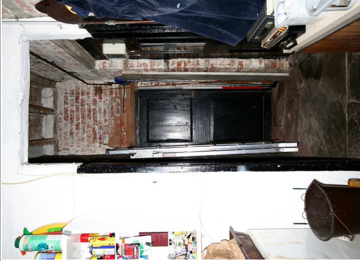
Plate 59: Rear range, hallway outside the Well Room, looking east
