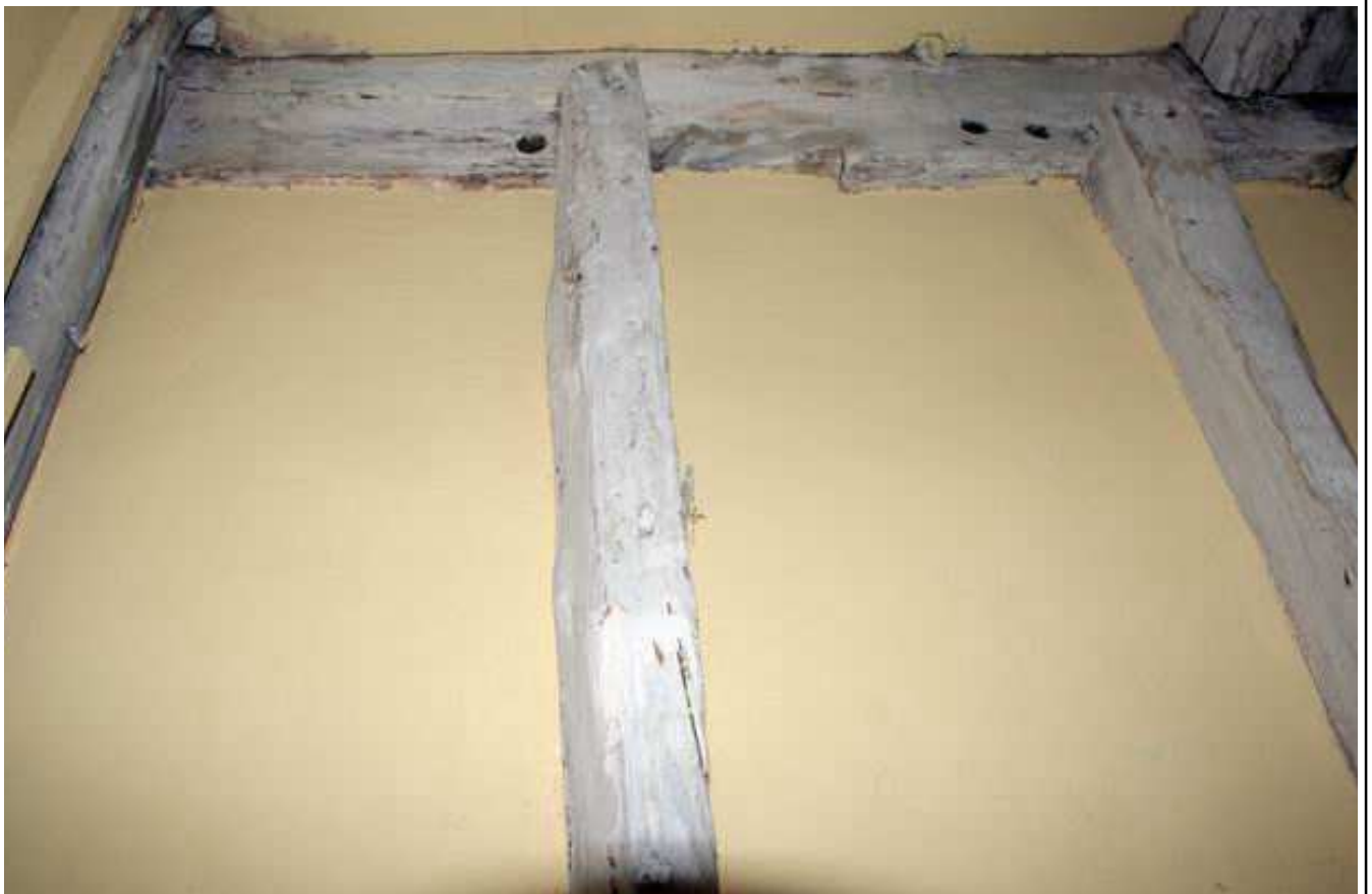
Plate 12: Hall cupboard, timber framing in south elevation
